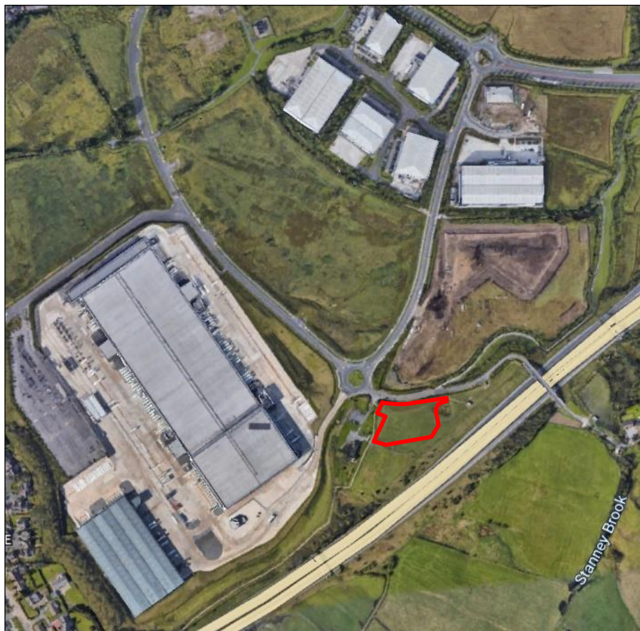
Figure 1– Aerial Plan of the Application Site in Wider Landscape – Site denoted by red line.
