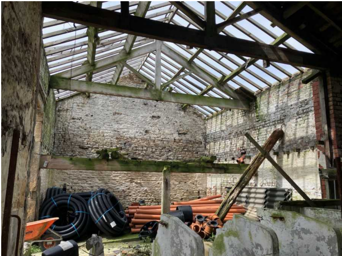
Photo 13: Roof Structure (Bay 1 & Bay 2)
