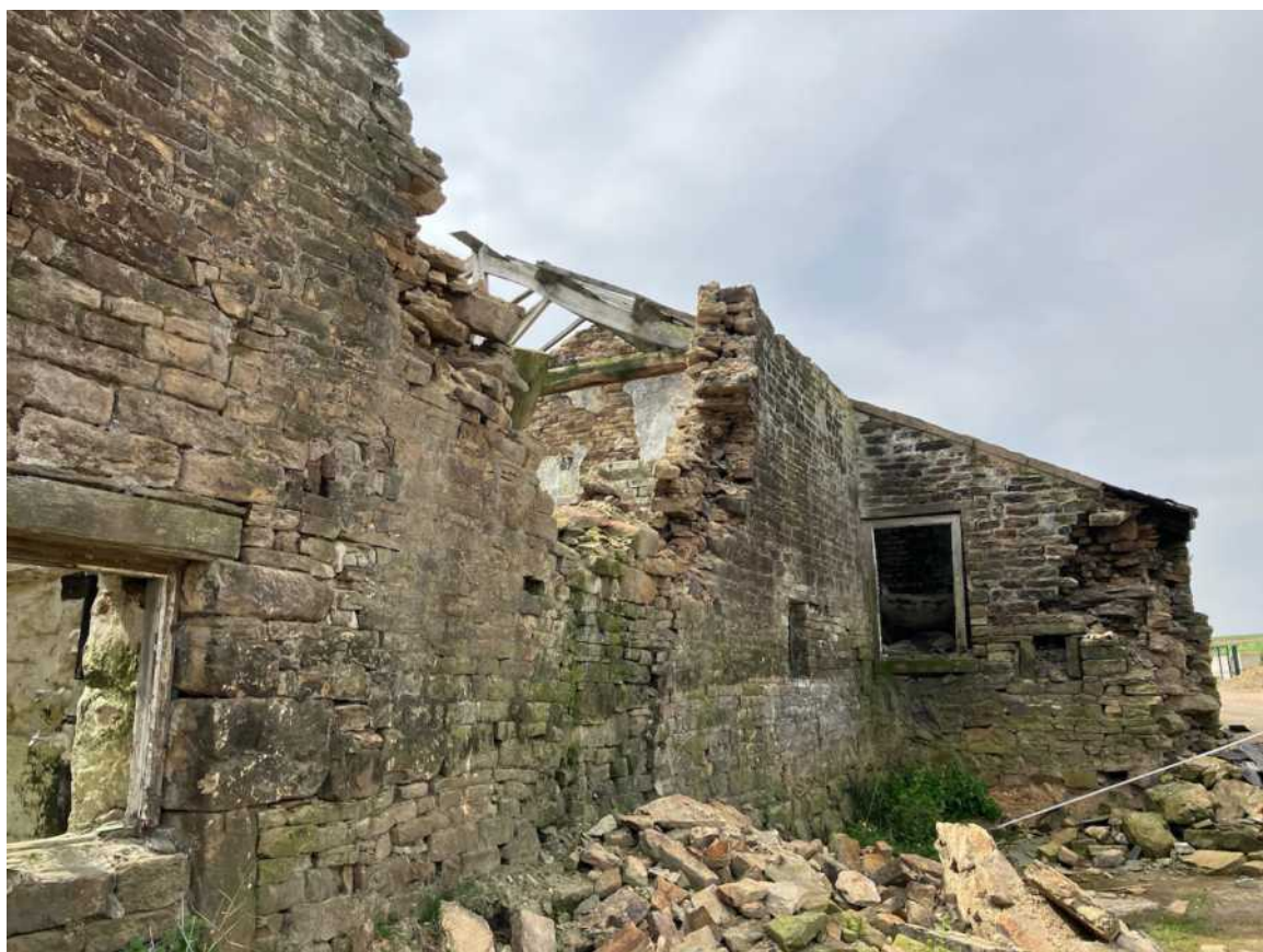
Photo 8: Collapsed Masonry
