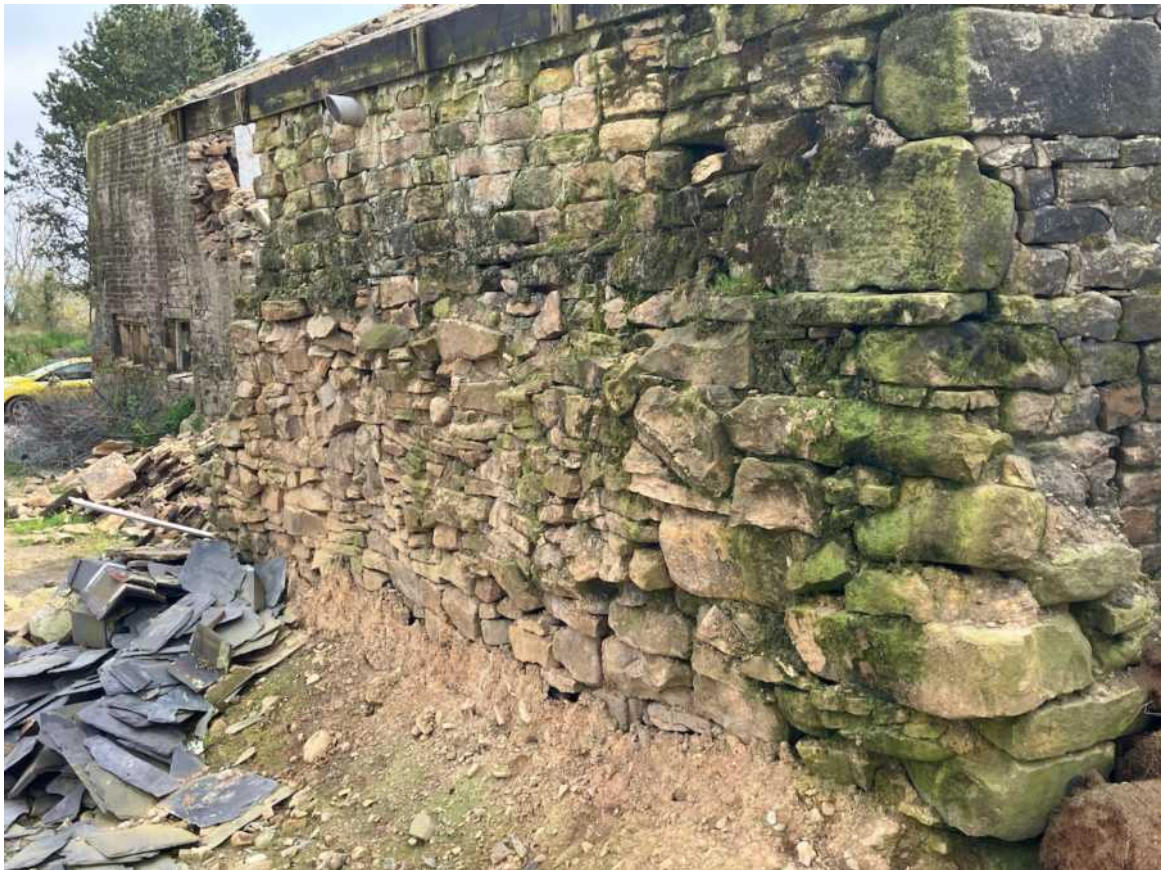
Photo 6: Lean-To Extension – Foundations Exposed
