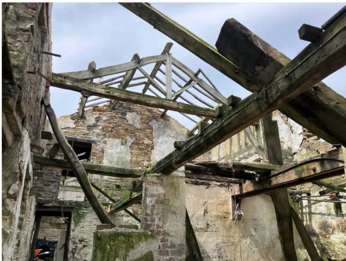
Photo 15: Roof Structure (Bay 4)
