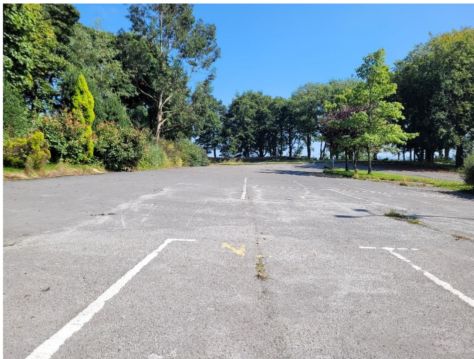
Photo 4: Showing trees within car park area.
