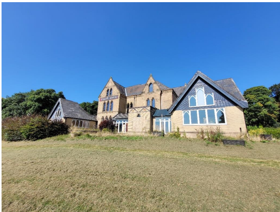
Photo 1: Showing exterior of the restaurant building.
