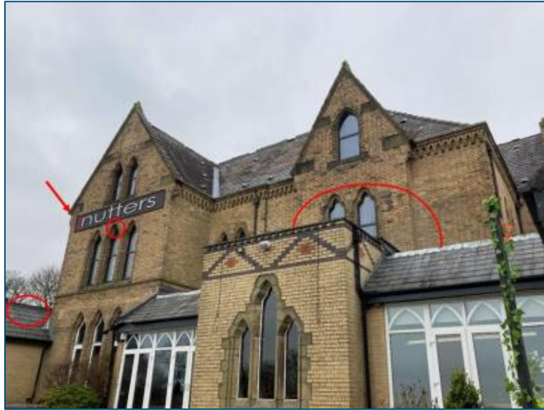
Photo 5: showing some of the emergence (2023) locations on the southern elevation.
