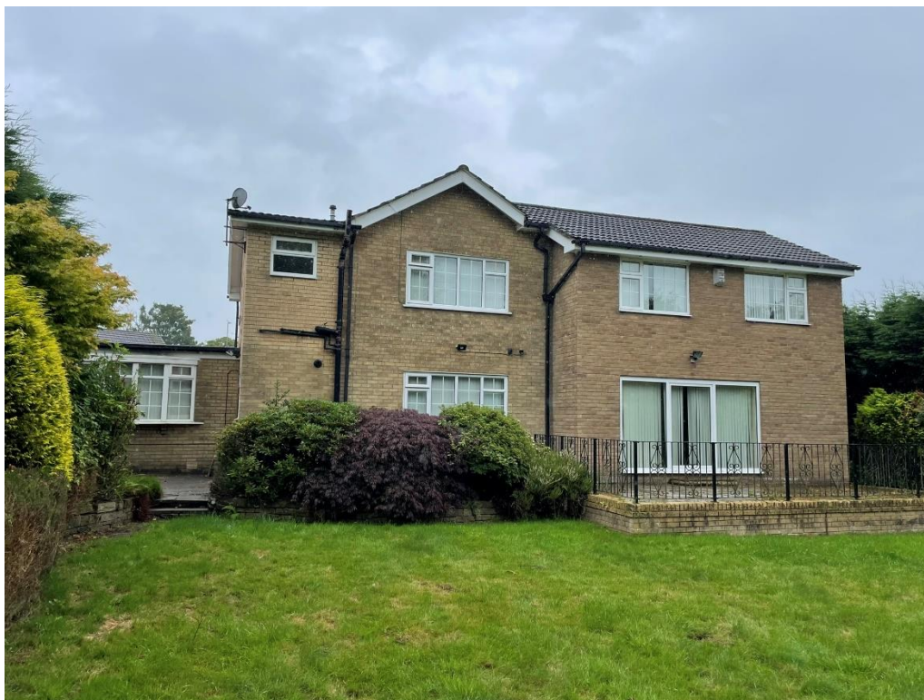
The existing rear elevation of the property
