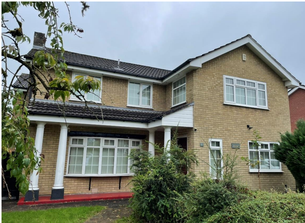
The existing front elevation of the property
