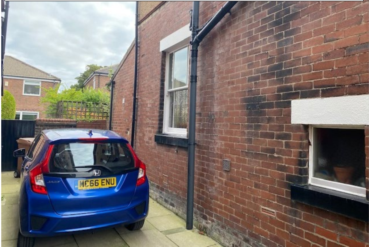
Side elevation view of 4 Hargreaves Street – taken from driveway of No.6 – single storey extension visible
