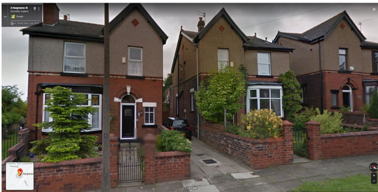
Google Street View Image dated June 2012 showing frontage of property – side of wall and roof of single storey rear extension clearly visible in gap between No.4 and No.6 Hargreaves Street
