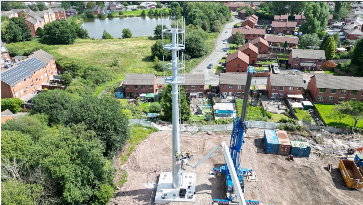
Figure 4 – Aerial imagery of a 30m-high tower deployed at Century Mill, George Street, Farnworth, BL4 9QW and approved by Bolton Council in 2022 (Source: Applicants drone imagery)
