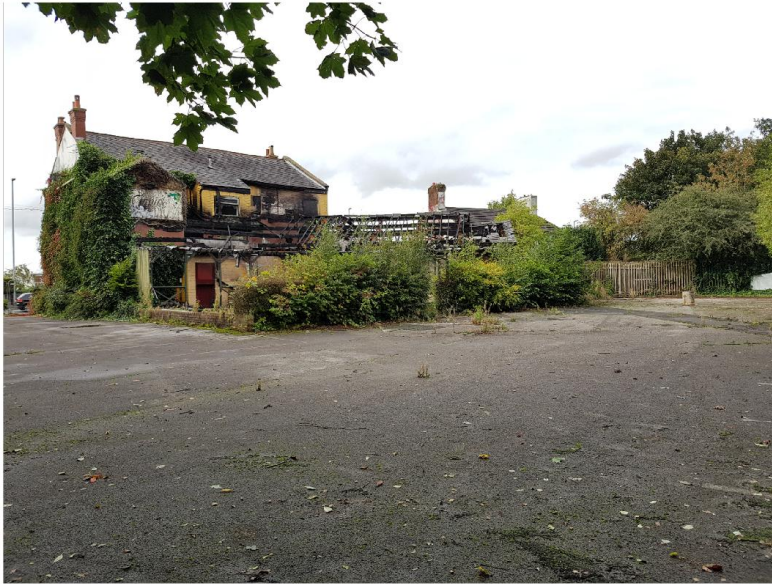
view of site looking northwest
