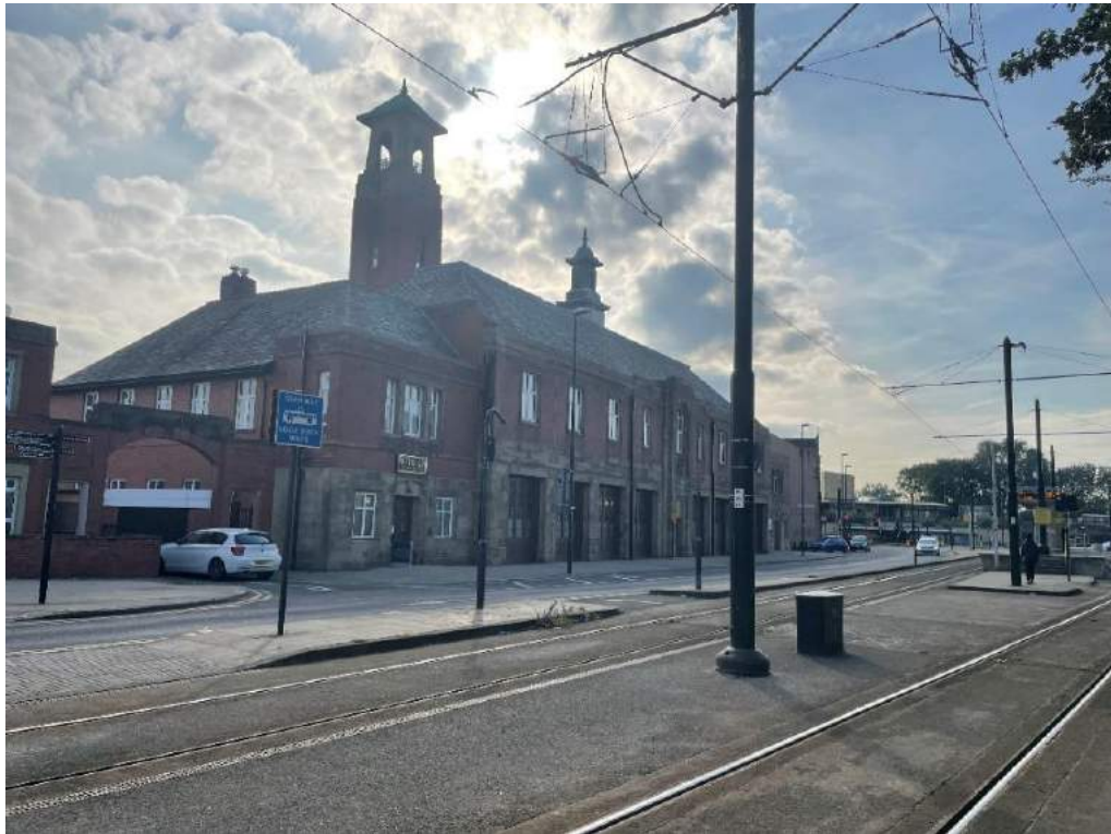
Figure 4-8 - fire station from road, facing south-east.
