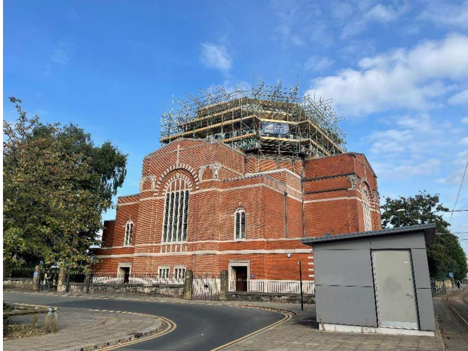
Figure 4-5 - Grade II* listed St John the Baptist RC Church, south elevation facing north.
