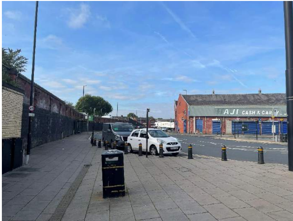
Figure 4-14 - Rochdale Station viaduct, from the front of Rochdale Railway Station, facing west. .
