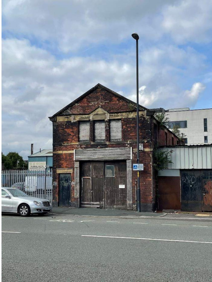
Figure 4-15 - Small early 20th century industrial building, from Station Road, facing north.
