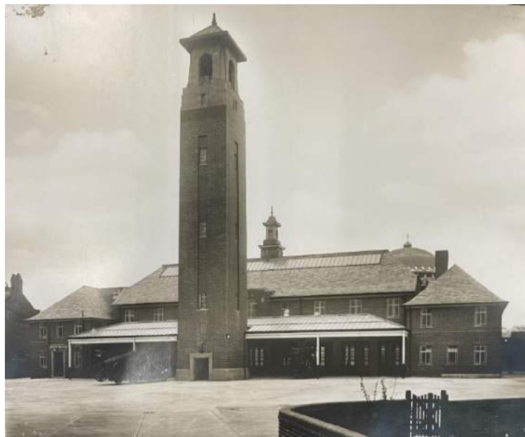
Figure 4-7 - Fire station (rear), drill yard and hose tower (the dome of St John's can be seen in the background) © Rochdale Local Studies and Archive 2022
