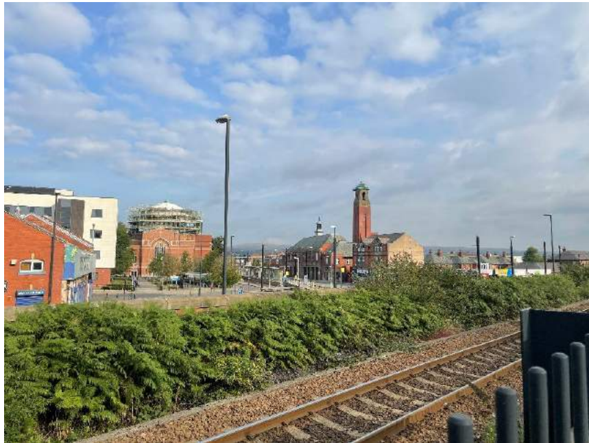
Figure 5-1 - View of the Church of St John the Baptist RC Church from the platforms at Rochdale Railway Station.
