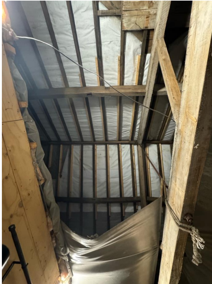
B1 Loft 2: loft void of barn section of B1
