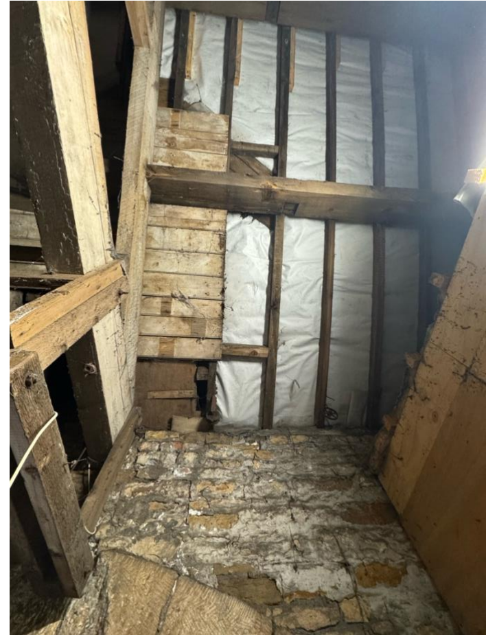
B1 Loft 2: loft void of barn section of B1
