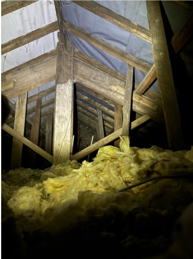
B1 Loft 1: loft void of currently occupied residential area
