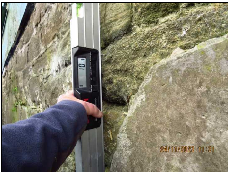
021 Satisfactory vertical alignment, \pm 5\text{mm} per metre
