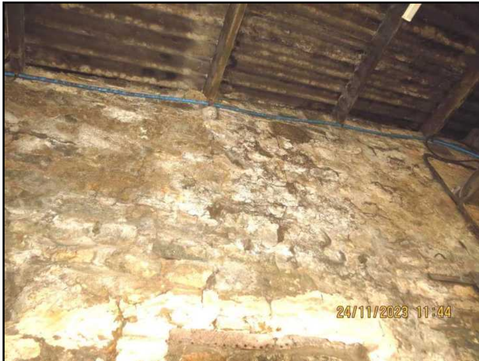
052 Upper wall, East
