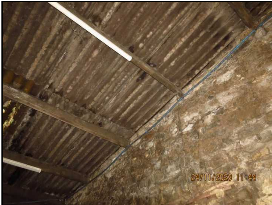
050 Eastern gable, roof support
