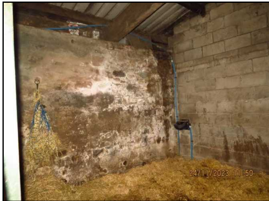
Photograph 072 Rear wall and party wall North East corner
