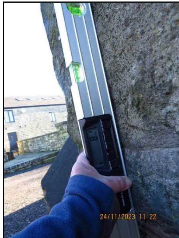
010 Good vertical alignment 8mm per metre
