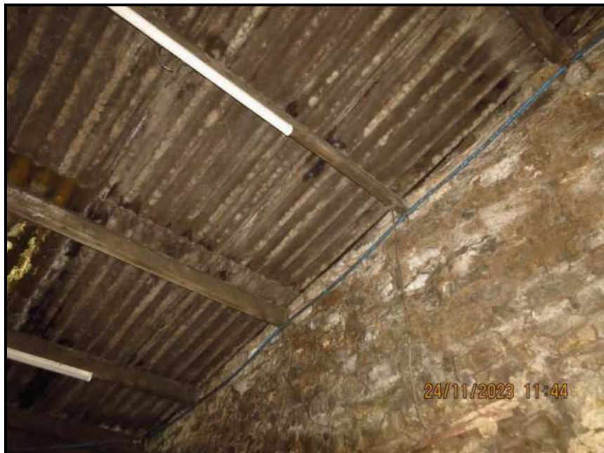
Photograph 050 Eastern gable roof support
