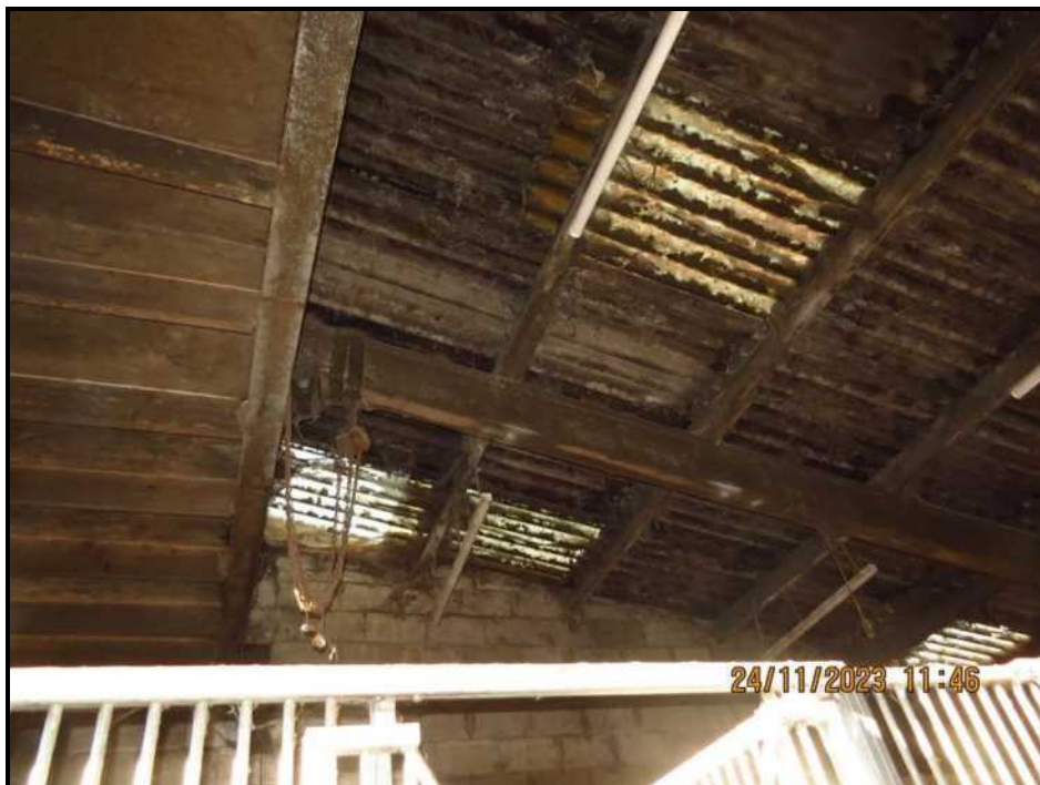
057 Internal cross wall to Stable No. 2
