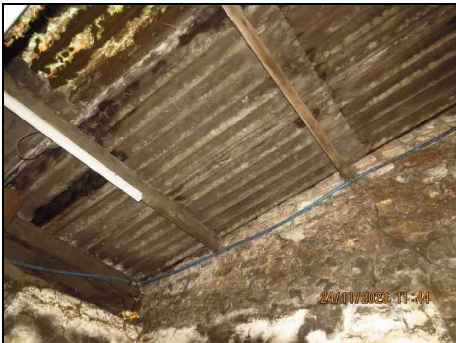
049 Eastern gable, roof support
