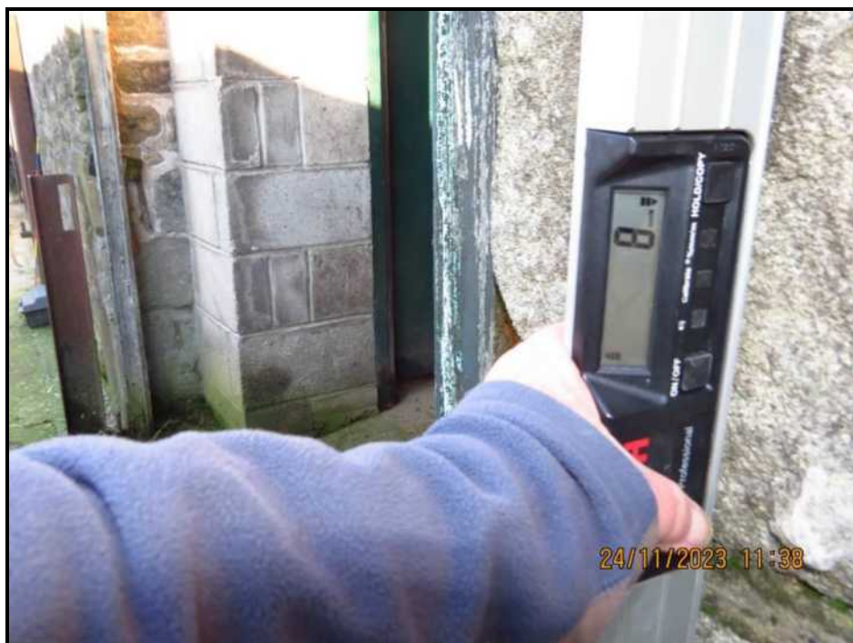
031 Good vertical alignment
