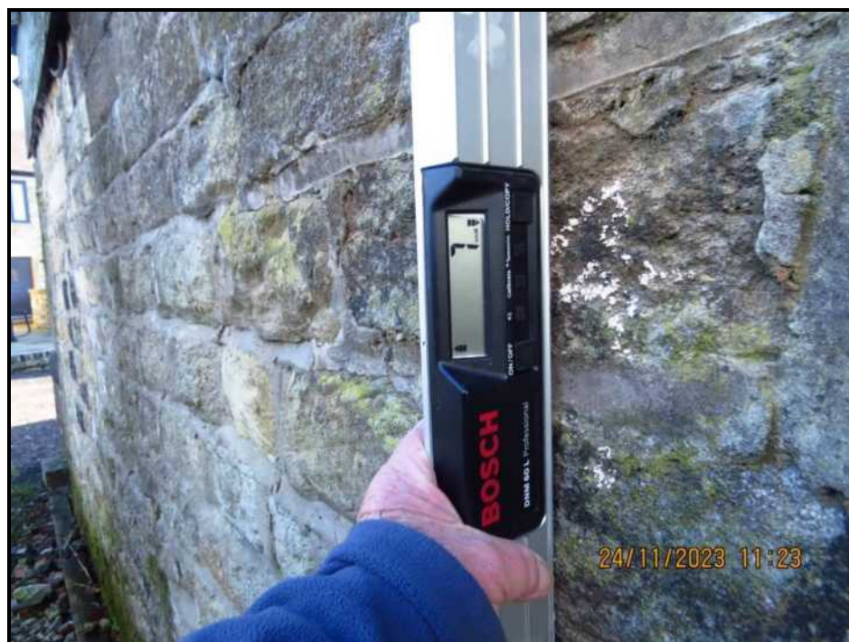
011 Chainage 4 metres, 7mm per metre
