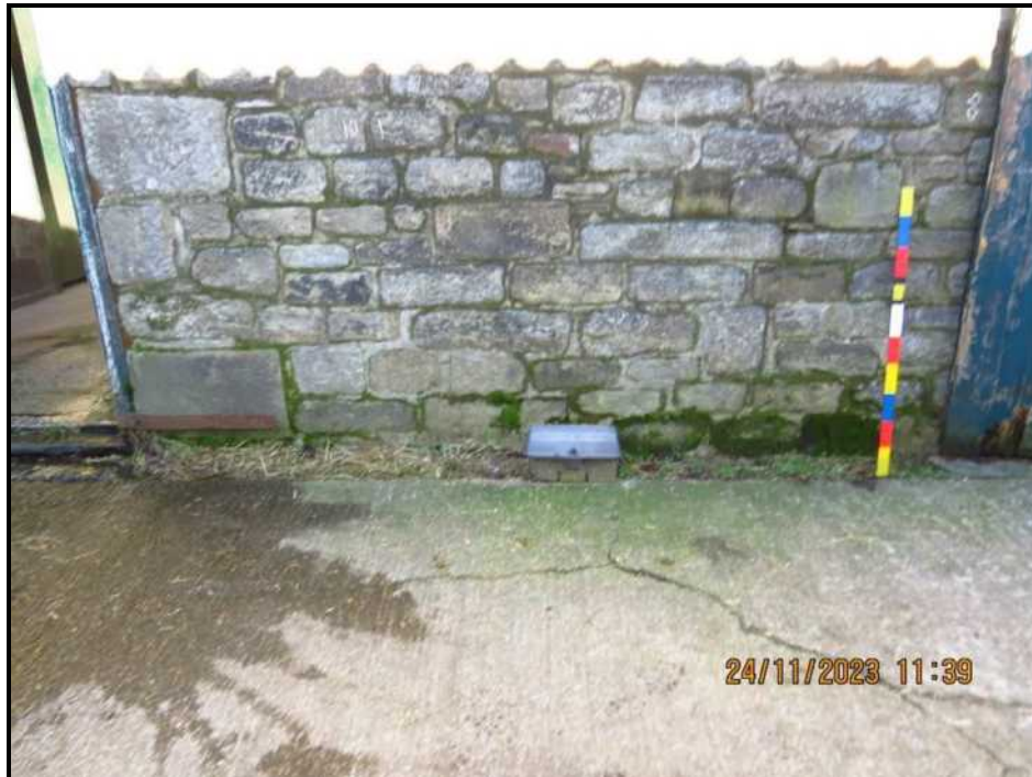
032 Plinth wall, chainage 10 – 7 metres
