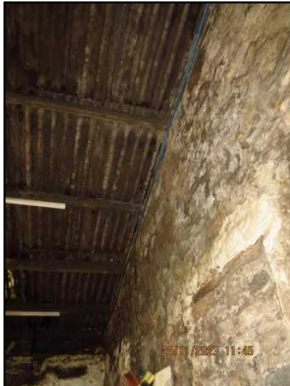
055 Gable elevation looking to rear
