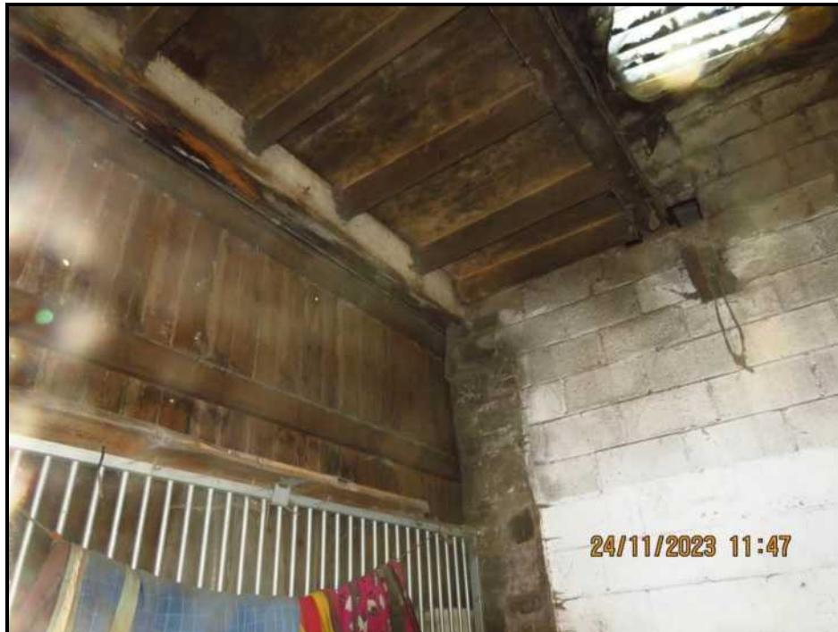
060 Front elevation, upper roof and cross wall
