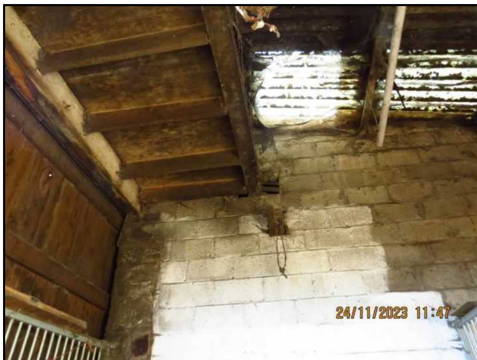
061 Internal party wall with Stable No. 2
