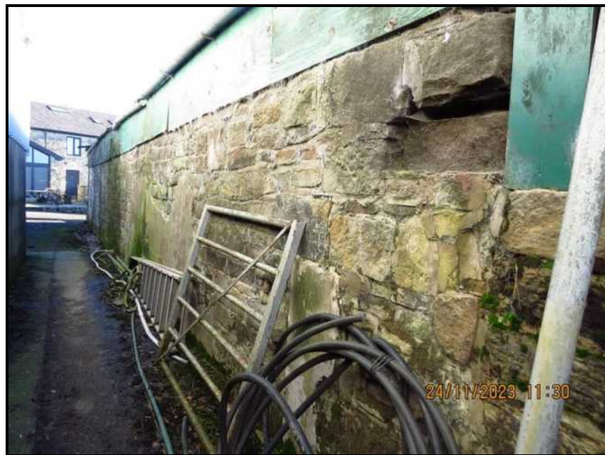
Photograph 020 Rear elevation looking South East
