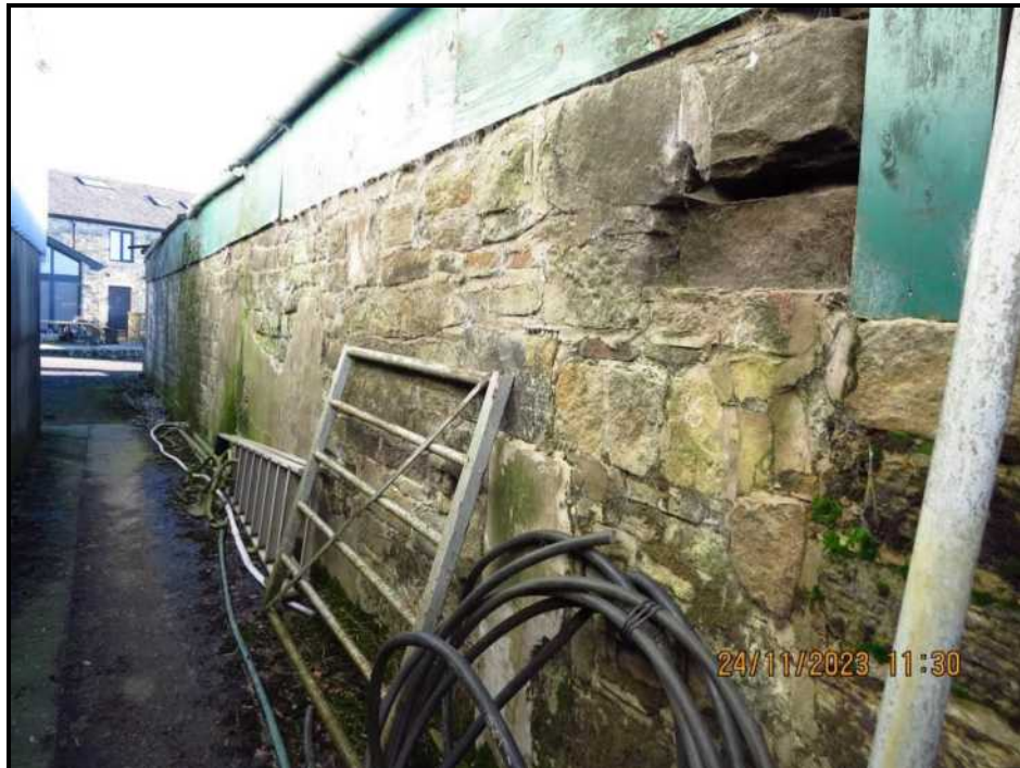
020 Rear elevation looking South East
