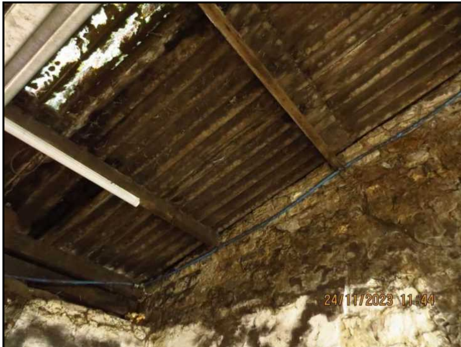
045 Purlin seating, Eastern gable
