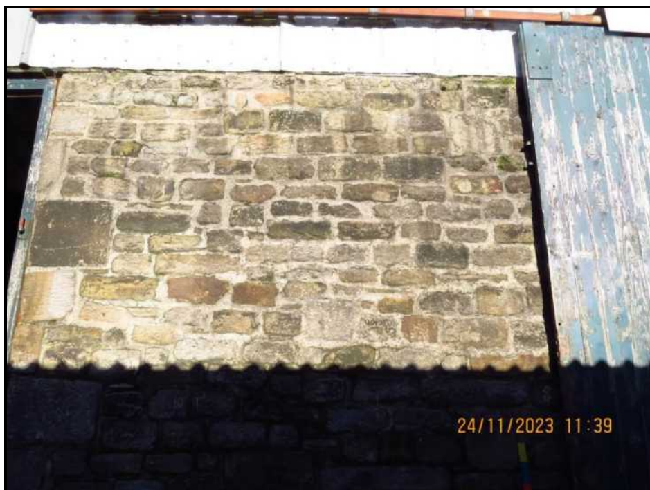
033 Upper wall, chainage 10 – 7 metres
