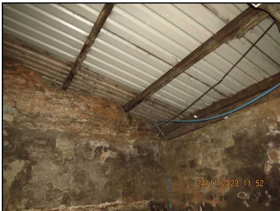
076 Western cross wall/rear wall
