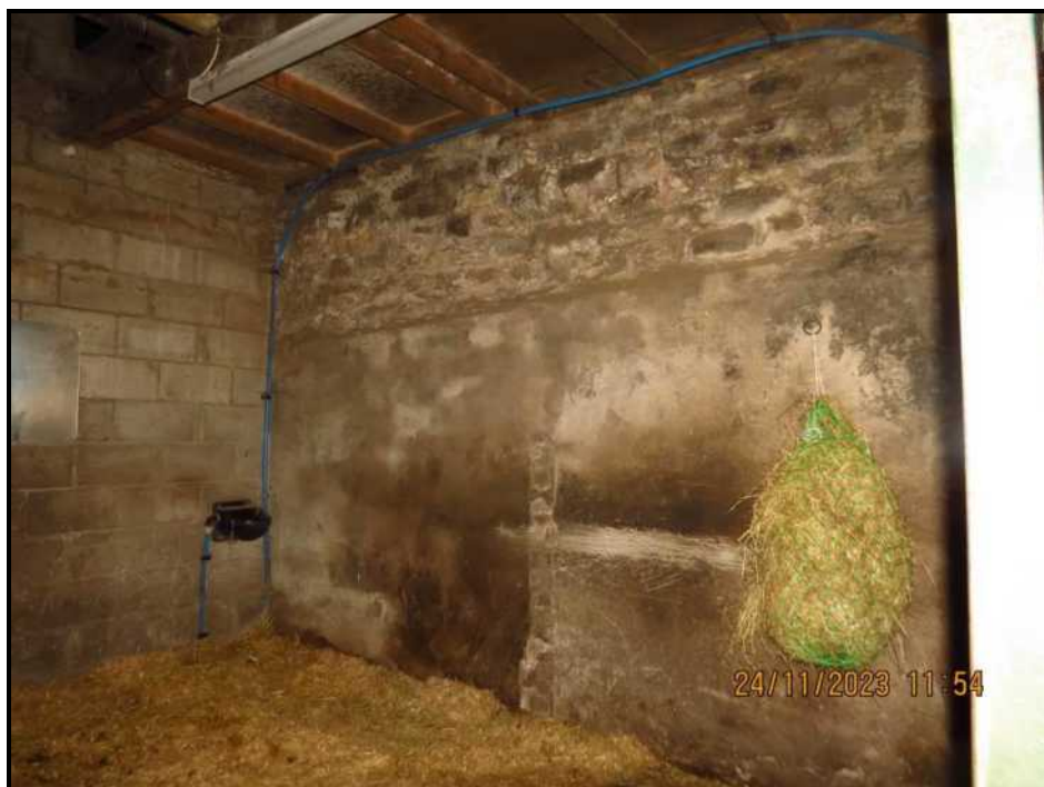
084 Party wall/front wall
