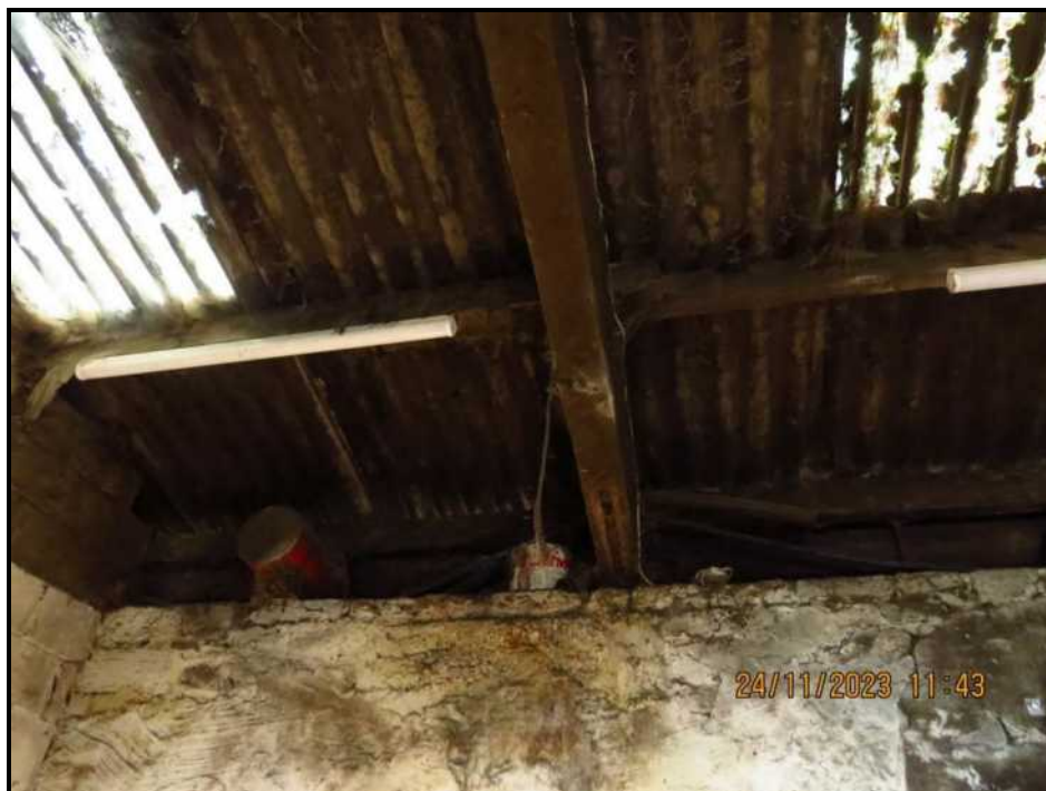
042 Rear wall rafter beam
