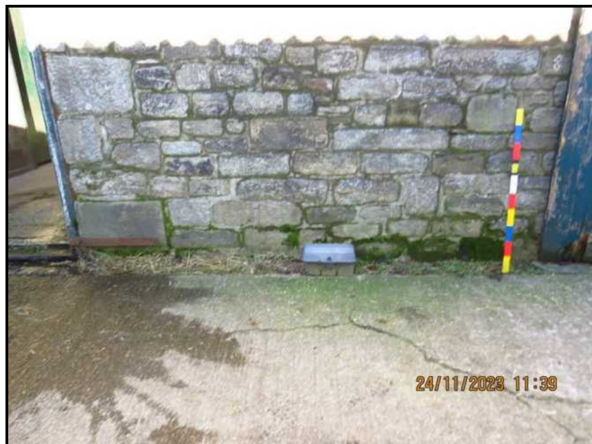
Photograph 032 Plinth wall, chainage 10 – 7 metres
