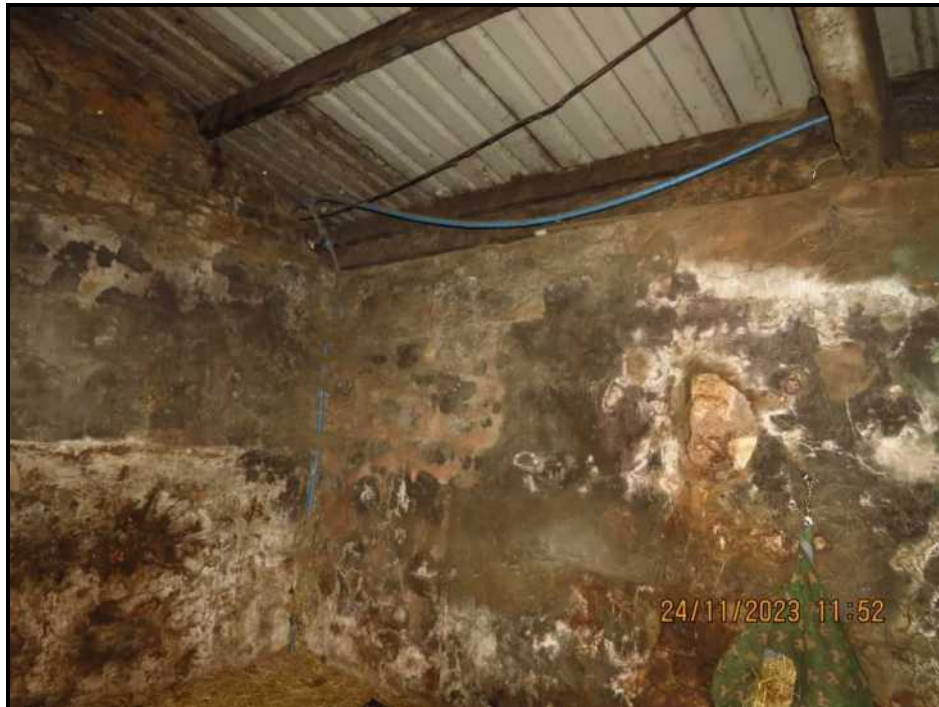
075 Rear wall Unit No. 2
