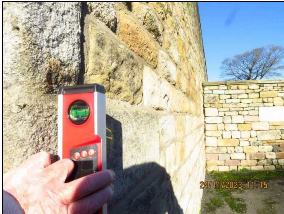
003 Satisfactory vertical alignment
