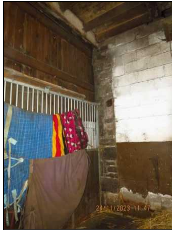
058 Front elevation and internal cross wall
