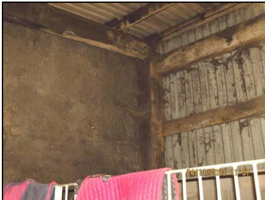
Photograph 093 Outside of West wall
