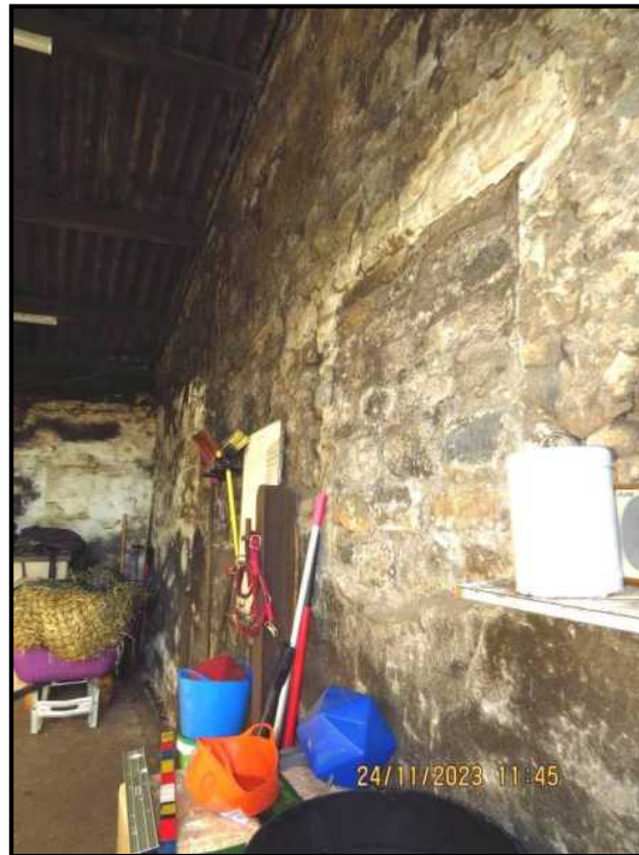
054 Gable elevation looking to rear
