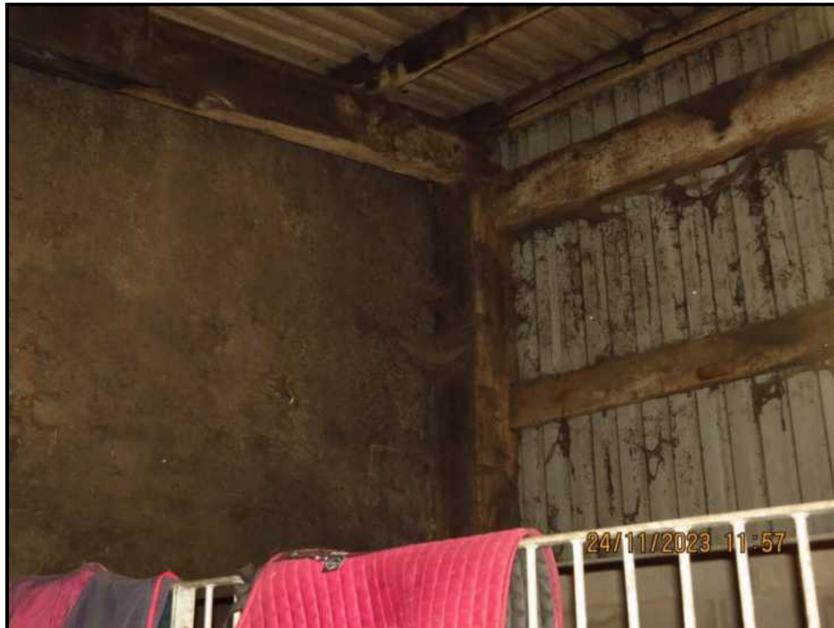
093 'Outside' of Western wall
