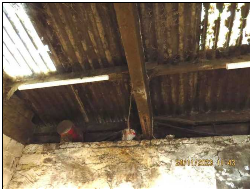
Photograph 042 Rear wall rafter beam
