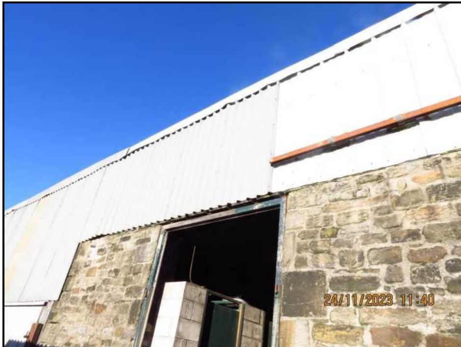
034 Upper wall, chainage 16 – 7 metres
