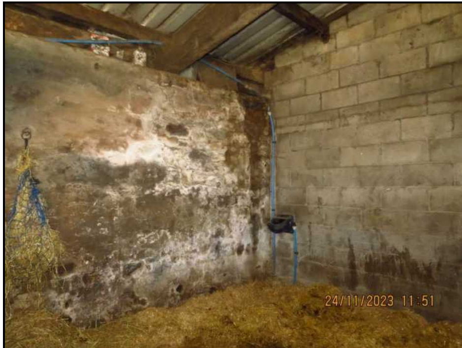
073 Rear wall and party wall, North East corner
