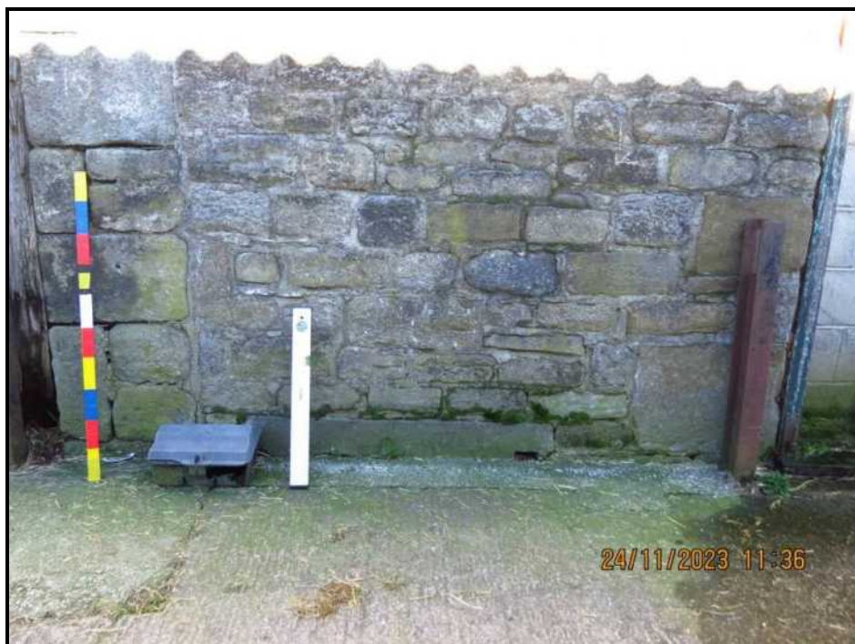
027 Ground floor, chainage 5 – 10 metres
