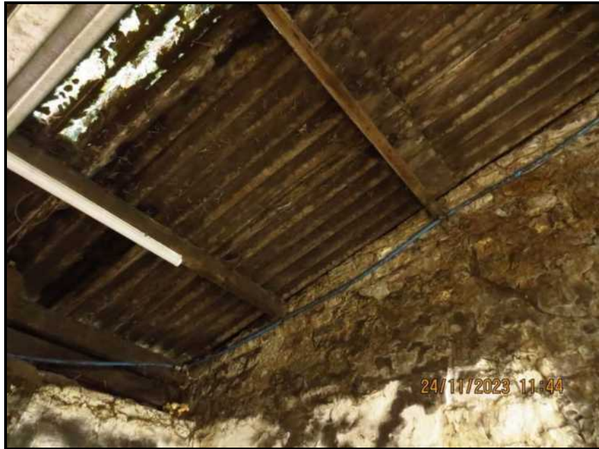
(Photograph 045 Purlin seating Eastern gable
