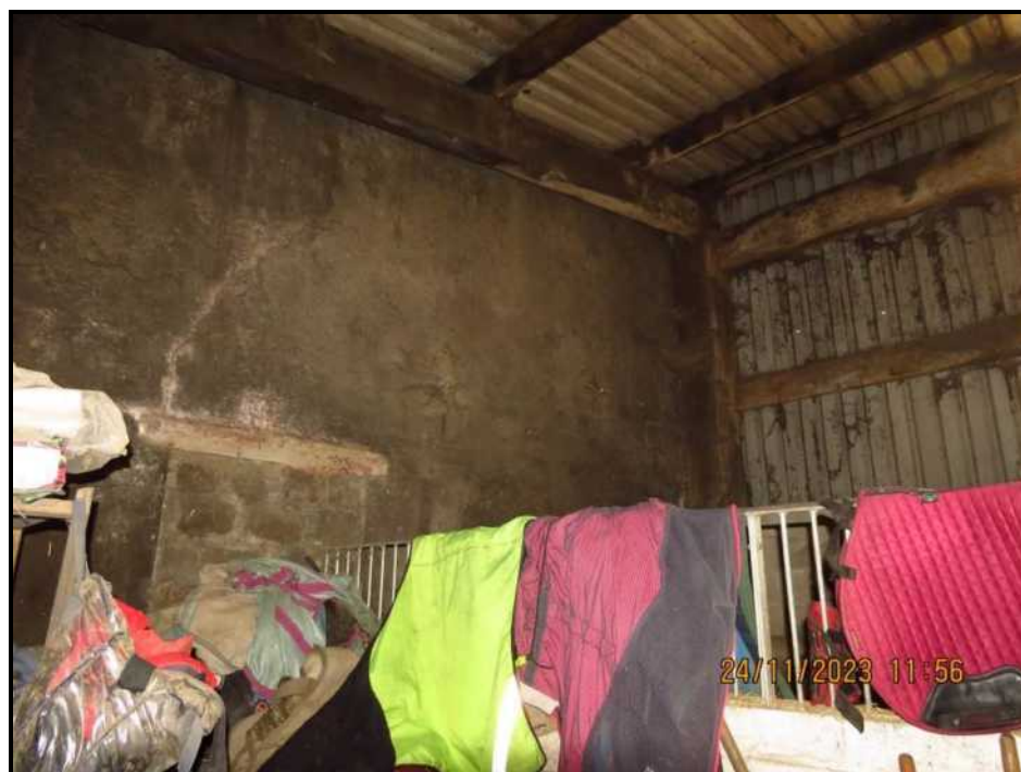
092 'Outside' of Western wall
