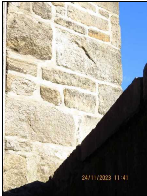
039 South Eastern corner, chainage 1.2 – 0 metres
