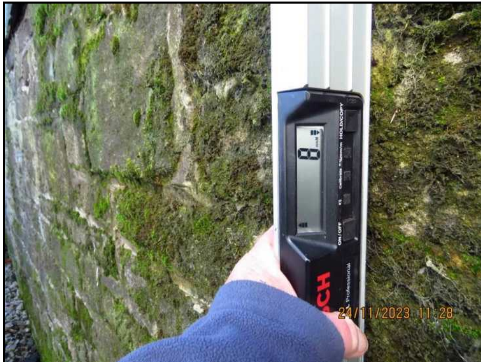
016 Satisfactory vertical alignment, chainage 12 metres
