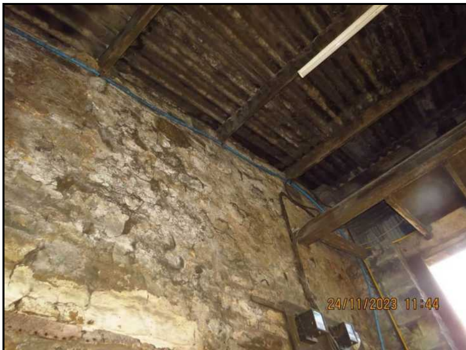
051 Eastern gable, front corner
