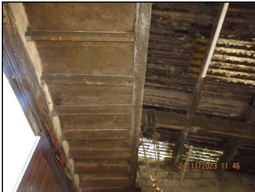
Photograph 056 Front elevation supporting timber detail
