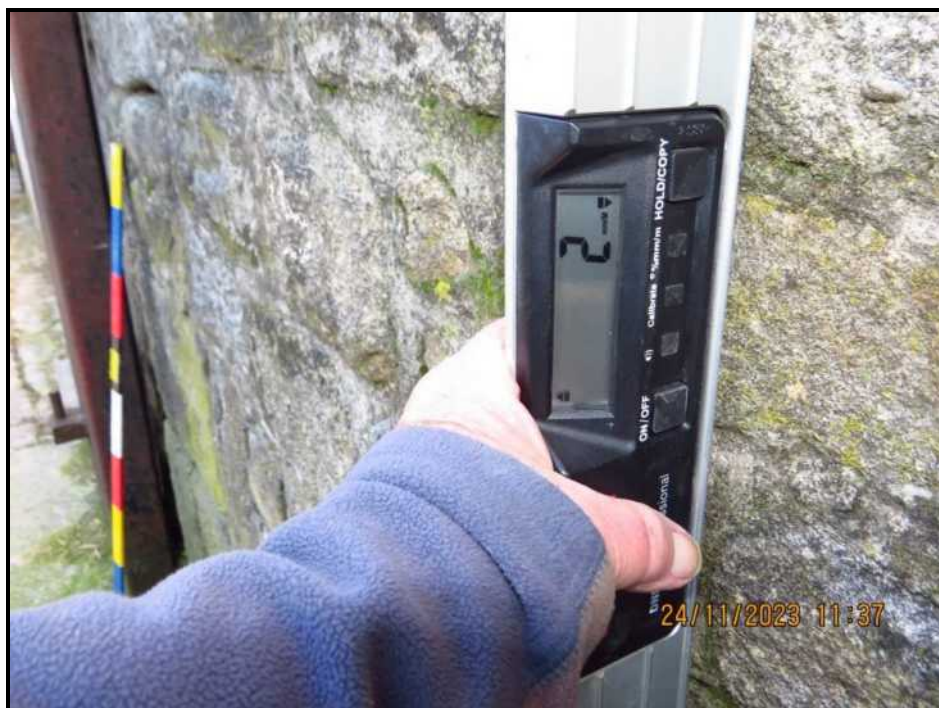
029 Good vertical alignment, 2mm per metre
