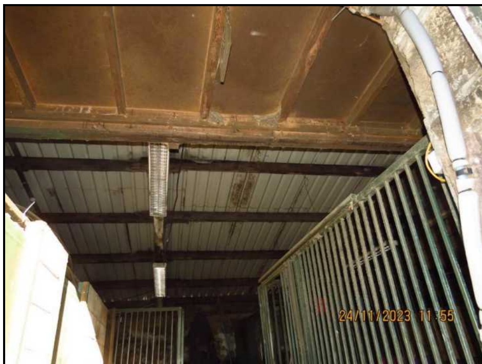
088 Roof, front elevation
