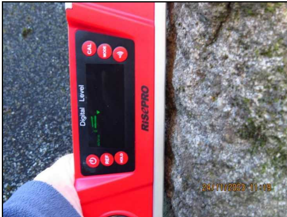
007 Satisfactory vertical alignment 5mm per metre
