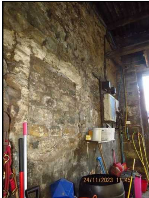
Photograph 053 Former window, internal corner South/East
