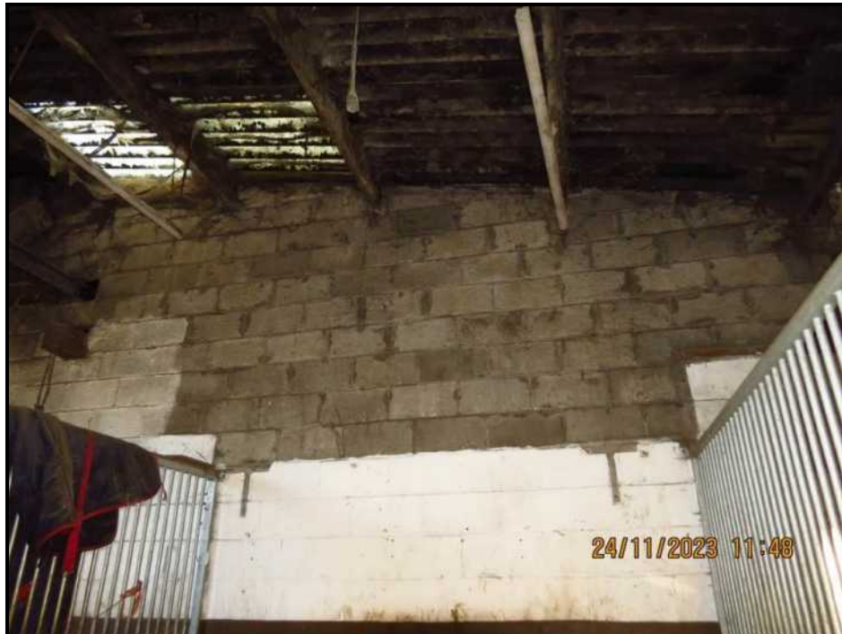
062 Internal party wall with Stable No. 2
