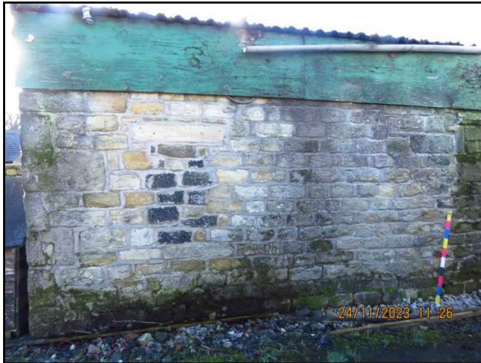
012 Rear wall, chainage 0 – 4 metres
