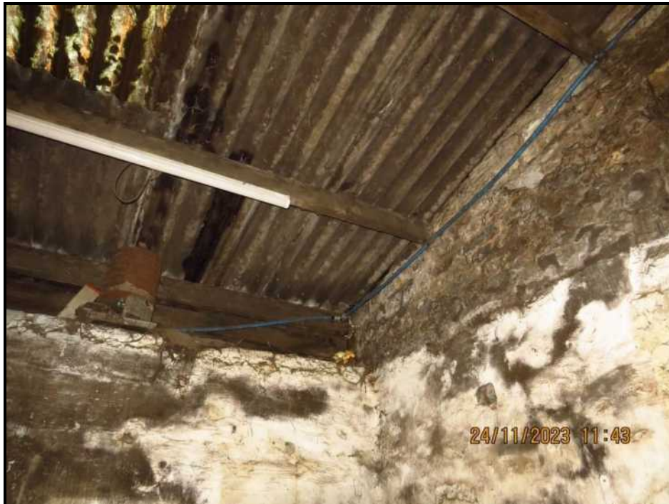
043 Roof, Northern corner
