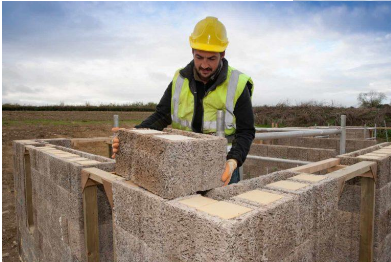
Durisol woodcrete blocks (made from recycled wood)
