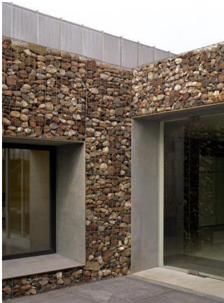
deep reveals to super-insulated walls
