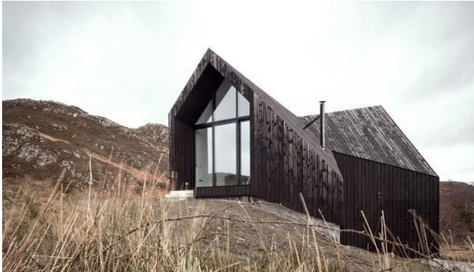
charred timber cladding
