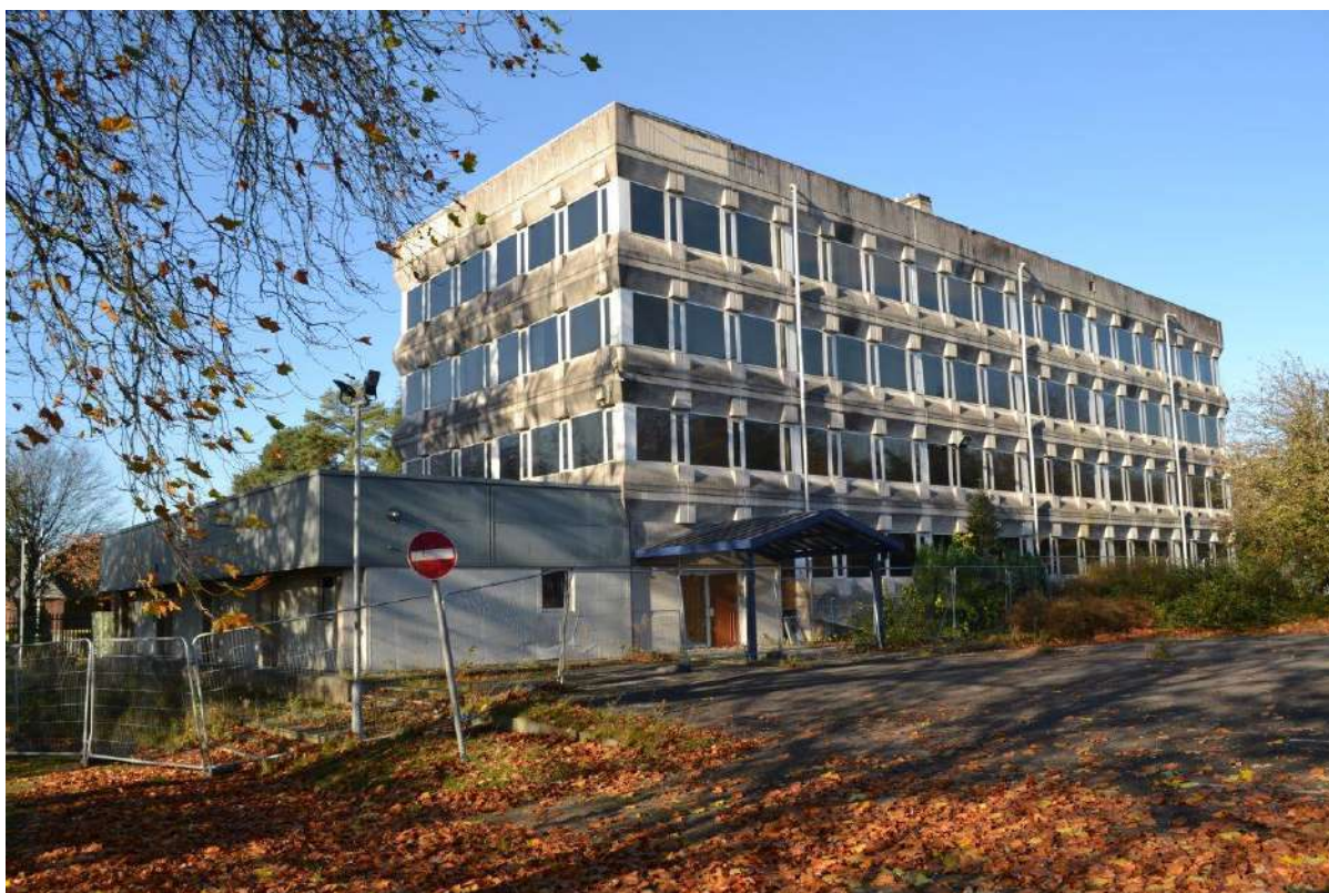
Plate 46: Sightline to the north-west showing the east-facing and south-facing elevations (and the single-storey, flat roof extension) of Parkfield House (non-designated heritage asset).
