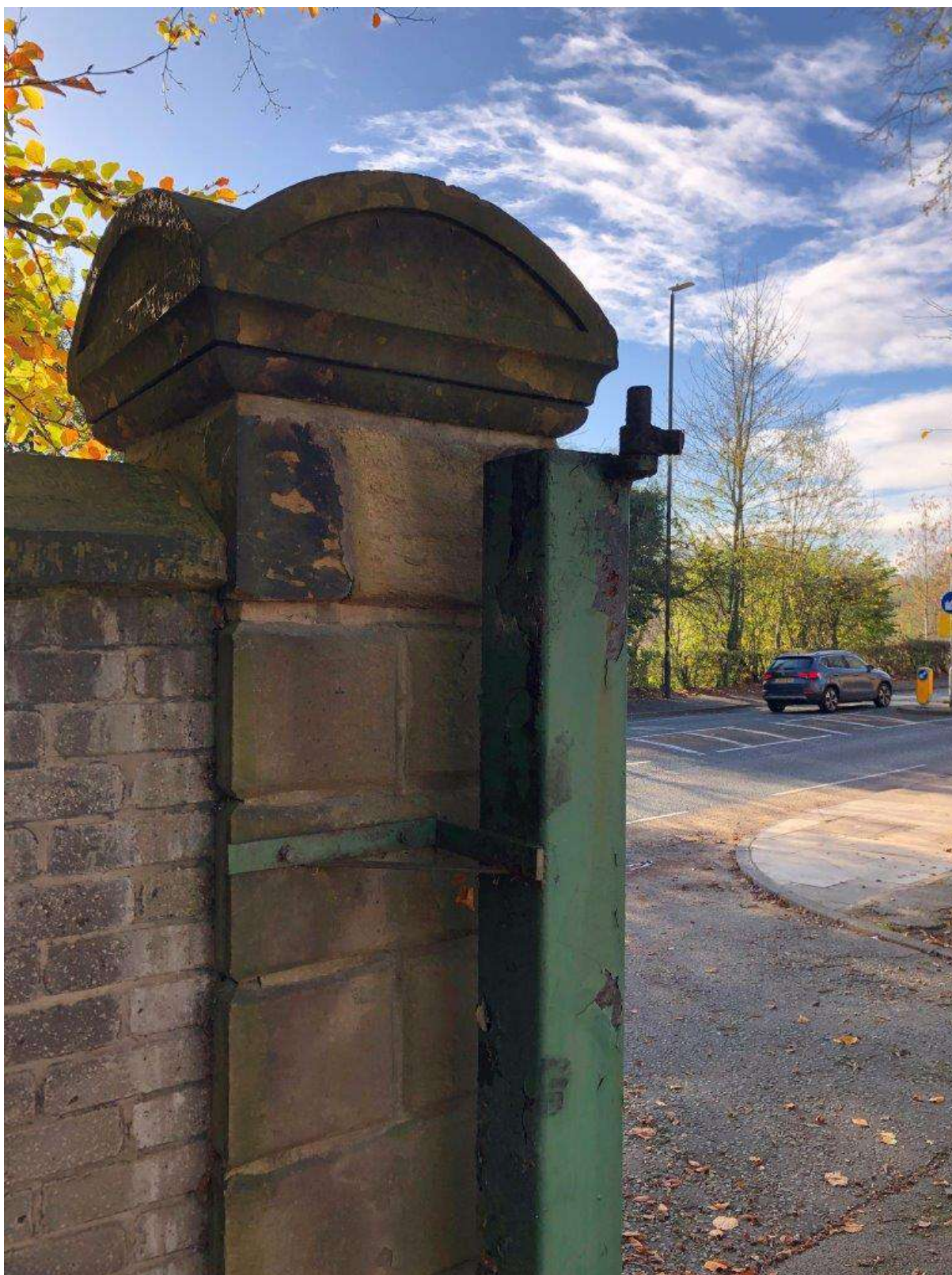
Plate 56: Sightline to the south-west showing detail of the finely tooled and chamfered eastern gate pillar with cast-iron gate post with surviving pintle affixed to the ashlar stonework. Brick-backing to the boundary wall also visible.
