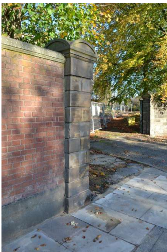
Plate 55: Sightline to the north-east showing the detail of the western-most pillar and its articulation with the boundary wall of the War memorial (Grade I* Listed Building, NHLE ref. 1415410)
