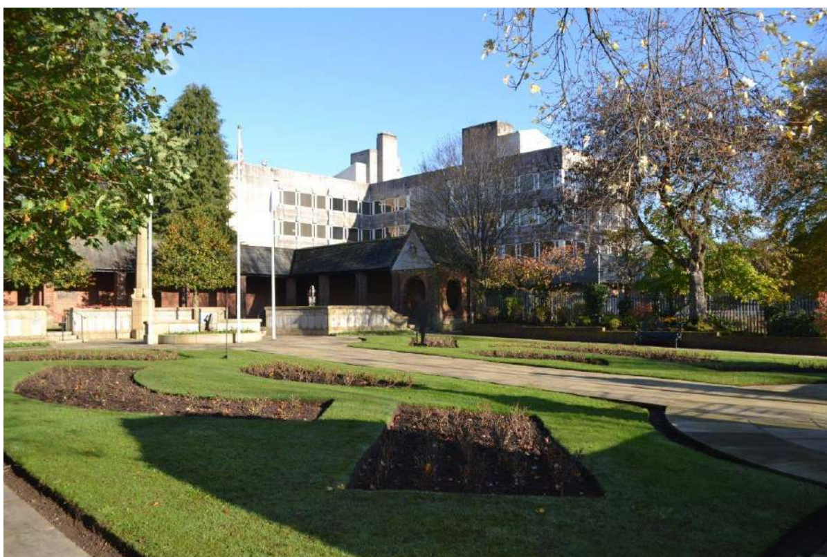
Plate 28: Sightline to the north-east within the War Memorial (Listed Building). Parkfield House is skylined behind.
