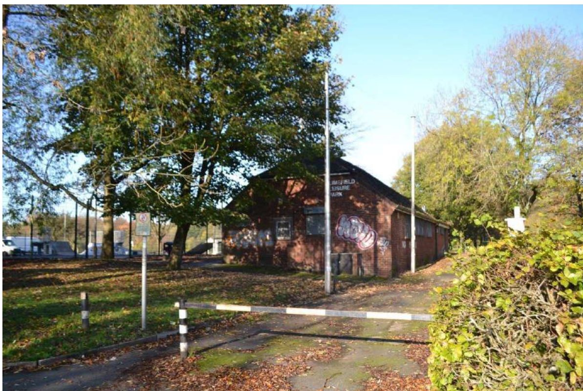
Plate 9: Sightline to the north showing the south-facing and east-facing elevations of the Limefield Leisure Park utility building (non-designate heritage asset).
