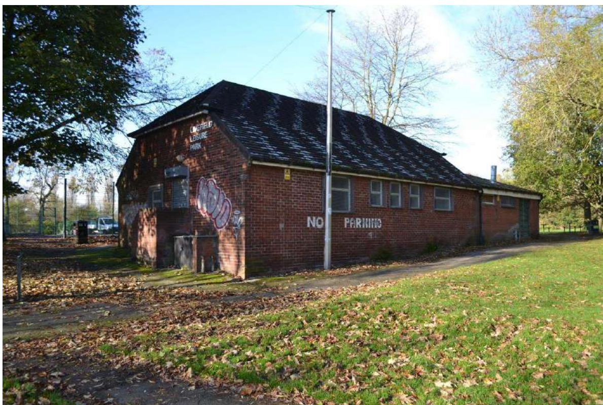
Plate 10: Sightline to the north-west showing the south-facing and east-facing elevations of the Limefield Leisure Park utility building (non-designate heritage asset) and also highlighting the jerkinhead roof.
