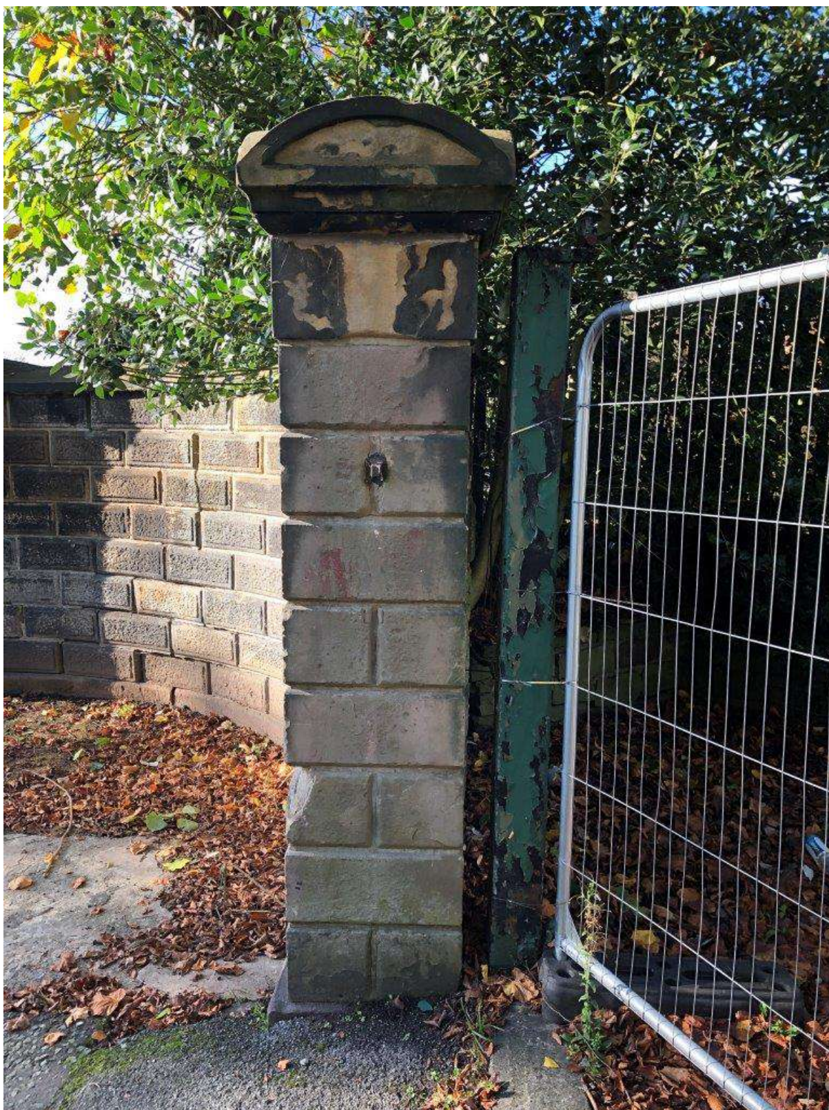
Plate 57: Sightline to the west showing detail of the finely tooled and chamfered western gate pillar Note rough-tooling to panels of the ashlar faces of wall behind to provide a rusticated effect.
