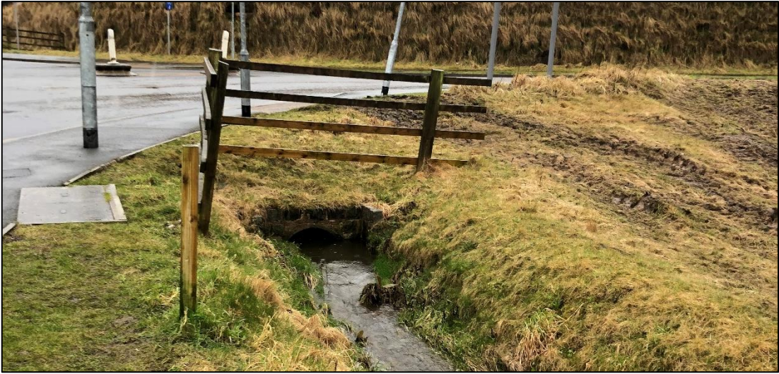
Figure 3.4: Photo taken on downstream end of circular culvert upstream of site, along the eastern boundary. (Photo taken on 10/03/21)
