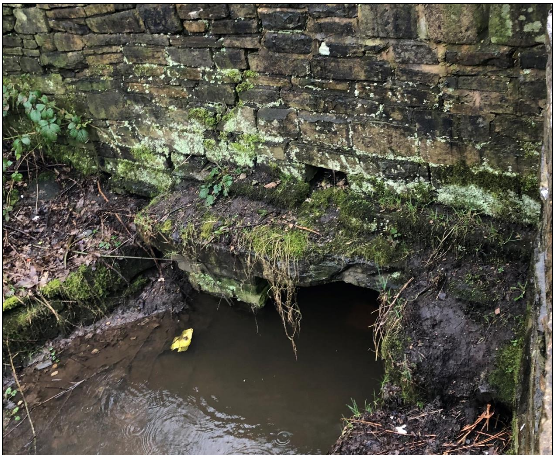
Figure 3.5: Photo taken on downstream end of box culvert downstream of the site, along the eastern boundary. (Photo taken on 10/03/21)
