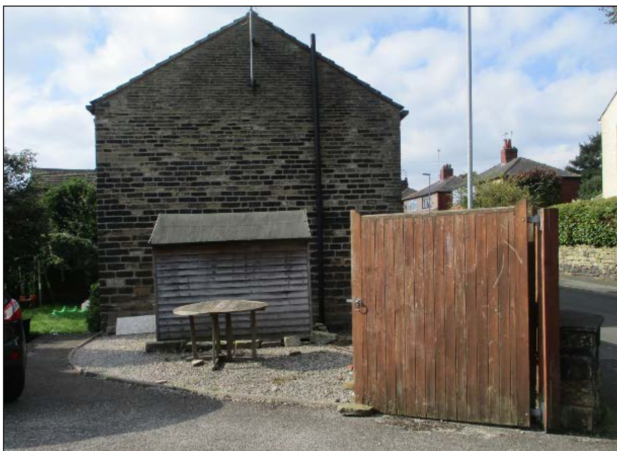
4. Site of the proposed extension, facing the blank side wall of the application property
