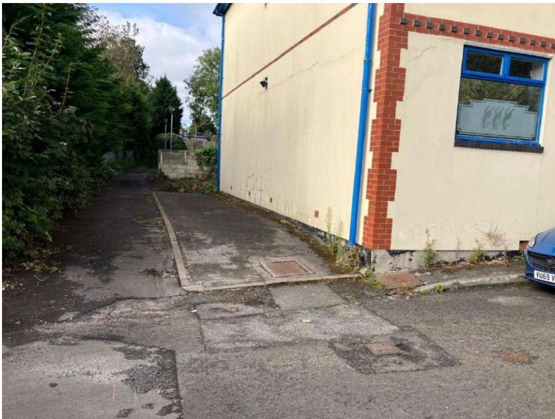
Photograph 2 – View of the developed land / sealed surface along the southern development boundary.
