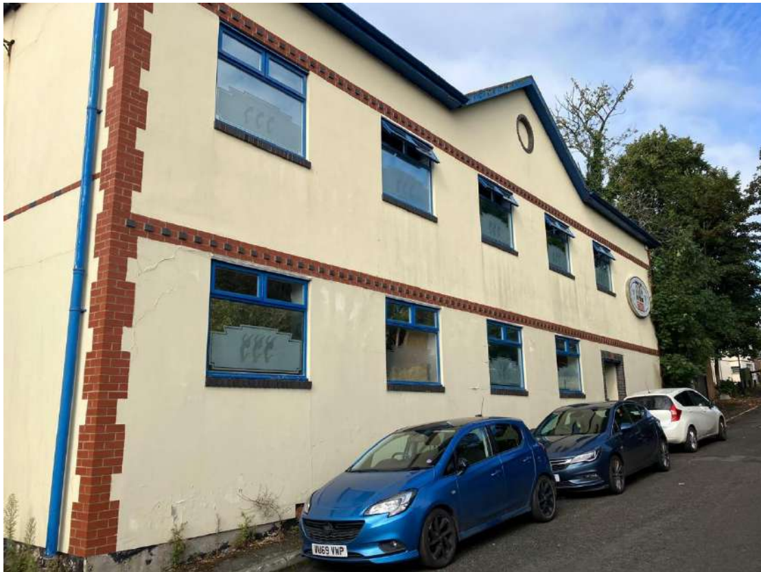
Photograph 3 – Eastern aspect of the building on site.
