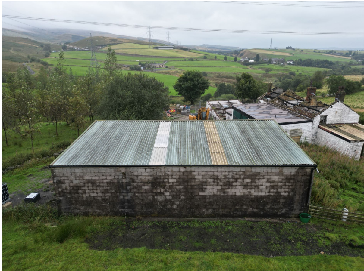
2 – The rear of the building.
