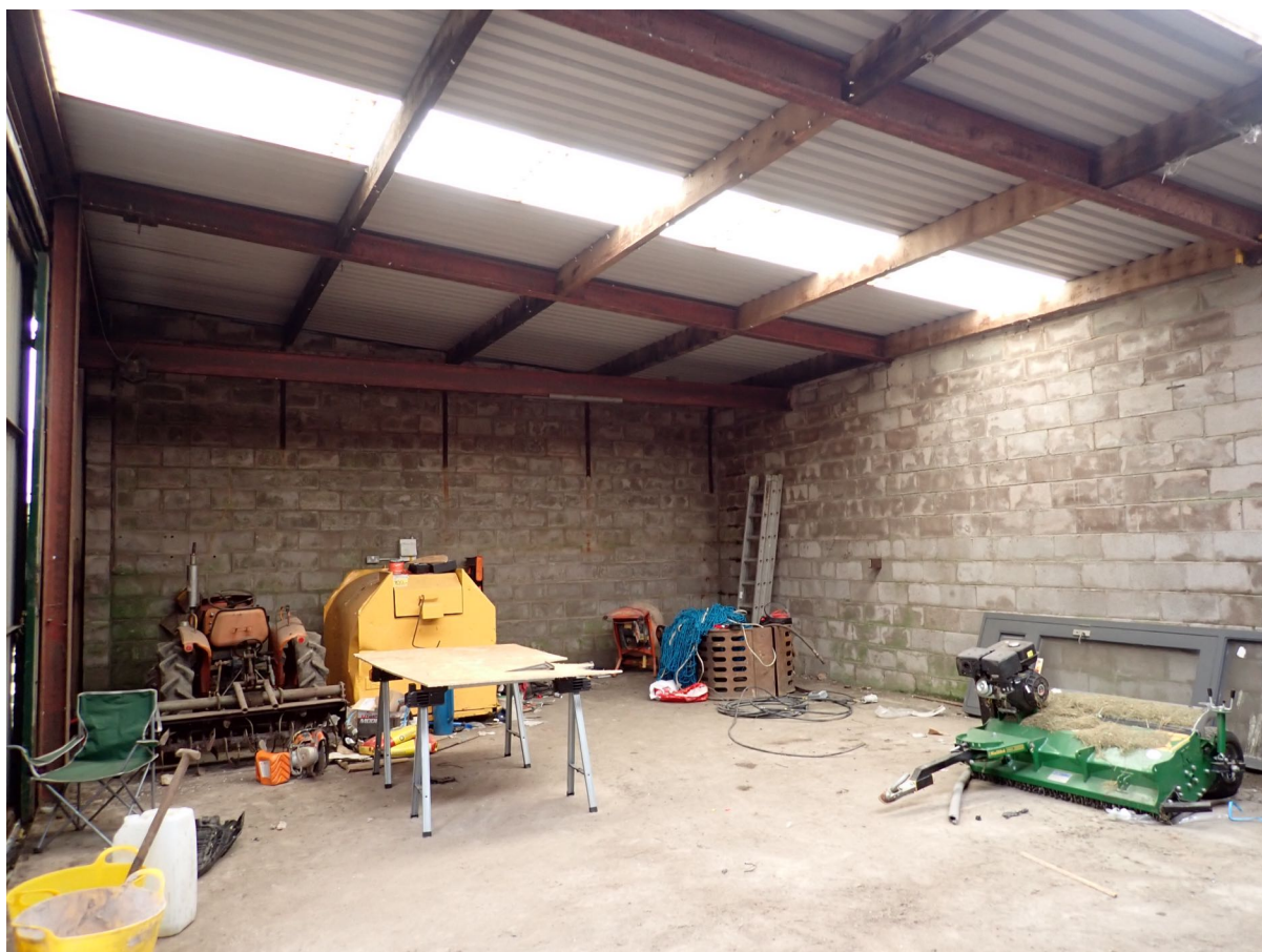
7 – The building has no enclosed spaces and is well-lit by natural light.
