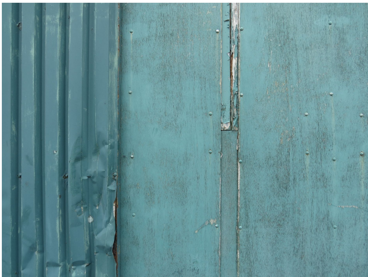
3 – The front walls are a single layer of timber boarding, sliding doors are corrugated steel.
