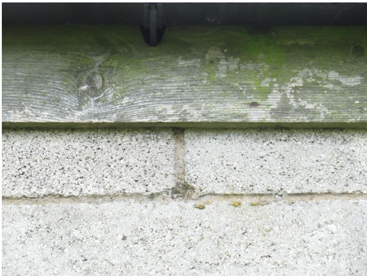
6 – Timber fascia are fitted tightly.
