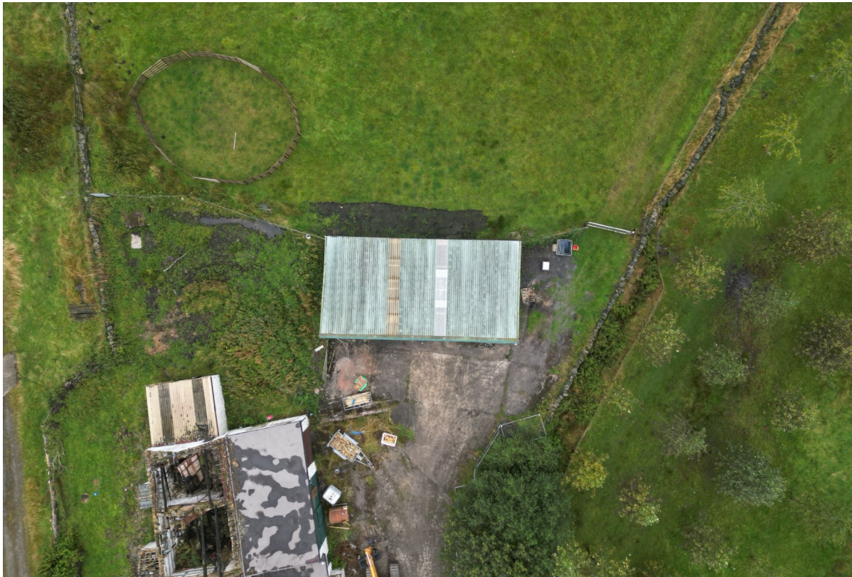
1.6b – Outbuilding rear of Longley Hey Farm – aerial photograph.
