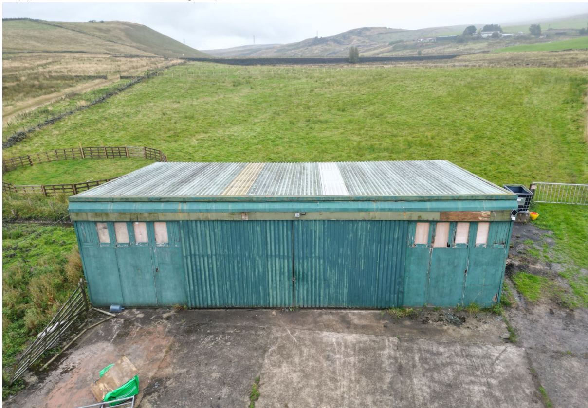
1 – The front of the building.
