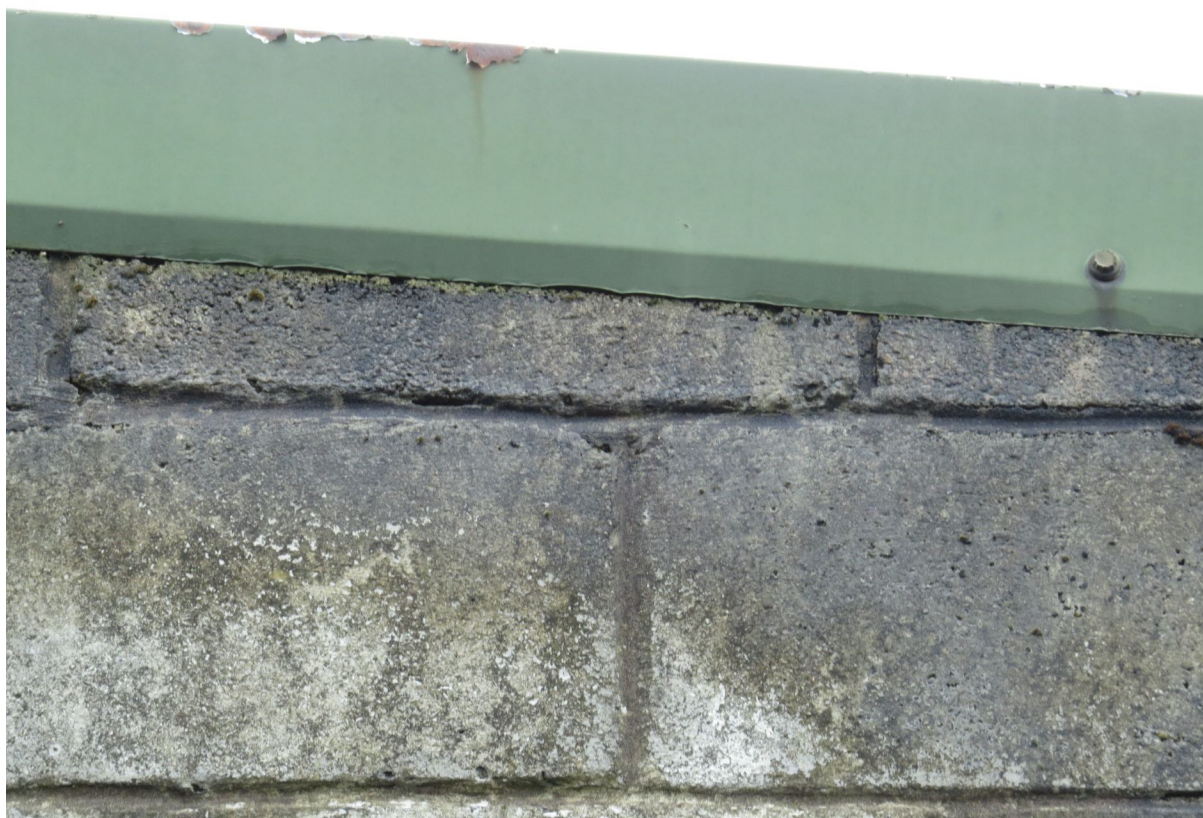
5 – Steel fascia panels are fitted tightly.
