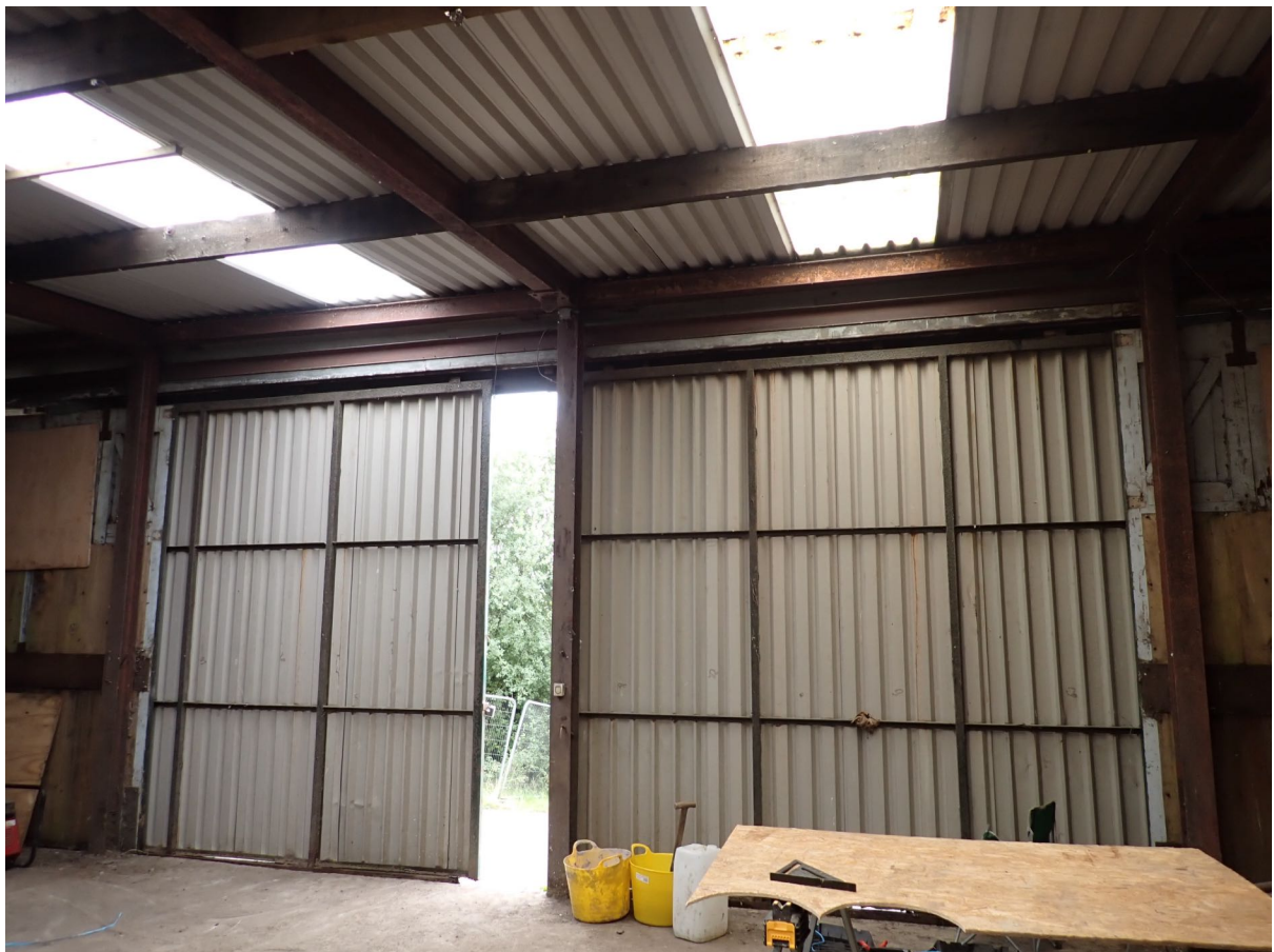
10 – The front doors and walls are of single layered materials with no enclosed crevices.
