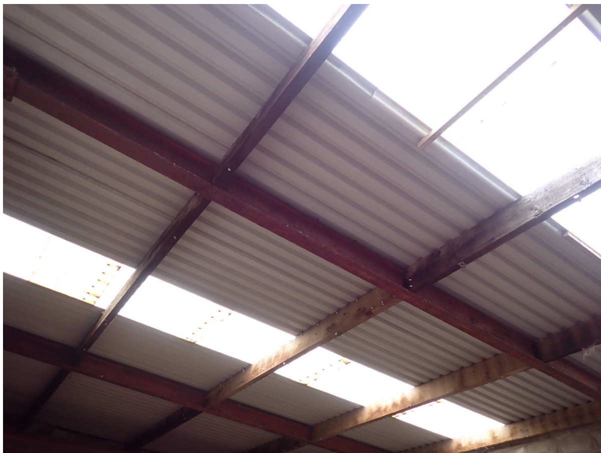
8 – The roof has a simple steel and timber structure with no insulation.
