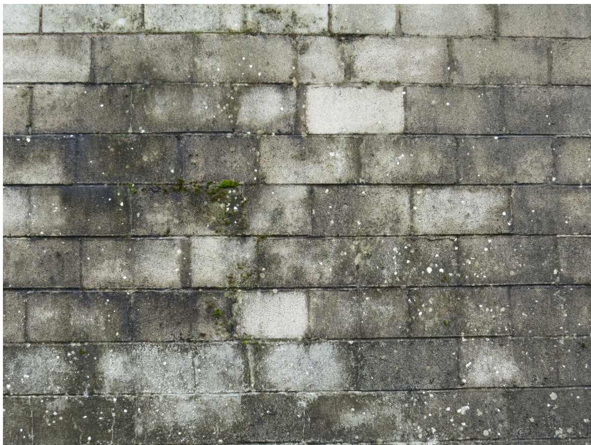
4 – Side and rear walls are a single layer or solid concrete blocks.
