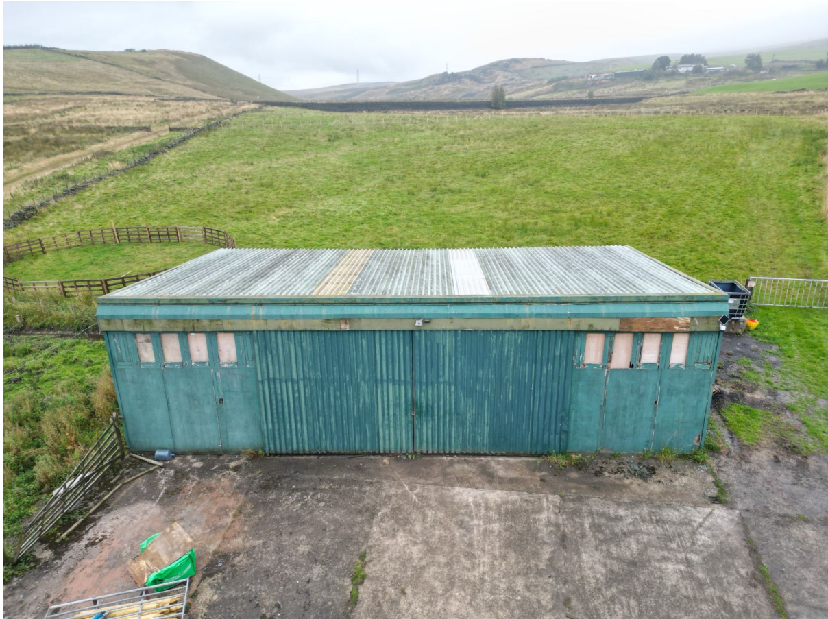
3.1a – Looking north toward the front of outbuilding.
