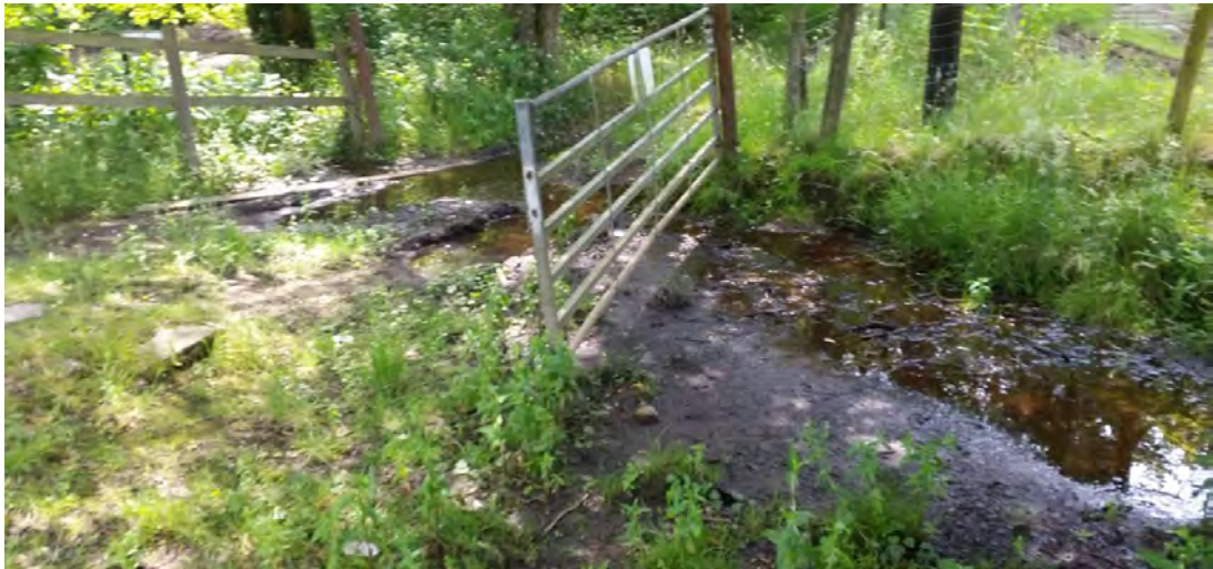
Figure 4.7: Location where ditch spills over access track prior to discharge location to pond to the south
