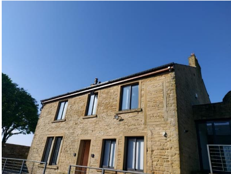
PLATE 1 SHOWING NORTH EASTERN ASPECT OF BUILDING 1
