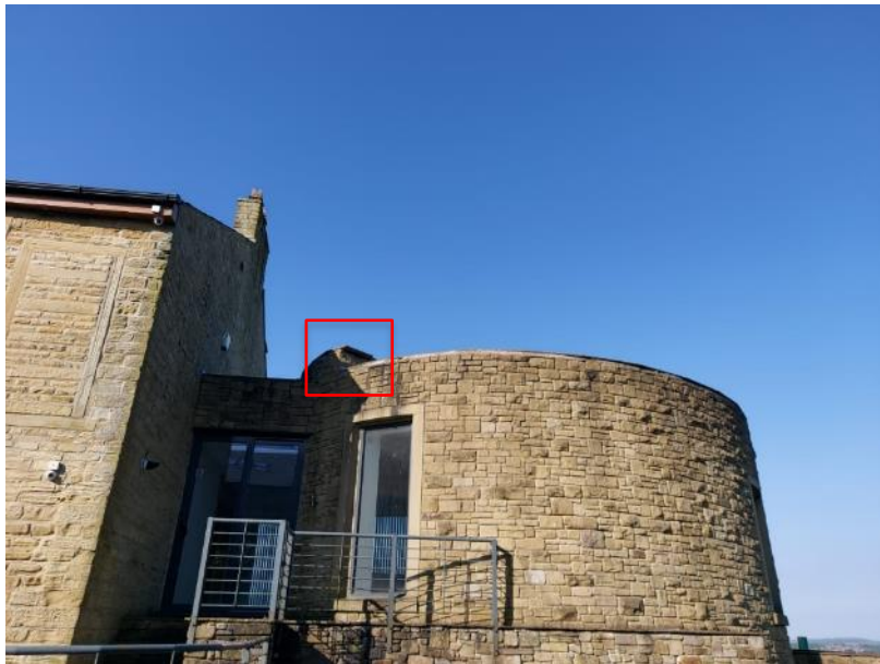
PLATE 7 SHOWING NORTH EASTERN FACING ASPECT OF BUILDING 1A
