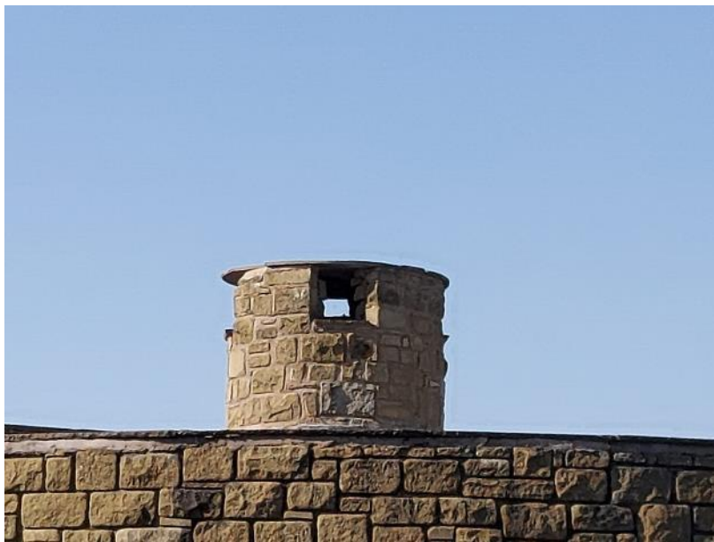
PLATE 9 SHOWING CHIMNEY AT CENTRE OF BUILDING 1A
