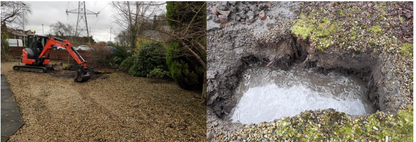
Site investigation photos February 2024 - Trial Hole TH3.
