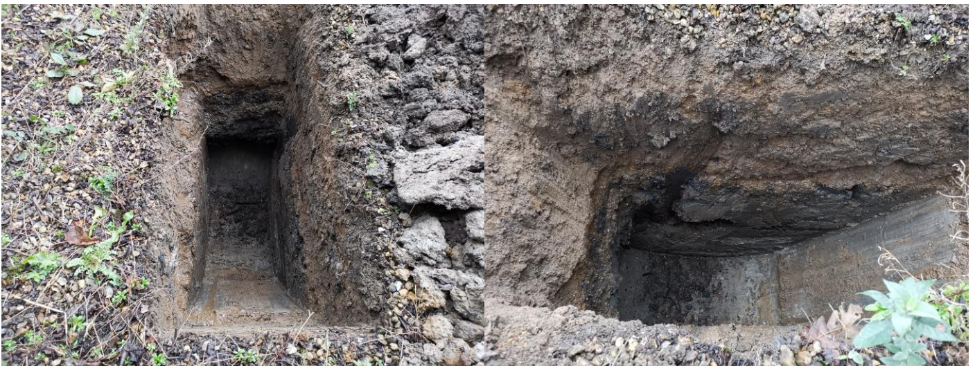
Site investigation photos February 2024 - Trial Hole TH3.
