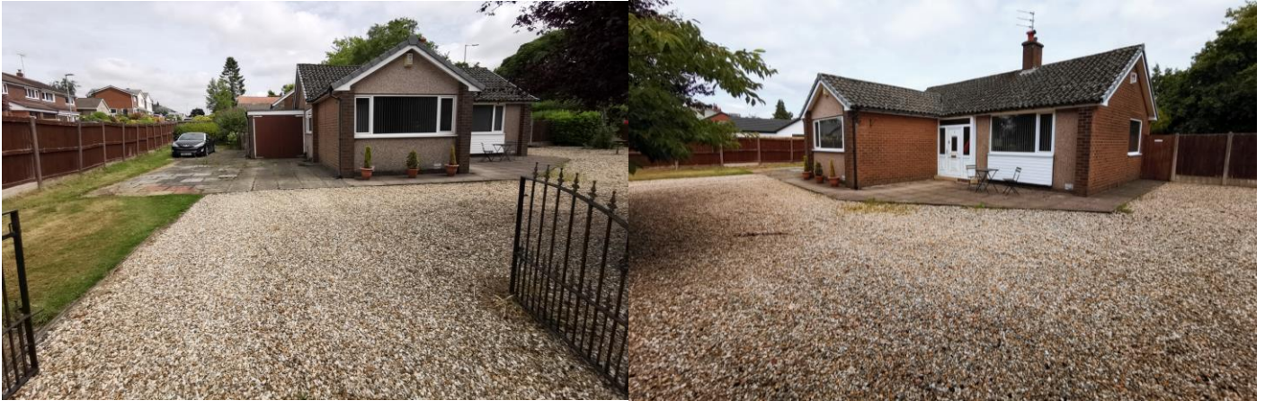
Reconnaissance photos July 2022.
