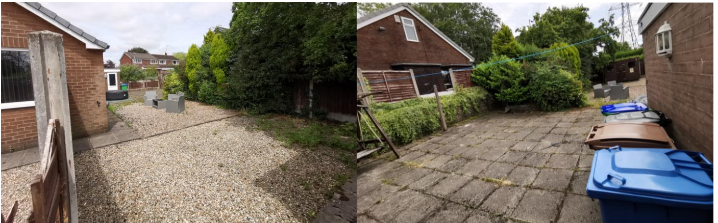
Reconnaissance photos July 2022.
