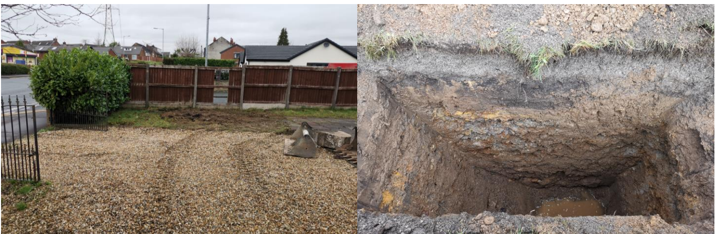
Site investigation photos February 2024 - Trial Hole TH1.
