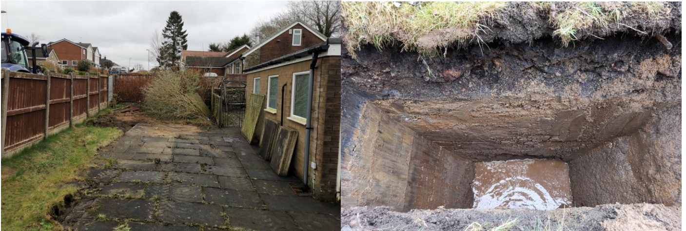
Site investigation photos February 2024 - Trial Hole TH2.
