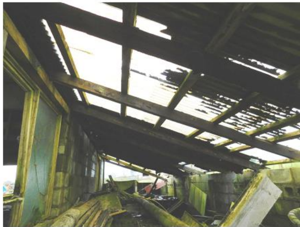
PHOTO 15 Underside of Lean-to Roof
