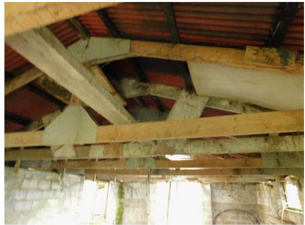
PHOTO 14 Underside of Main Building Roof
