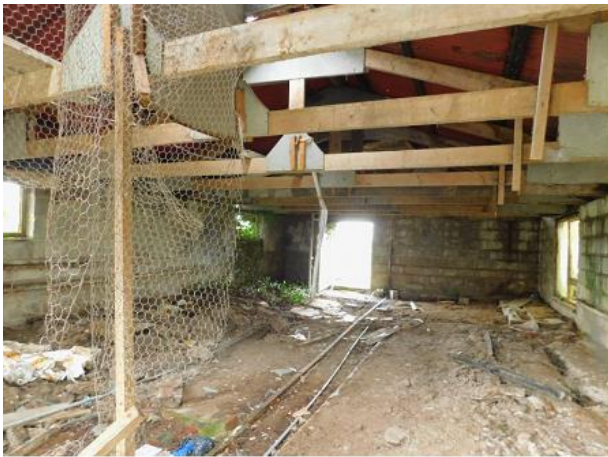
PHOTO 13 View Within Main Building
