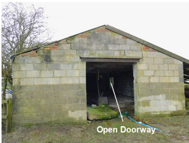
PHOTO 3 Eastern Elevation of Main Barn
