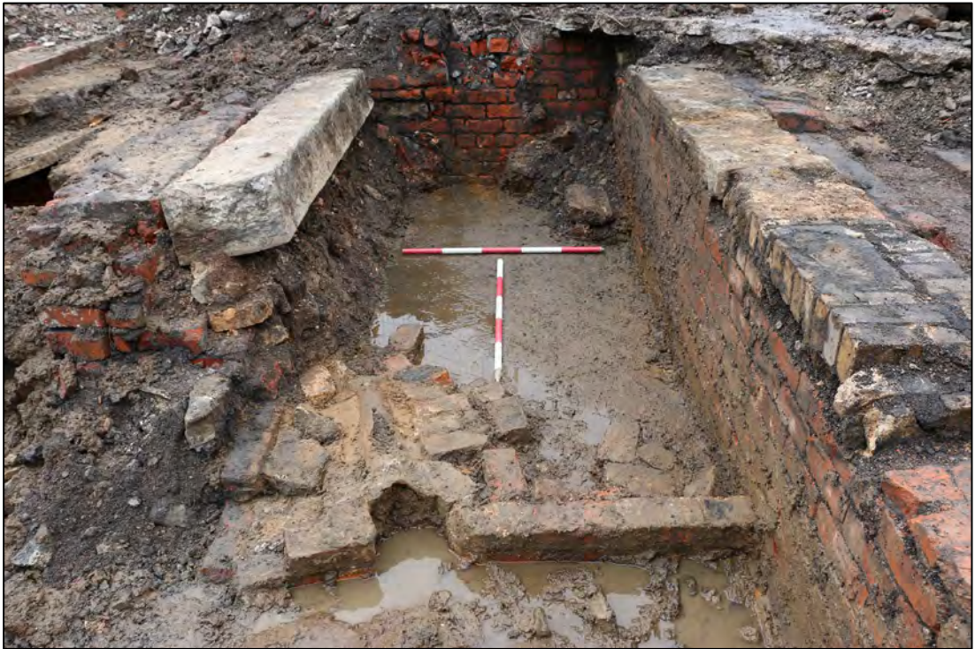
Plate 48 Shot of walls [4015] (left), [4020] in the foreground, [4014] in the background and [4013] (right), and surface [4019], looking south. Scales = 2 x 1m.
