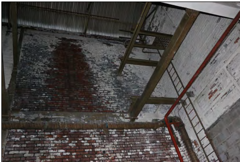
Photograph 10: Internal space of the tower in Building 1, looking north-west.
