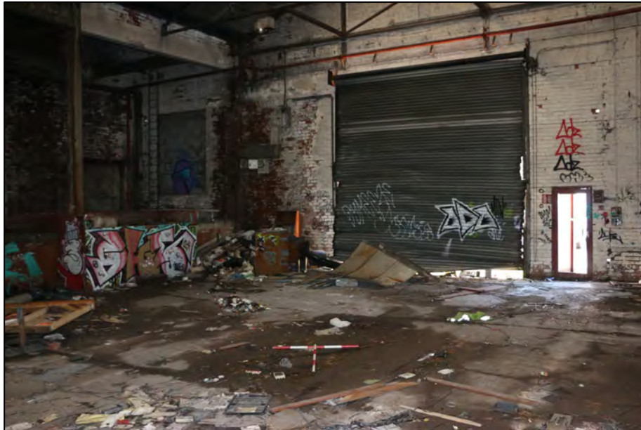
Photograph 7: Internal space of Building 1, looking south-east. Scale = 2 x 1m.
