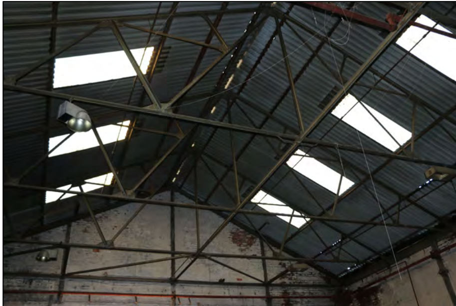
Photograph 11: Roof joists in Building 1, looking south-west.
