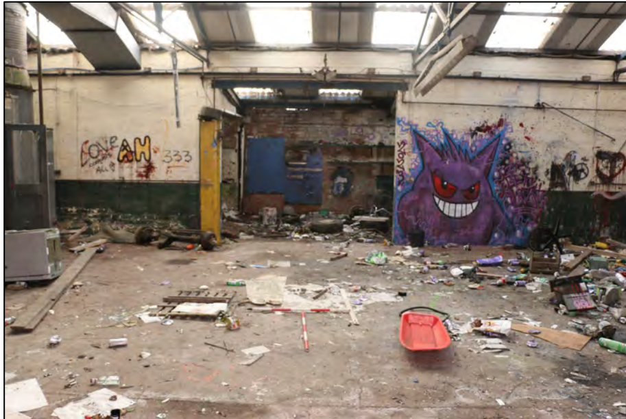
Photograph 18: Opening from the southern room of Building 2 to the northern room, looking north. Scales = 2 x 1m.
