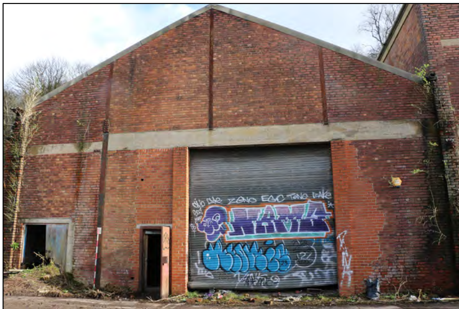
Photograph 2: Southern elevation of Building 1, looking north. Scale = 1 x 2m.
