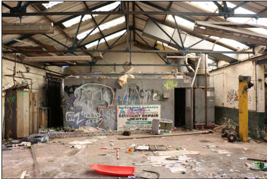
Photograph 16: Internal space of Building 2 showing the construction of smaller room, looking west. Scale = 2 x 1m.
