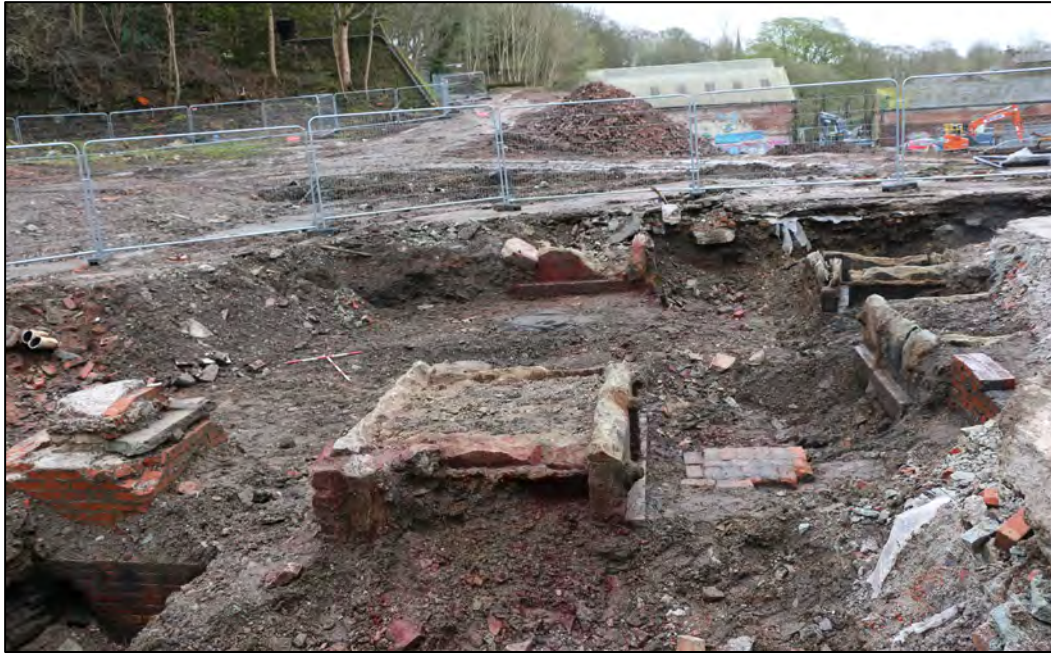
Plate 36 General shot of Area A, showing a series of stone-lined tanks looking south-east.
