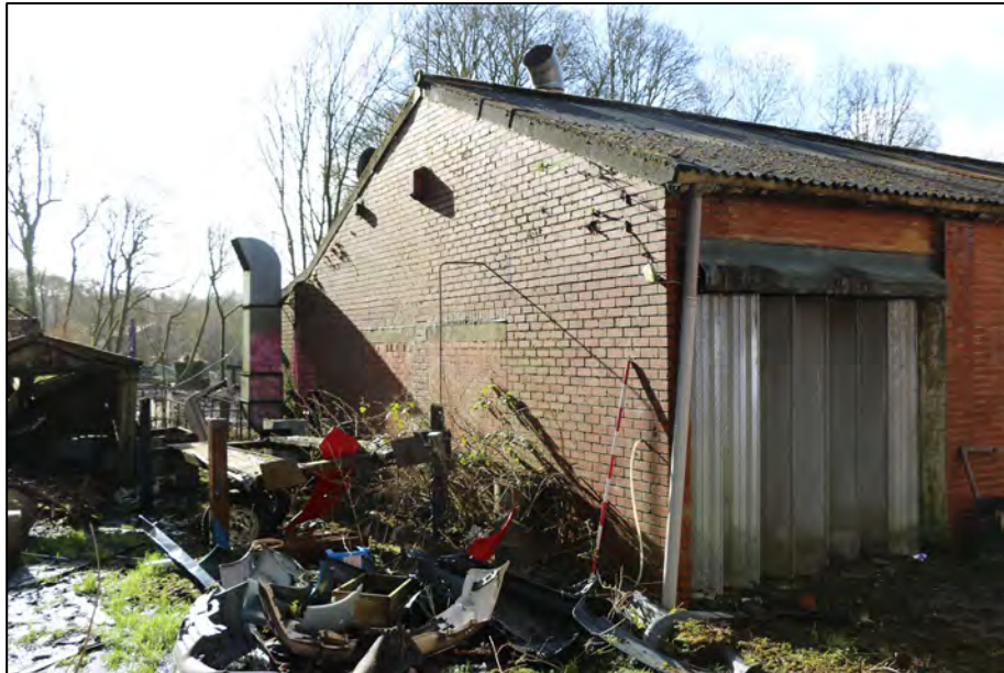
Photograph 15: Northern elevation of Building 2, looking south-east. Scale = 1 x 2m.
