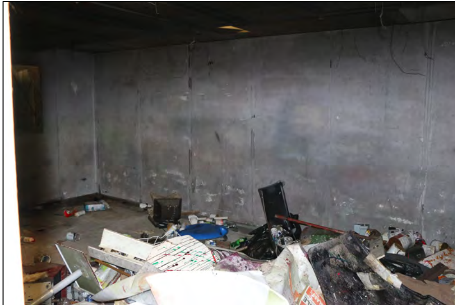
Photograph 17: Internal space of the metal room in Building 2, looking north-west.
