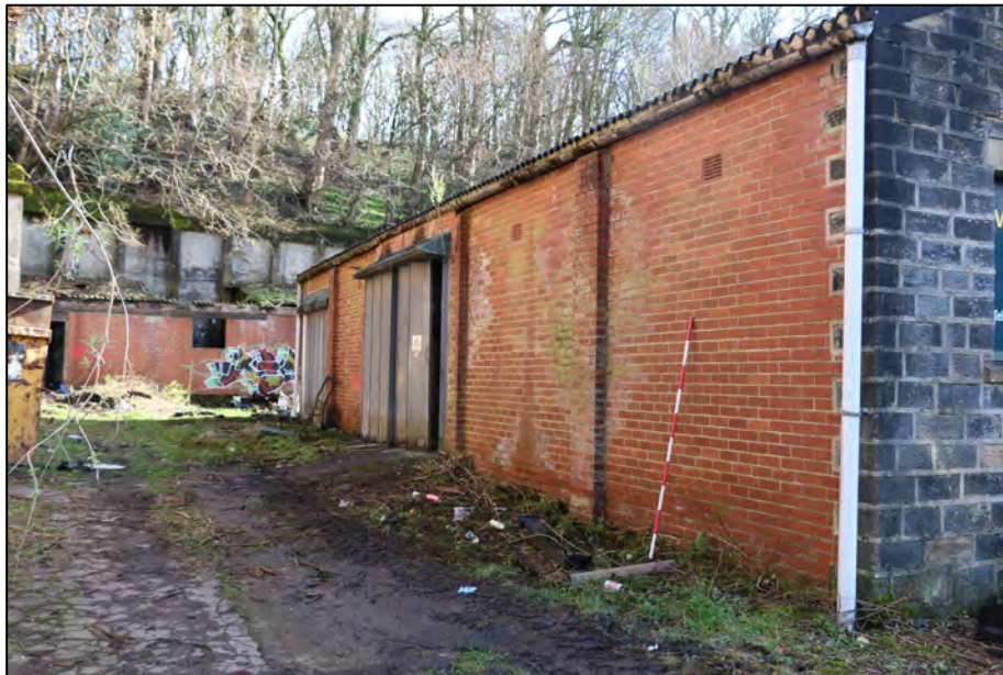
Photograph 13: Western elevation of Building 2, looking north-east. Scale = 1 x 2m.
