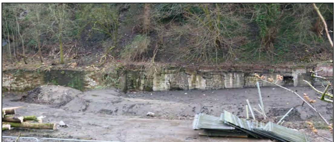
Plate 57 Shot of extant 19 th century walls in southern area of Site, looking north. Scale = 1 x 2m
