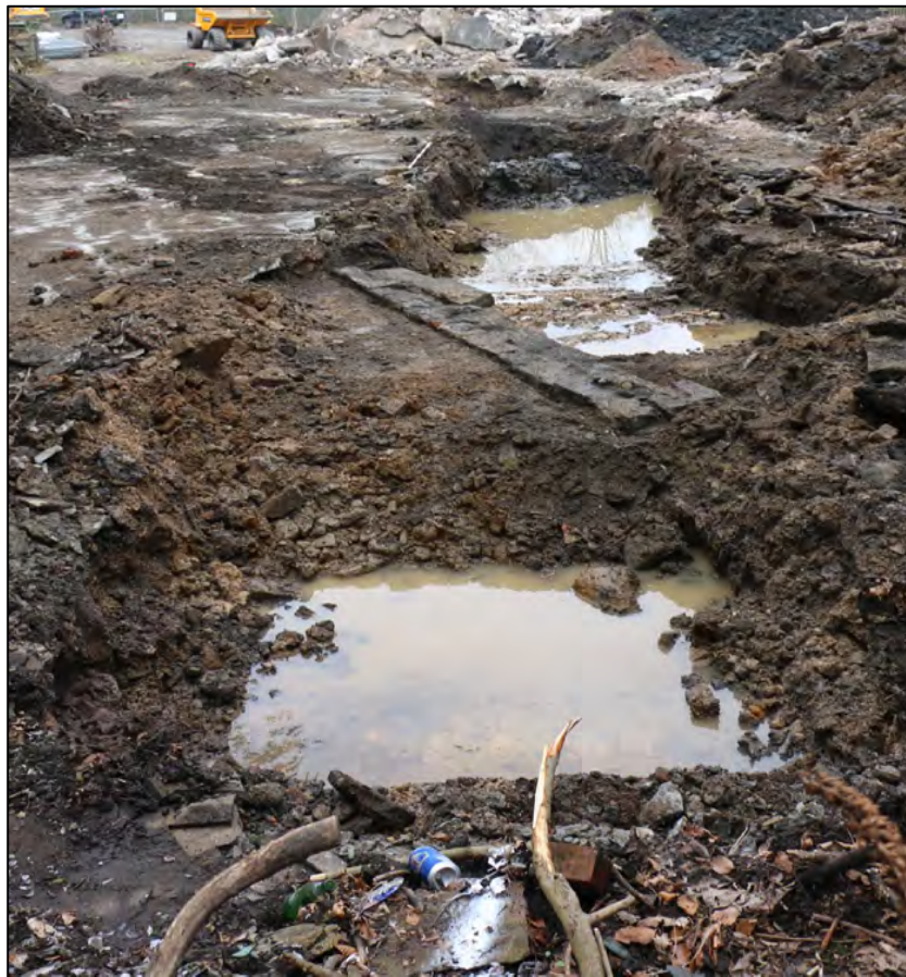
Plate 26 General shot of Trench 8, looking south-south-east. Scale = 1 x 2m.
