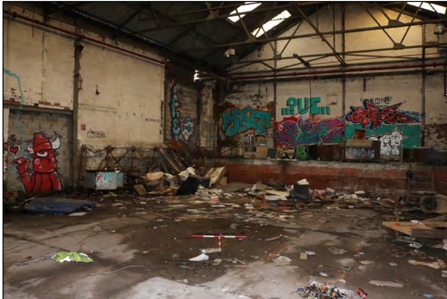
Photograph 9: Internal space of Building 1, looking north-west. Scale = 2 x 1m.
