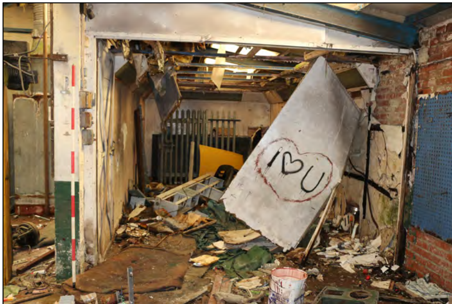
Photograph 20: Western end of the northern room of Building 2, looking west. Scales = 1 x
