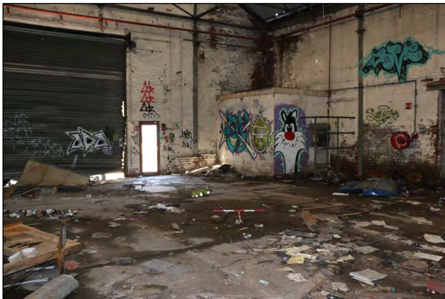
Photograph 6: Internal space of Building 1 showing the construction of smaller room, looking south-west. Scale = 2 x 1m.
