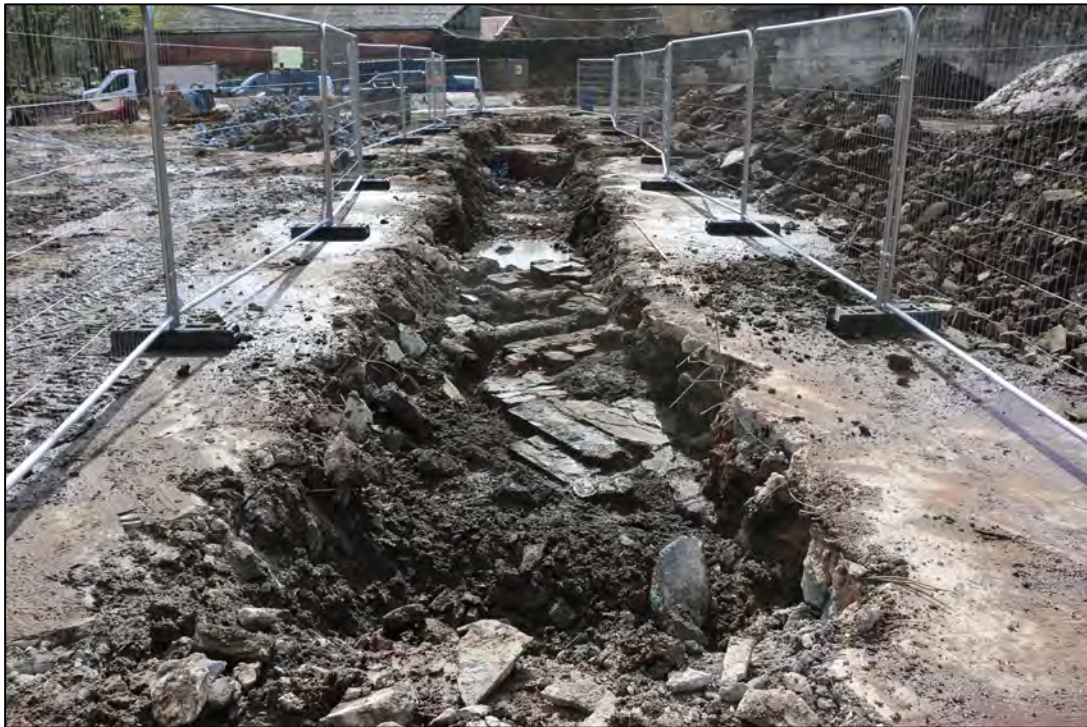
Plate 16 General shot of Trench 5, looking south-east. Scale = 1 x 2m.
