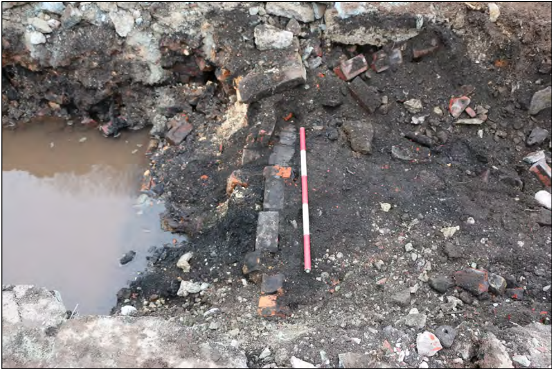
Plate 24 Shot of poorly preserved wall [604], also showing flooded area that covered surface [607]
