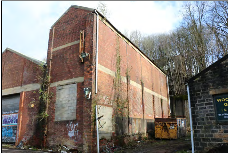
Photograph 5: Eastern elevation of Building 1 tower, looking north-west. Scale = 1 x 2m.
