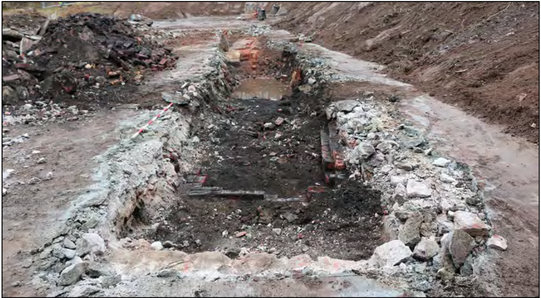
Plate 22 General shot of Trench 6, looking north-west, showing concrete [606] and modern wall [605] in the foreground. Scale = 1 x 2m.
