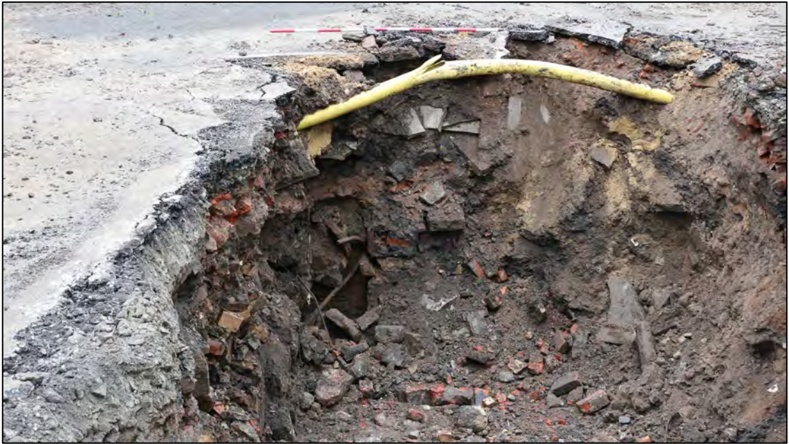
Plate 34 Shot of wall [1005] partly visible in the north-east end of the trench, looking south-west
