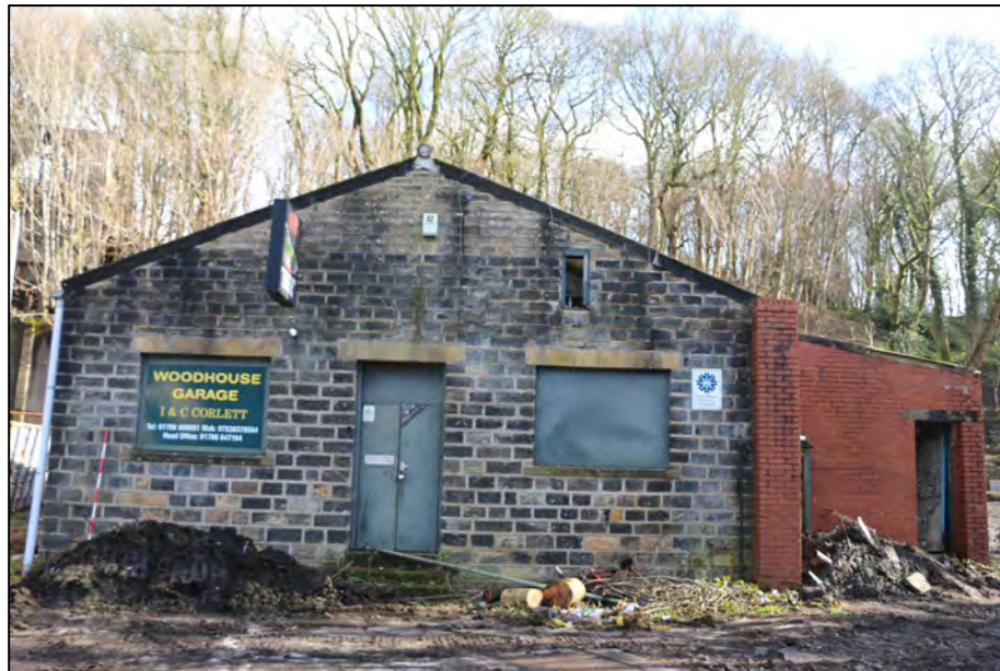
Photograph 12: Southern elevation of Building 2, looking north. Scale = 1 x 2m.
