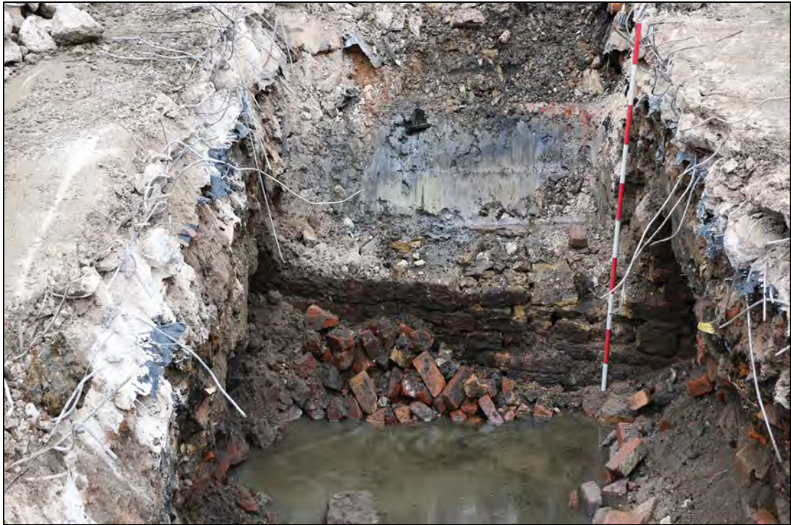
Plate 31 South-west elevation of reservoir wall [904], looking north-east. Scale = 1 x 2m.
