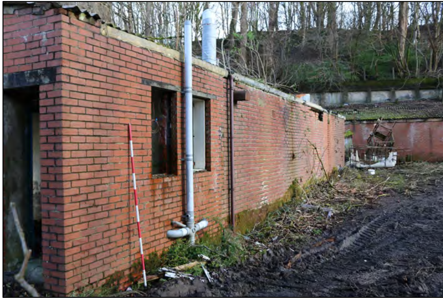
Photograph 14: Eastern elevation of Building 2, looking north-west. Scale = 1 x 2m.
