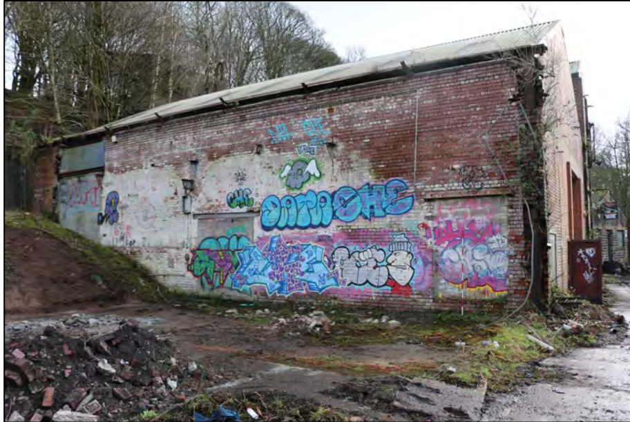
Photograph 4: Western elevation of Building 1, looking north-east. Scale = 1 x 2m.
