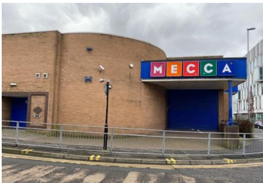
Customer access point into the building
