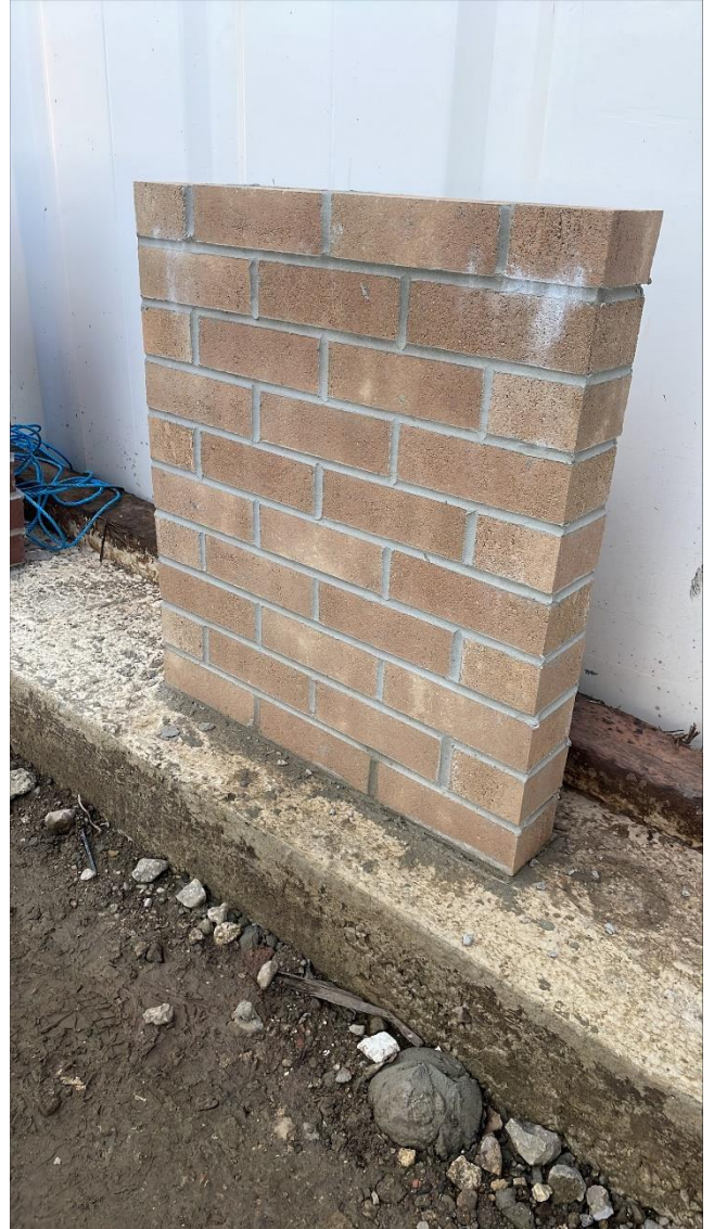
Brick Panel constructed on site.
