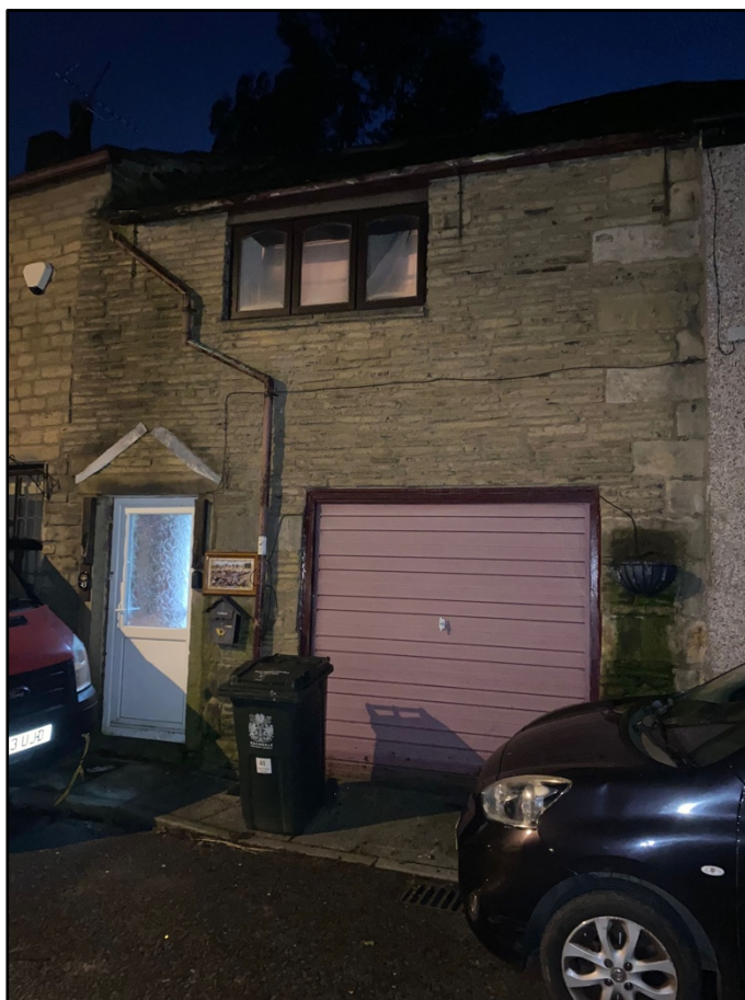
Plate 3: No. 43, a garage door replaced the original window © Client
