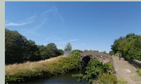
4. Existing bridge to the North of the site.
