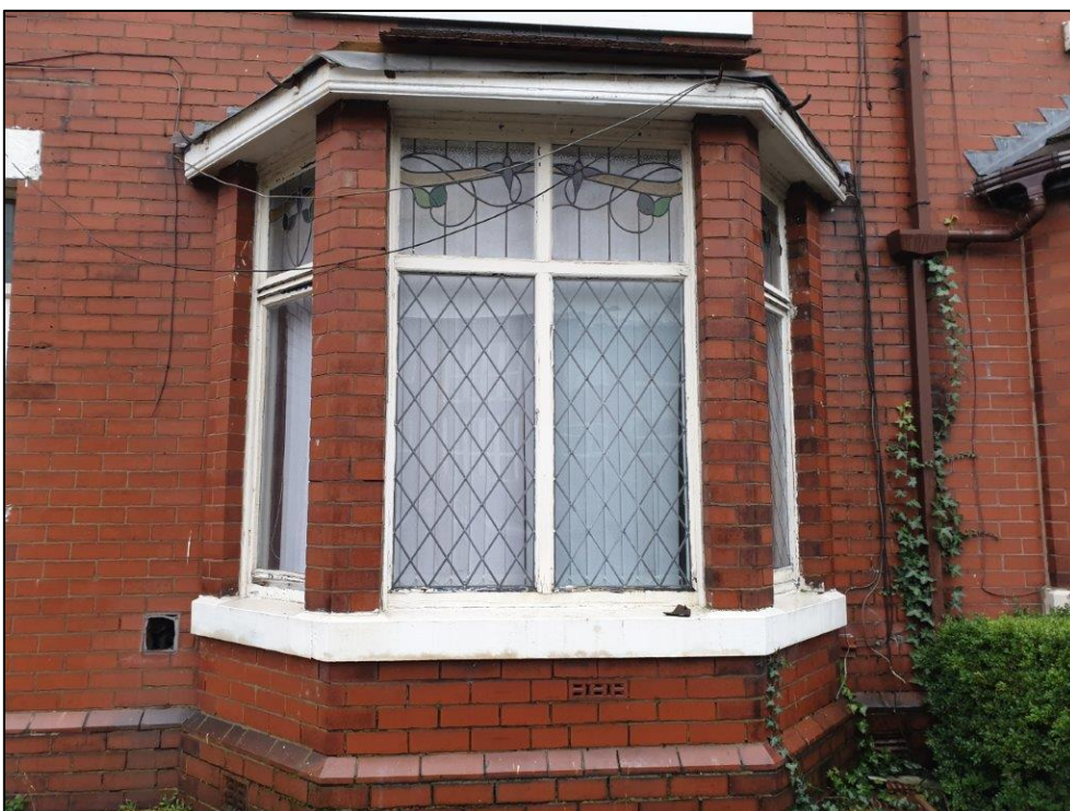
Image 2: Bay window at front elevation
