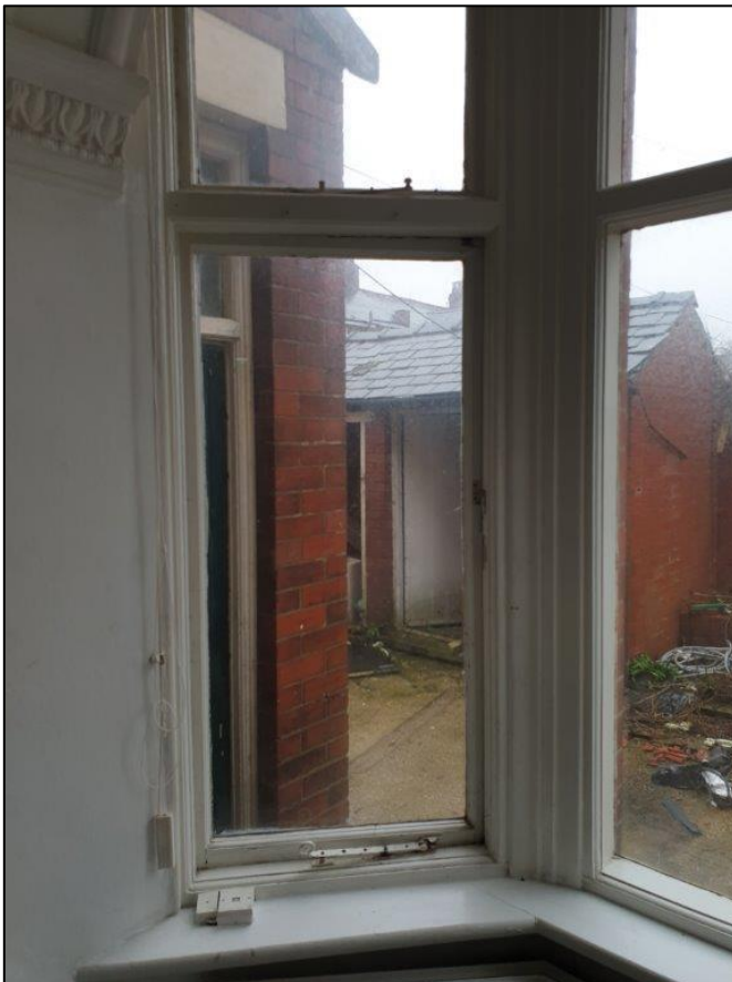
Image 20: Detailing of bay window frames at rear of the property
