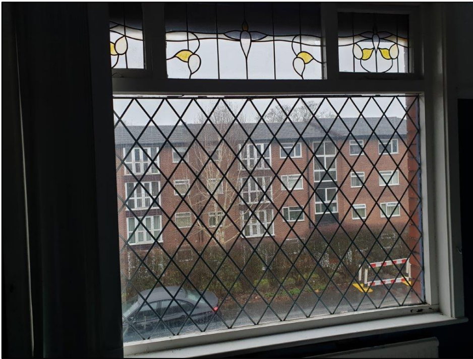
Image 25: Window on first floor at front elevation
