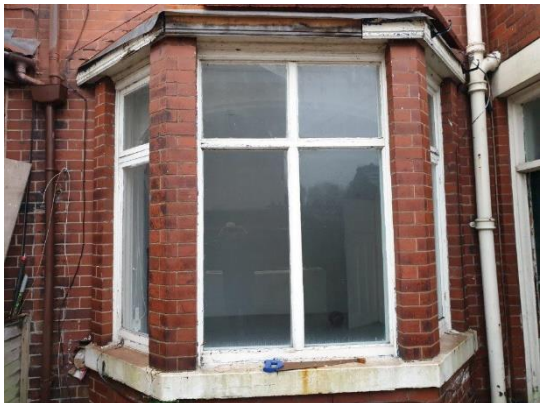
Figure 2.4: Bay window at rear elevation
