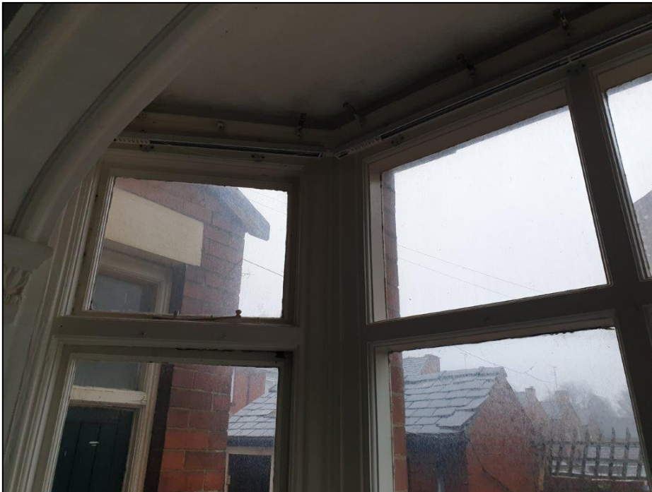
Image 19: Detailing of bay window frames at rear of the property
