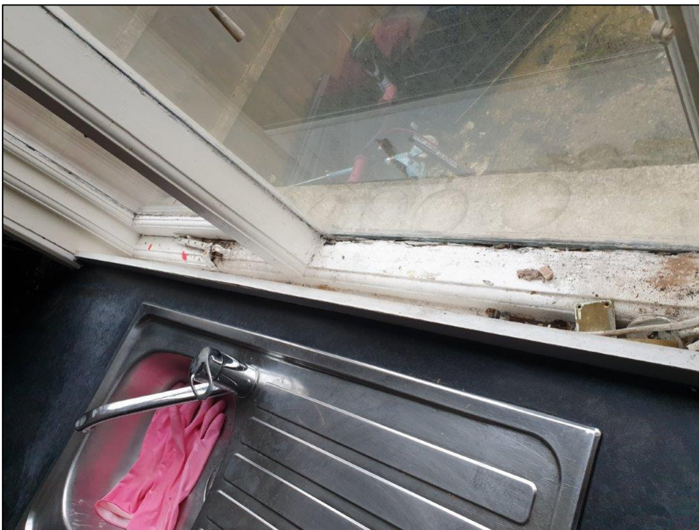
Image 22: Detailing of the window frame in kitchen window
