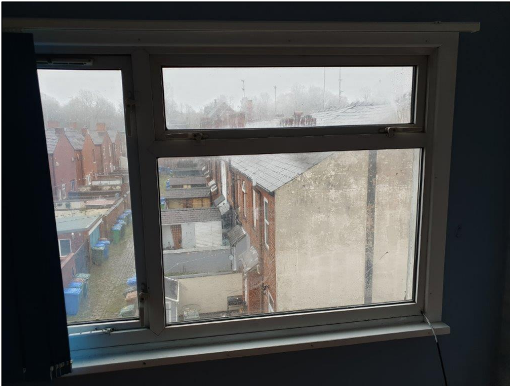
Image 31: Window from rear dormer extension
