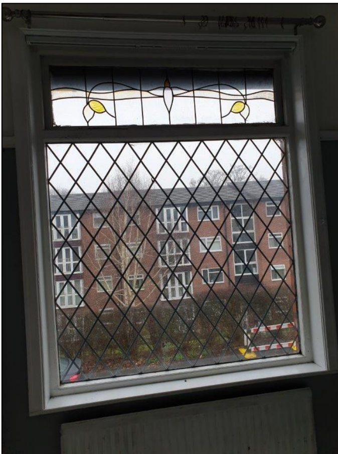
Image 26: Window on first floor at front elevation
