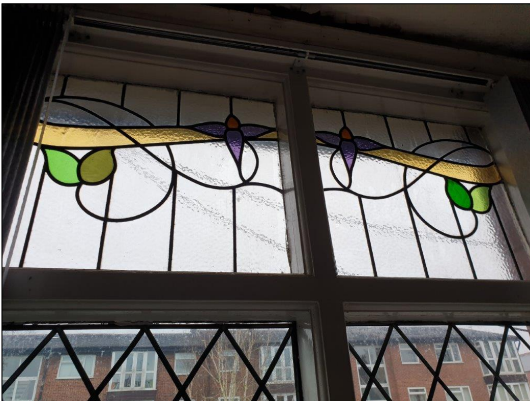
Image 16: Detailing of the front reception window glass pane
