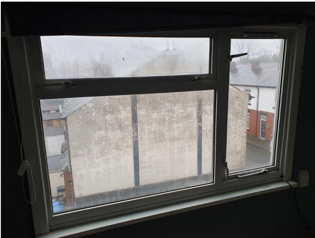
Image 32: Window from rear dormer extension
