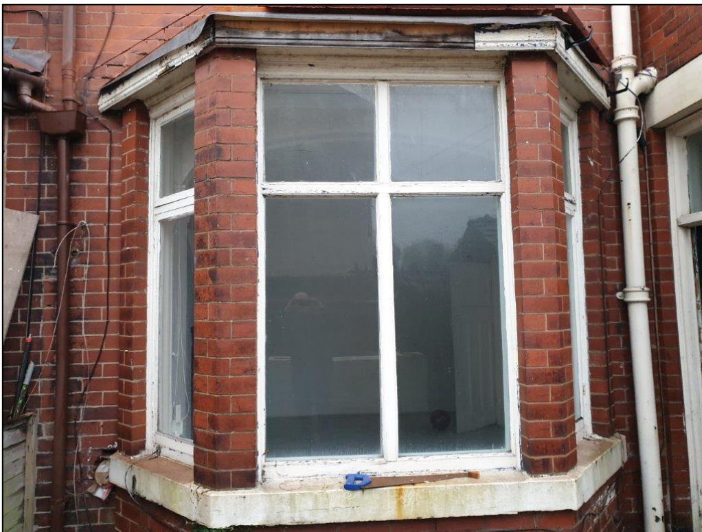
Image 4: Bay window at rear elevation
