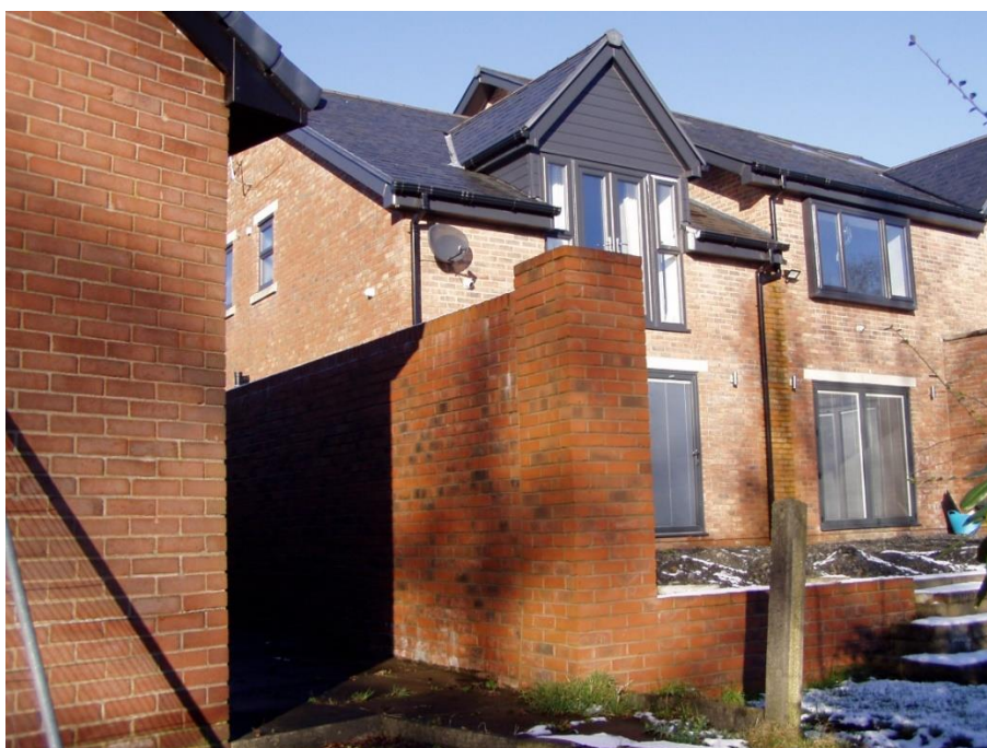
View of rear of number 45 – from rear garden on number 47 Bamford Way.
