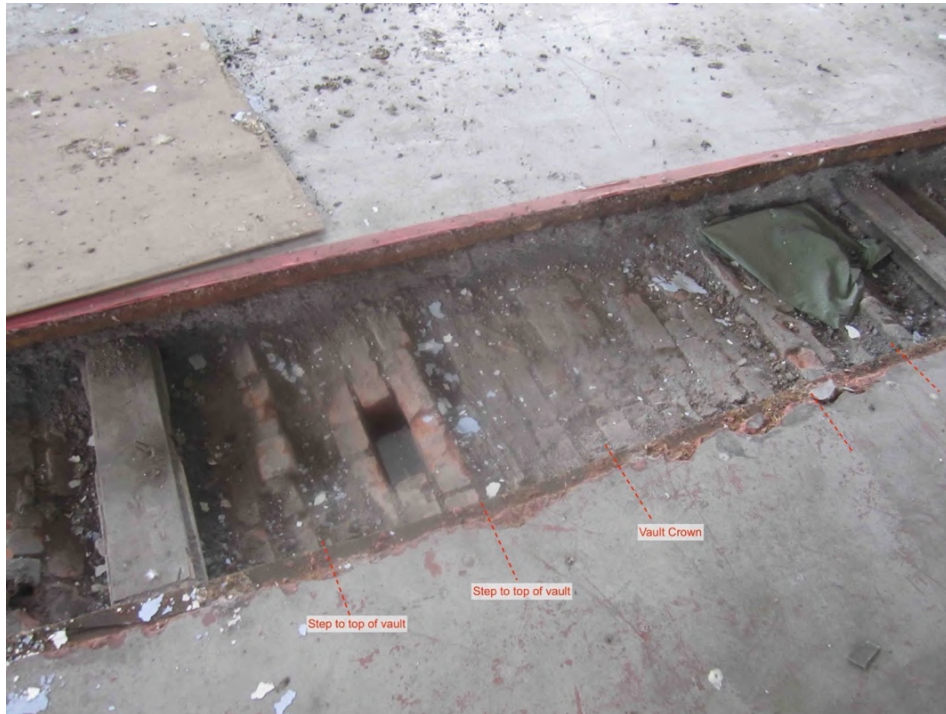
Photo 7 - Historic investigation (still open) to expose the top of the brick jack-arches (first floor)
