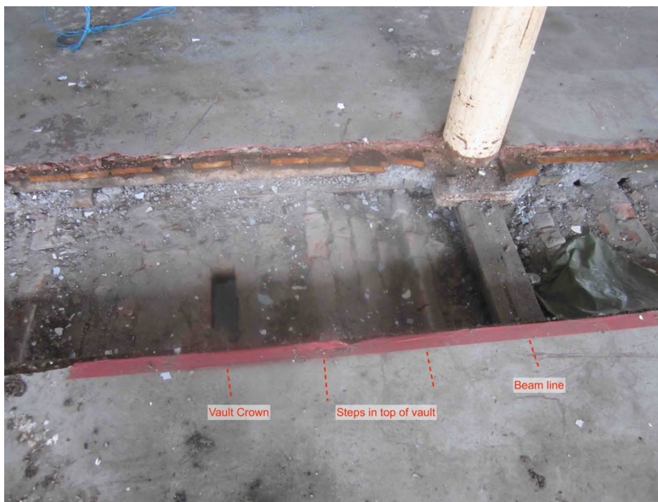
Photo 8 - Historic investigation (still open) to expose the top of the brick jack-arches (first floor)
