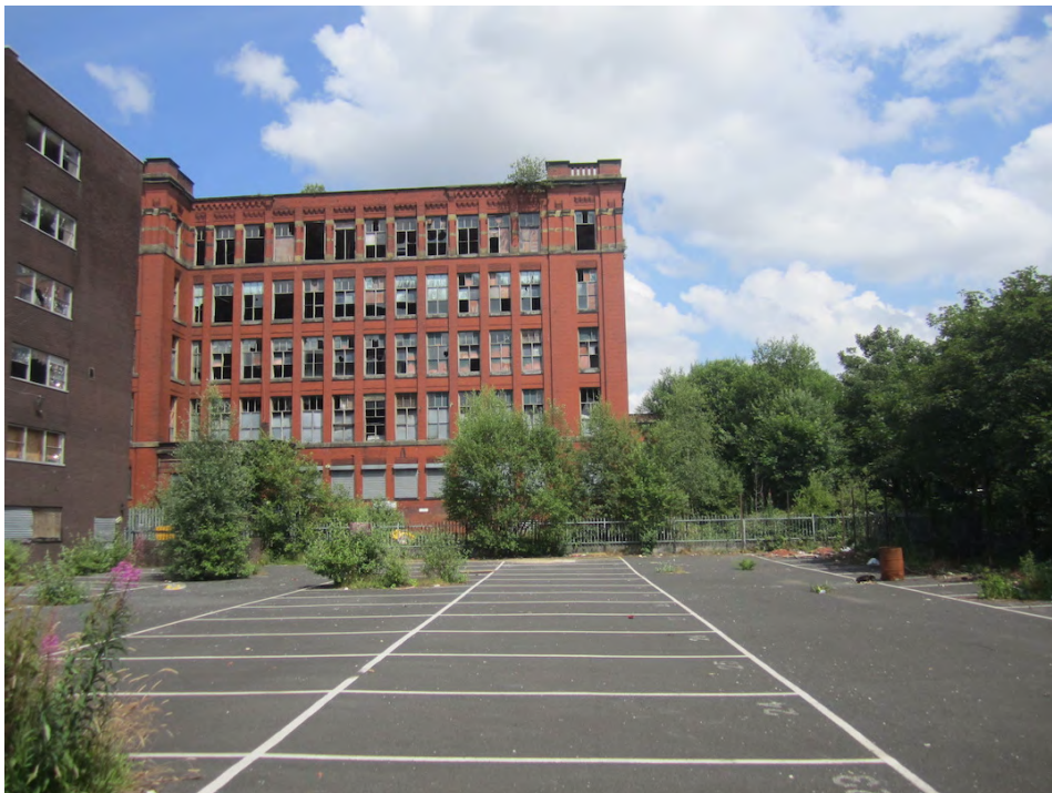
Photo 4 – Looking east across London House's car park
