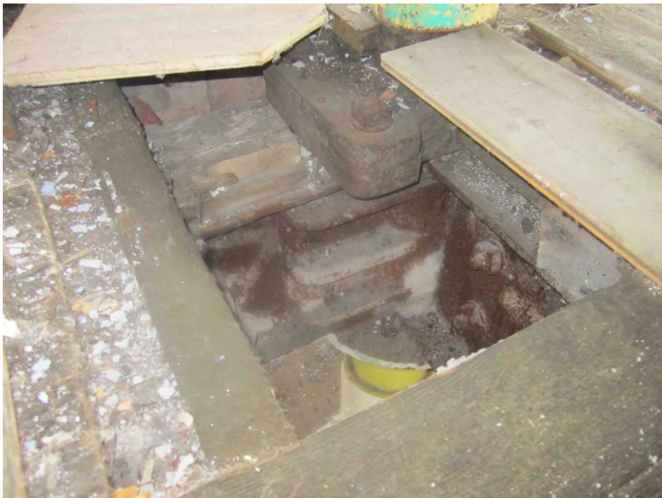
Photo 12 - Exposed column head detail at 3 rd floor level
