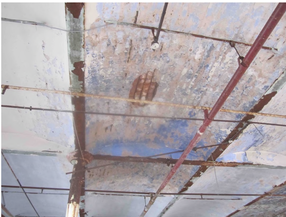
Photo 10 - Typical jack-arch soffit. Note tie bars (also sprinkler pipes)
