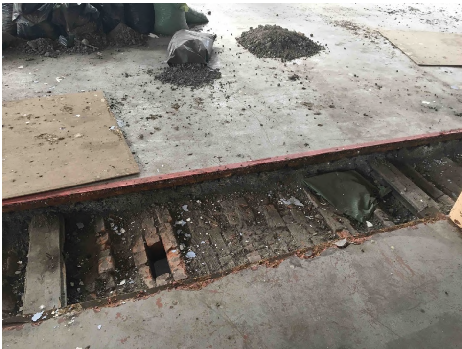
Photo 6 - Historic investigation (still open) to expose the top of the brick jack-arches (first floor)
