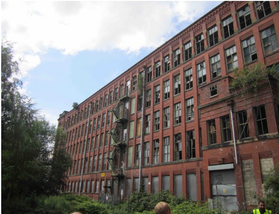
Photo 3 – View of the southern elevation
