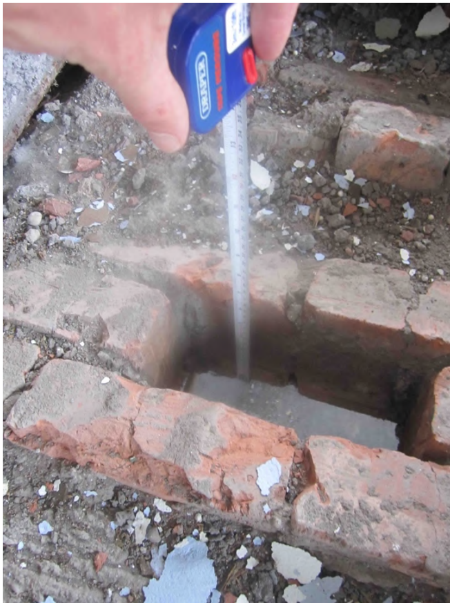
Photo 9 - Historic investigation (still open) exposing the half-brick crown of a brick jack-arch (first floor)
