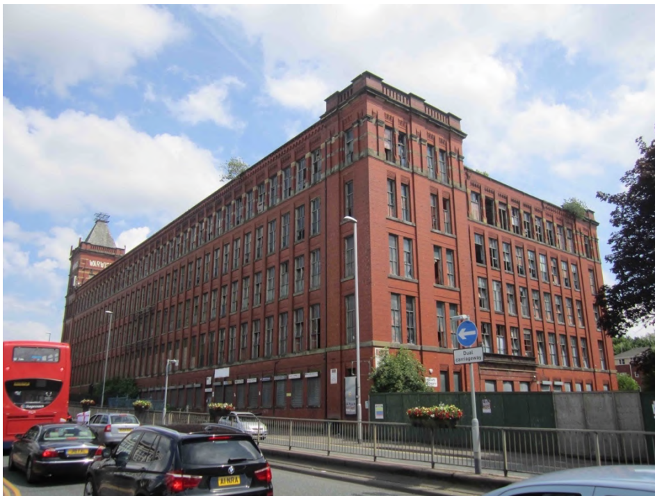
Photo 2 – View of the Mill from Oldham Road
