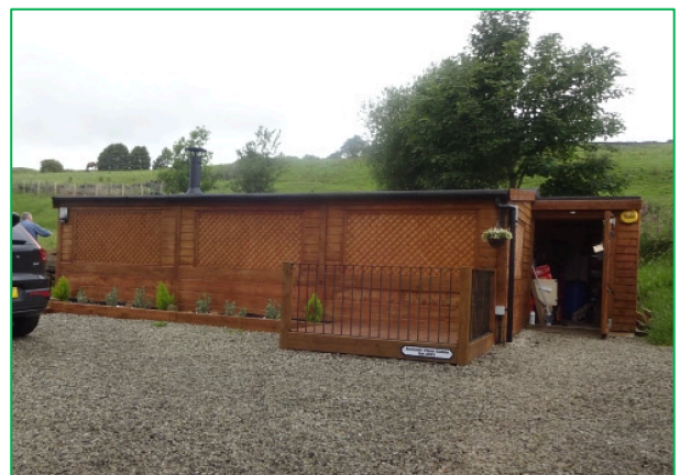
The cabin; developed land sealed surface
