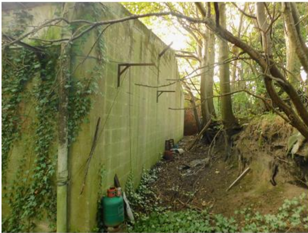
PHOTO 15 View along Eastern Elevation of Building 4
