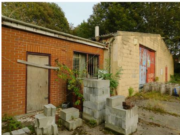
PHOTO 9 View Along Western Elevations
