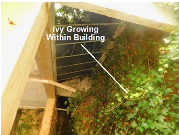
PHOTO 27 Underside of Eastern Part of Building 2 Roof
