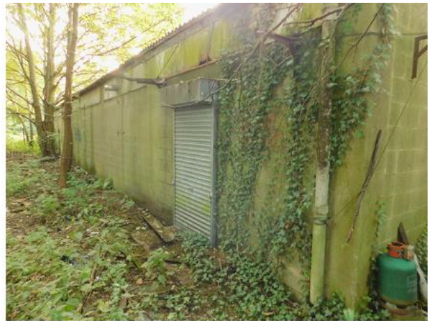
PHOTO 14 South-eastern Corner of Building 4
