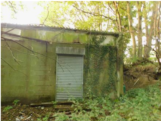
PHOTO 13 South-eastern Elevation of Building 4
