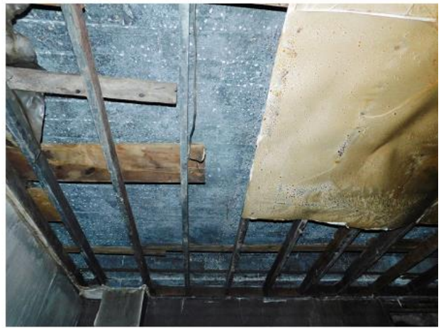
PHOTO 22 Underside of Building 1 Roof
