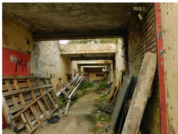
PHOTO 6 View Along Building 2 Passageway
