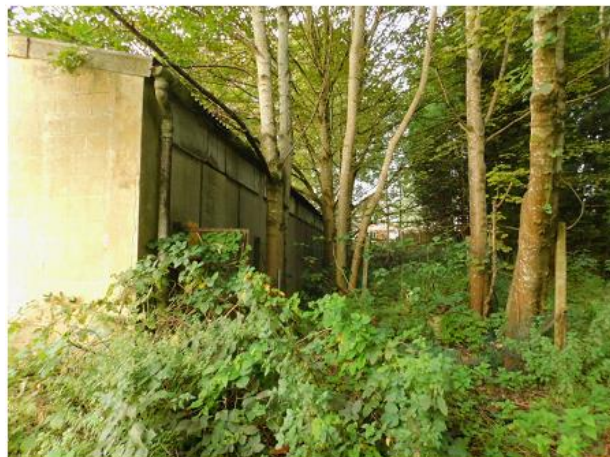
PHOTO 11 South-western Corner of Building 4
