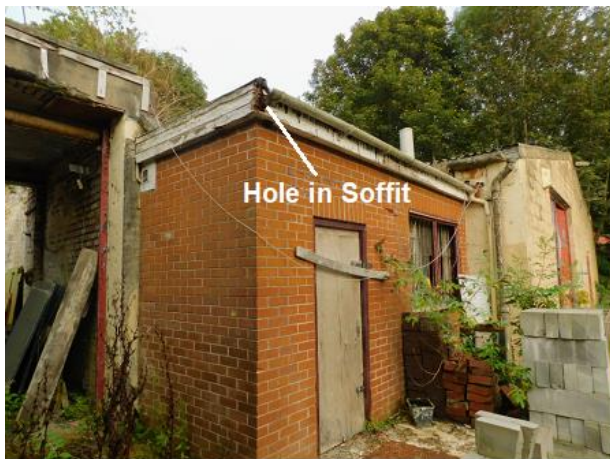
PHOTO 7 North-western Corner of Building 3
