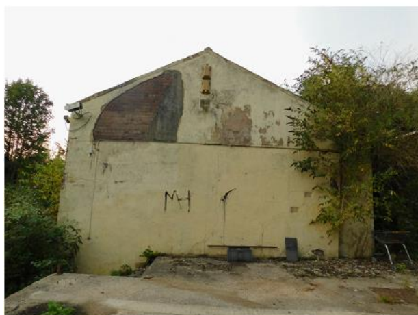
PHOTO 3 Southern Elevation of Building 1
