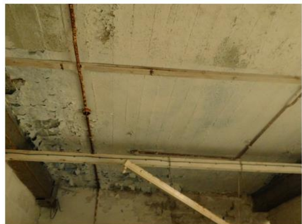
PHOTO 28 Underside of Building 3 Eastern Roof
