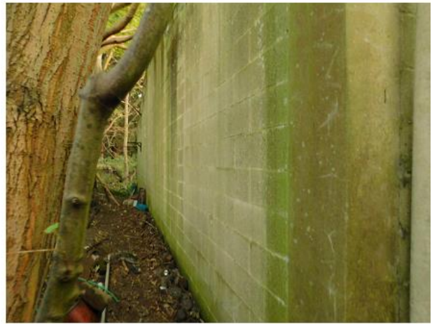
PHOTO 16 Eastern Elevation of Building 4
