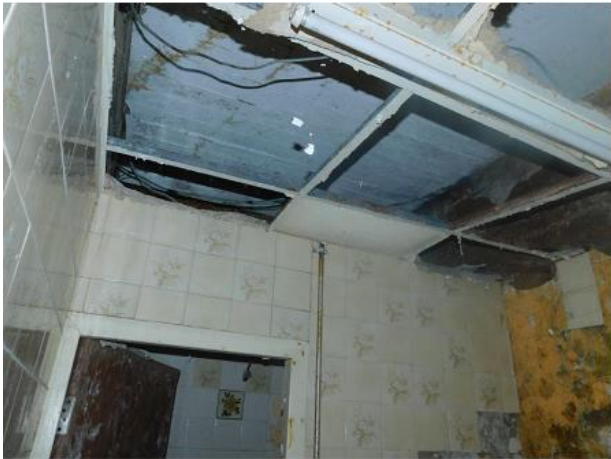
PHOTO 23 Underside of Building 2 South-western Roof
