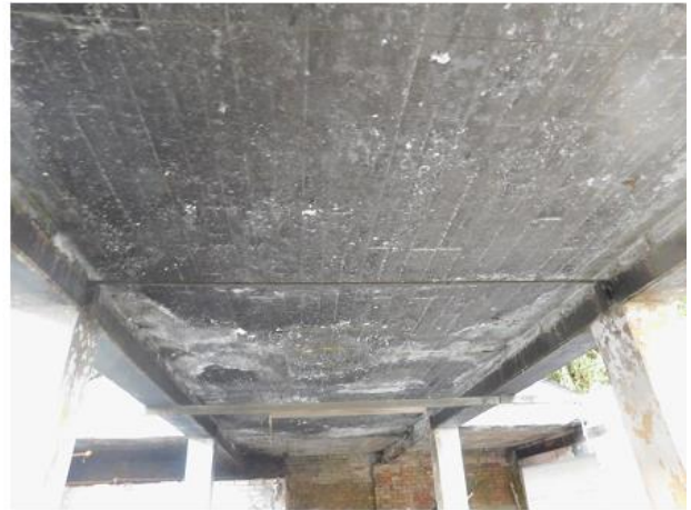
PHOTO 24 Underside of Building 2 Northern Roof
