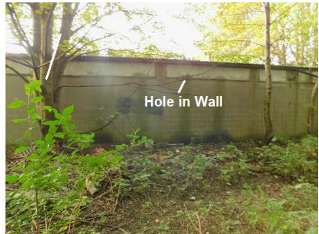
PHOTO 12 Southern Elevation of Building 4
