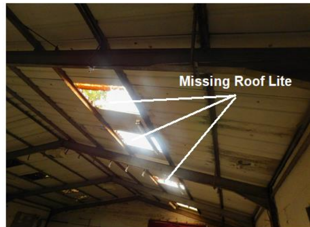
PHOTO 30 Underside of Western Roof of Building 4
