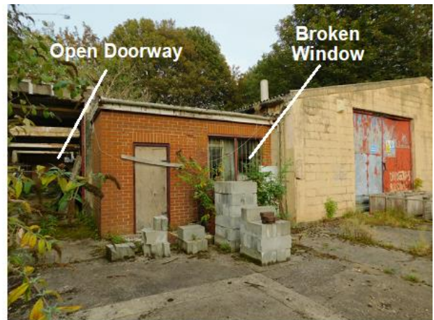
PHOTO 8 View along Western Elevation of Building 3
