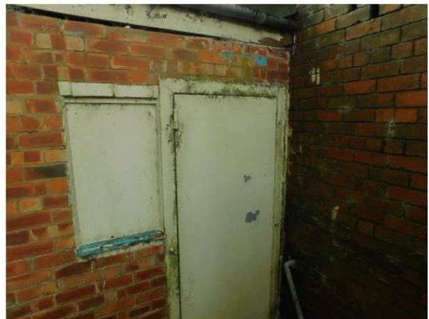
PHOTO 18 Junction of Buildings 2 and 3
