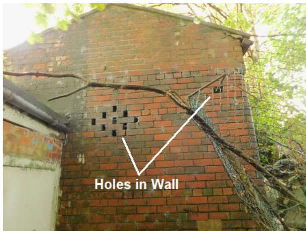
PHOTO 19 South-eastern Corner of Building 2
