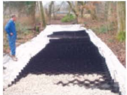
Installation of the CellWeb™ system.
