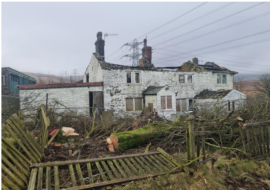
Derelict Longley Hey Farmhouse front view with dense vegetation in foreground.
