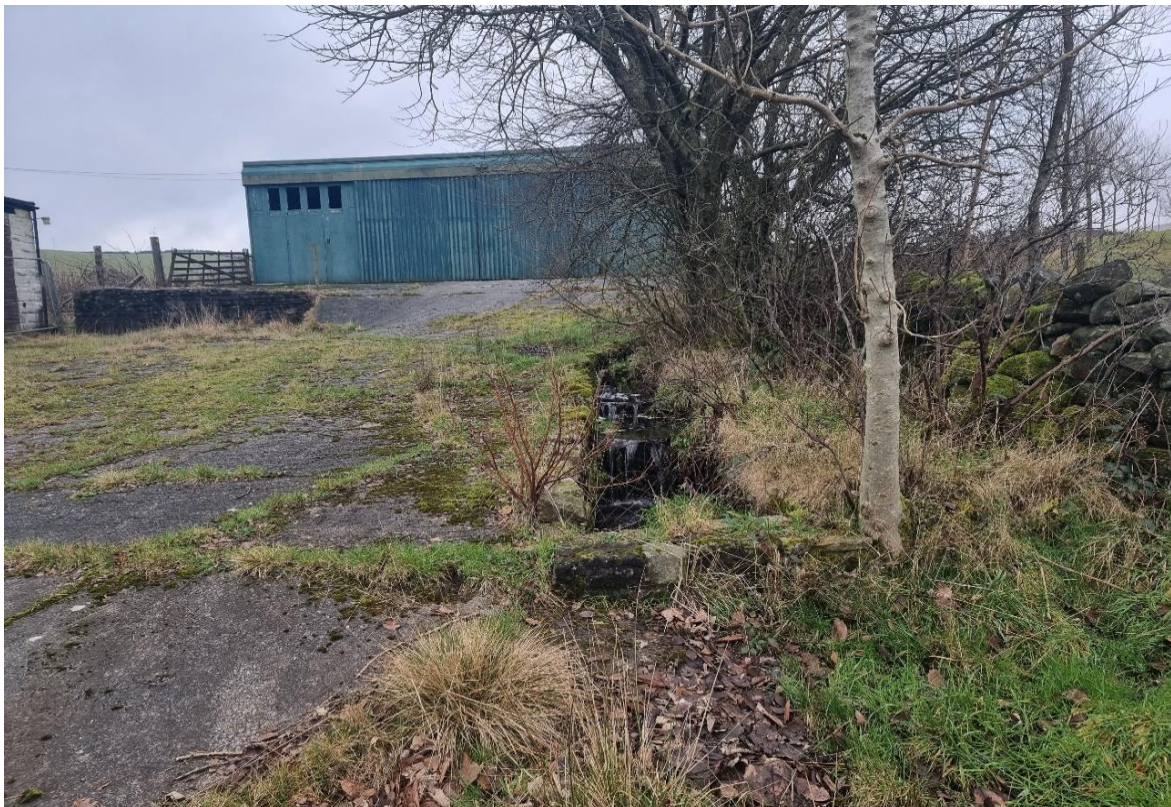
Open ditch and dry stone wall along the eastern site boundary.
