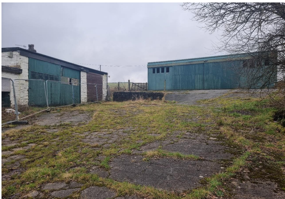
Out building on site in background with concrete hardstanding in foreground.
