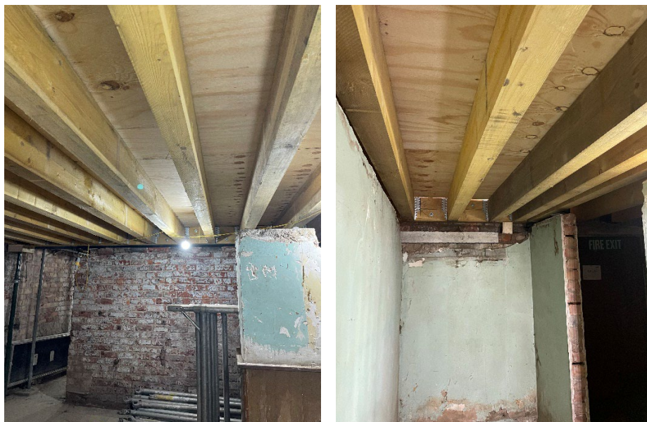
Figure.1 & Figure.2 showing softwood floor joists and softwood floorboards above.
