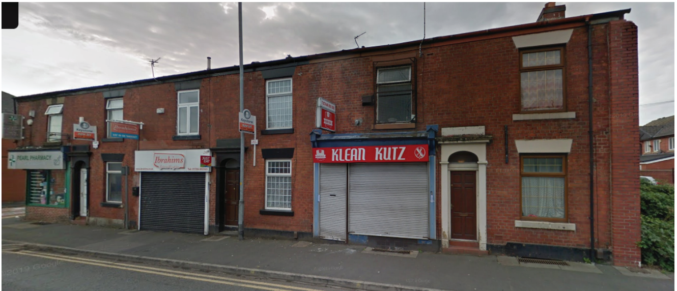
Above figure shows the front of the building on the end.
