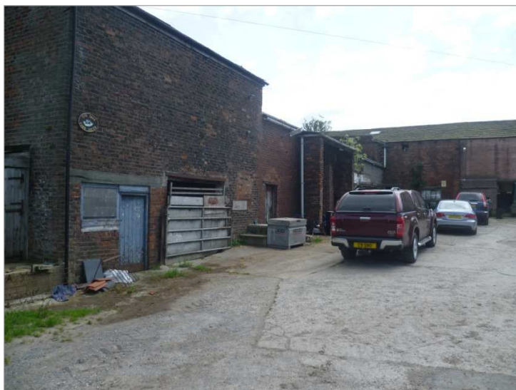
Western yard area roof water drainage discharges directly onto the yard and falls to access lane
