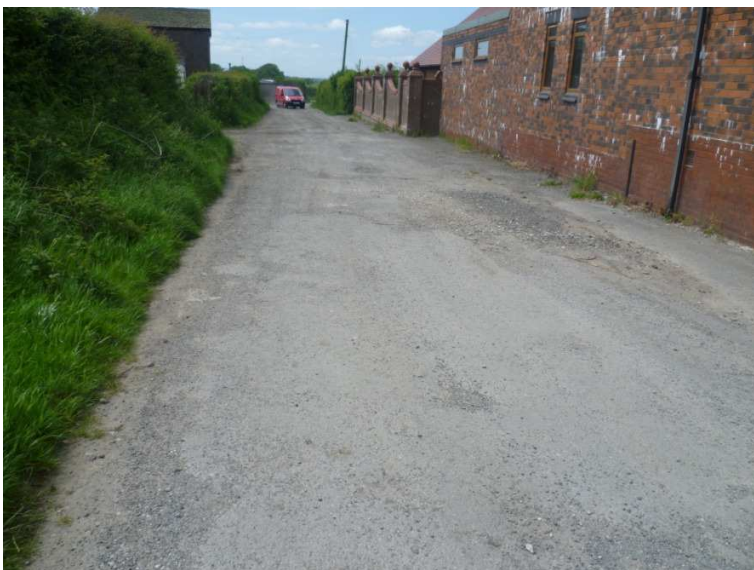
Access lane adjacent to the site
