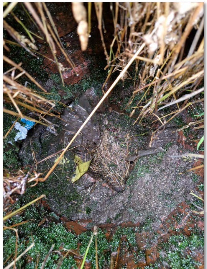
MH3 Internal View Before Clearing
