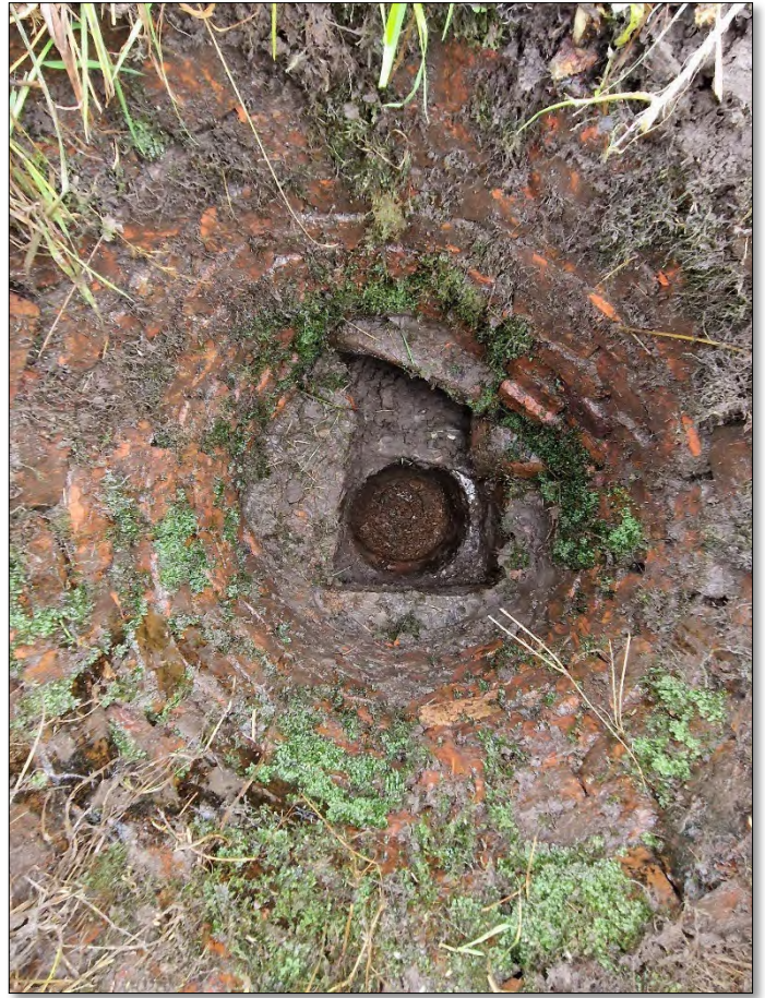
MH3 Internal View
