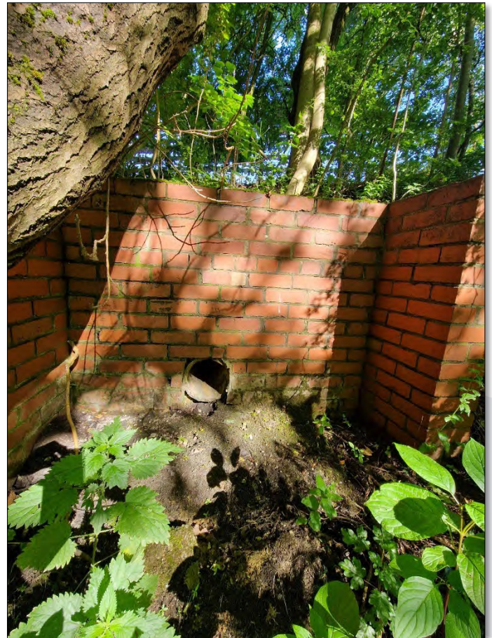
Pond Inlet Headwall
