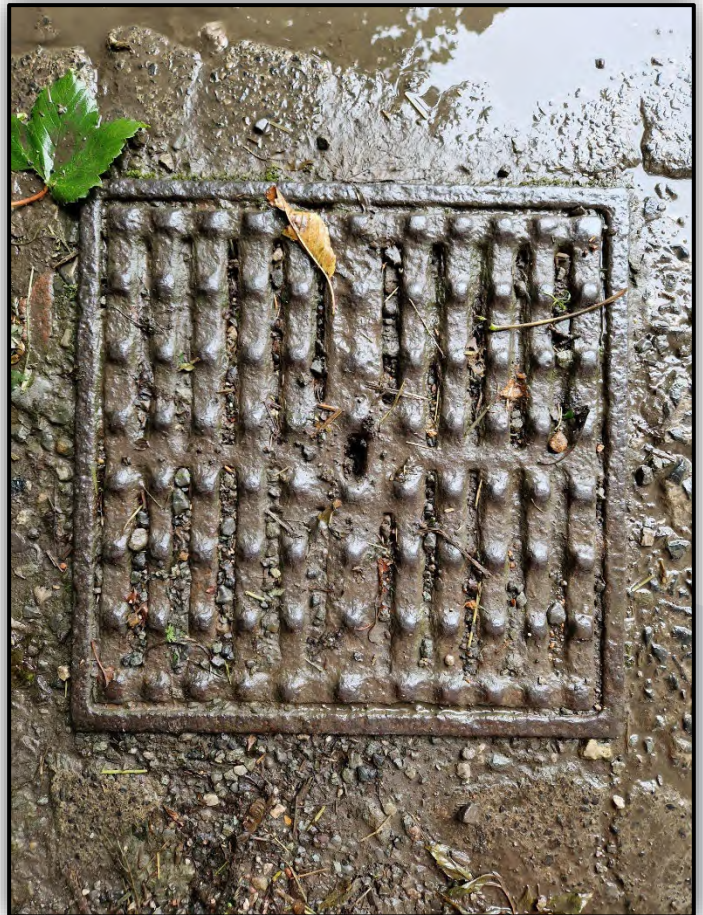
C5 Seized Grated Manhole Cover
