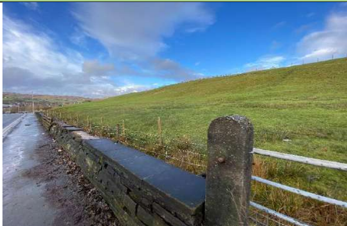
P5: Main Access gate looking north east along Hollingworth road
