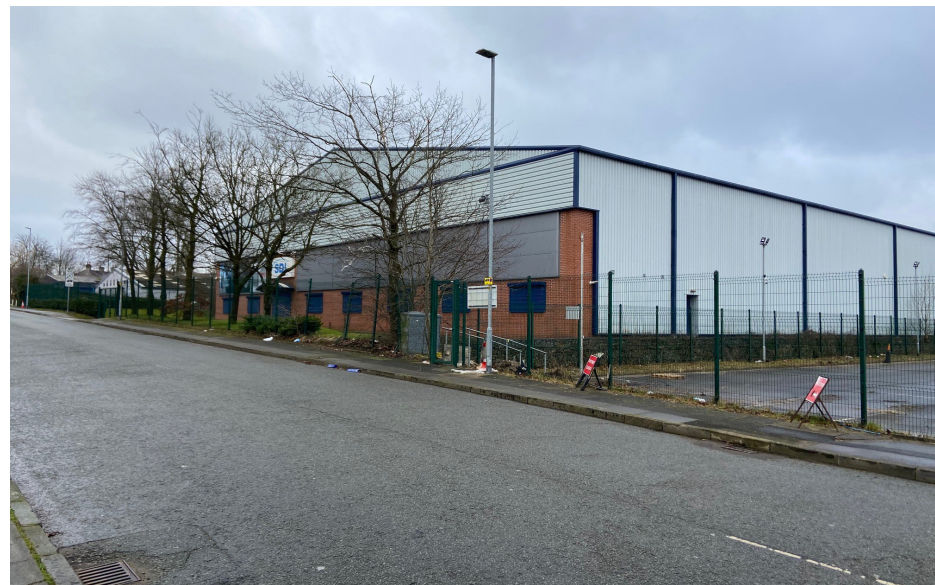
View looking east along Bentley Avenue taken from in front of site 15.02.24
