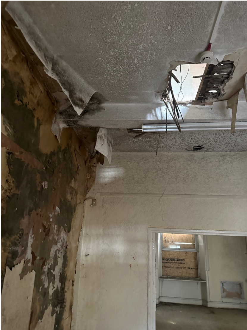
16. Office 2 wall & ceiling detail
