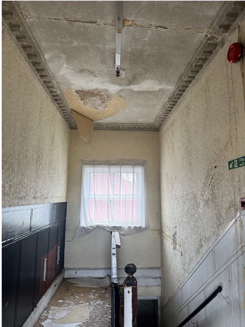
23. First floor landing
