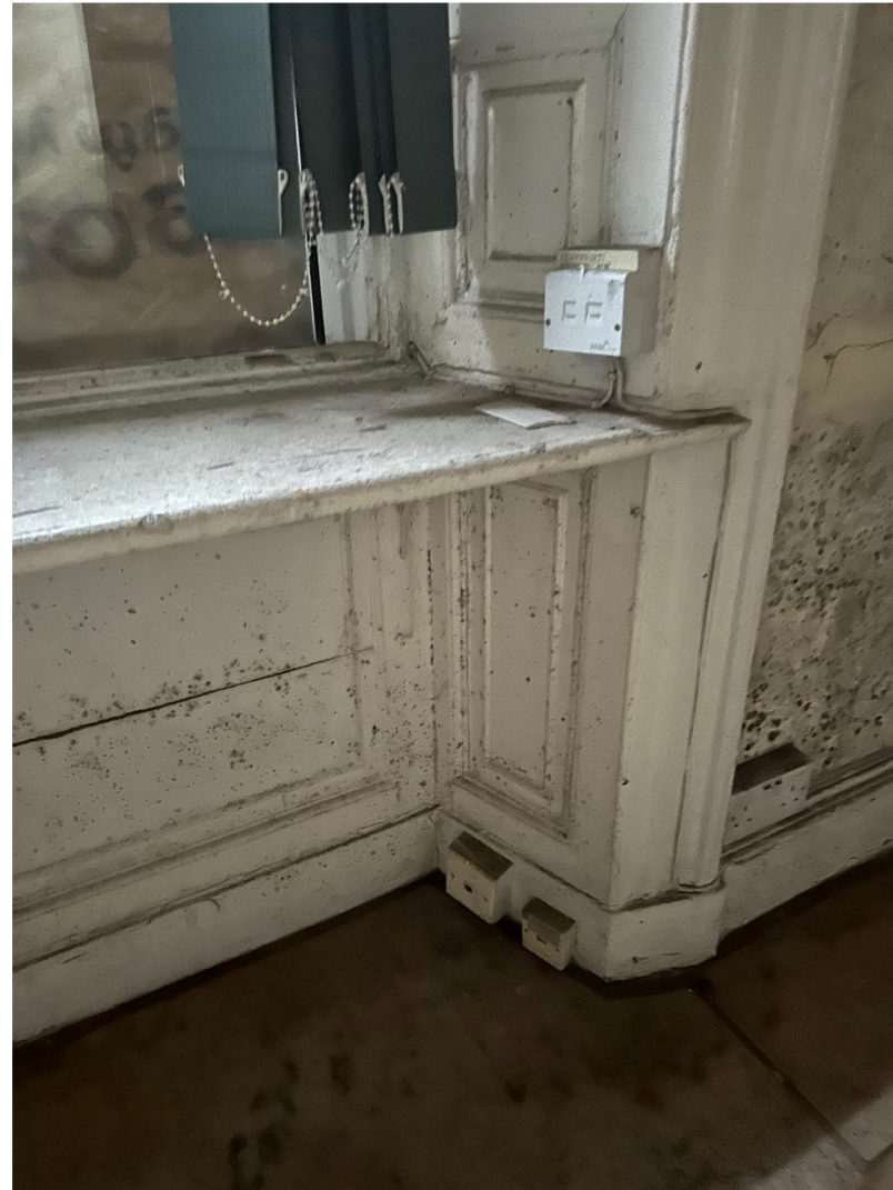
6. Admin front window lower panelling detail
