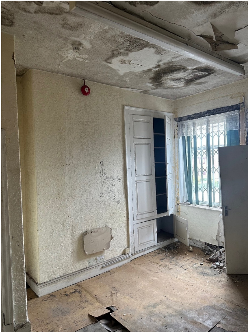
27. Office 6 general view
