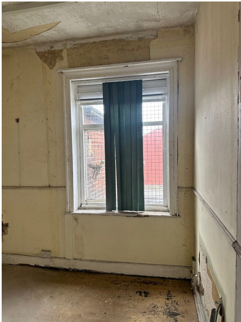
37.Office 9 window overlooking rear yard
