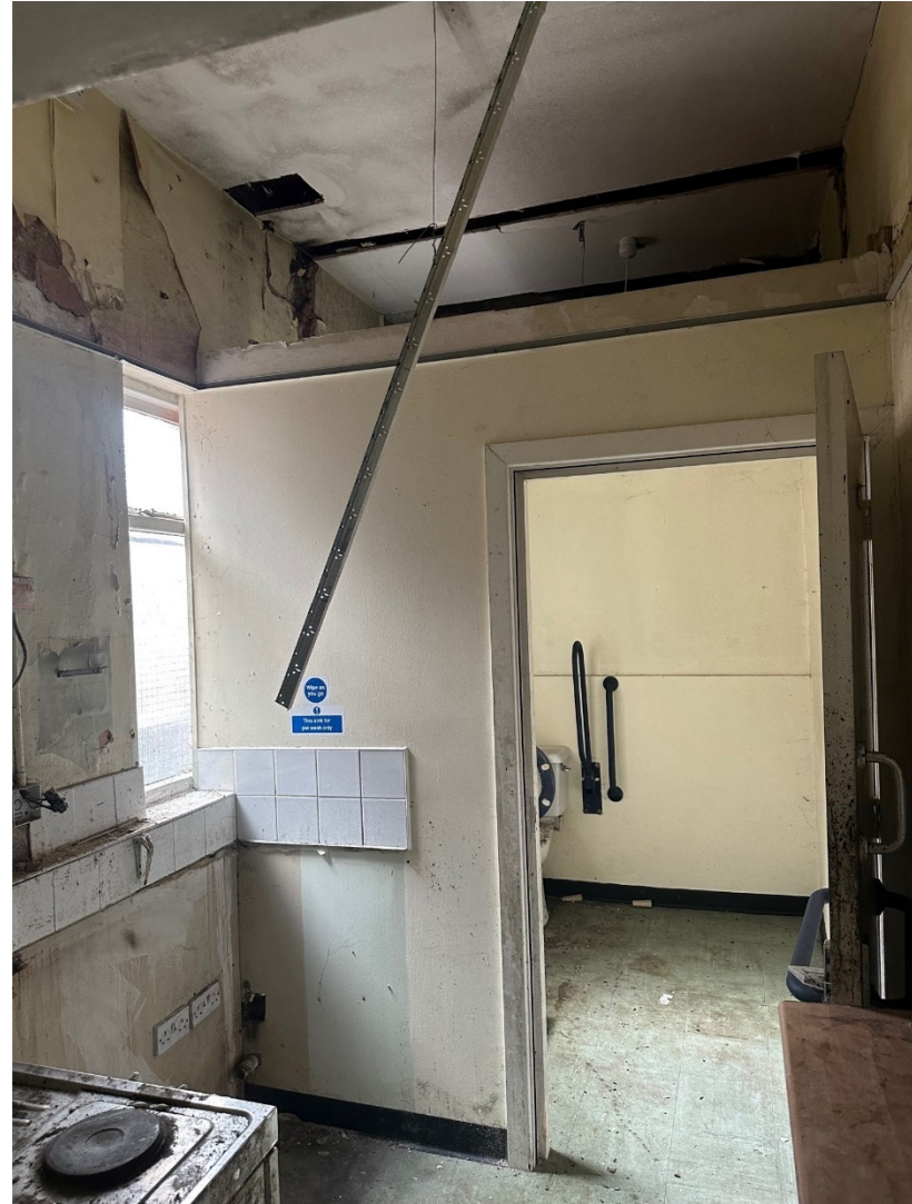
19. Kitchen & WC off office 2
