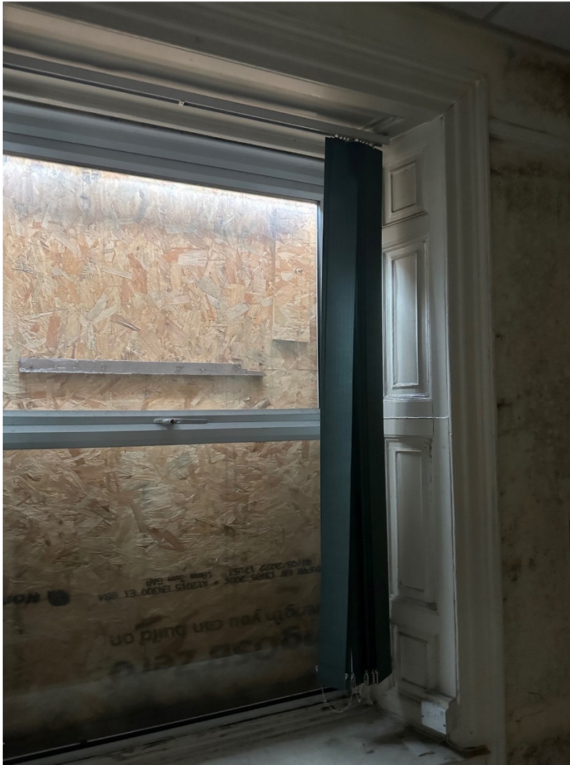
5. Admin front window panelling detail
