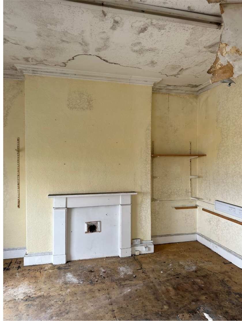
34. Office 8 chimney & ceiling detail
