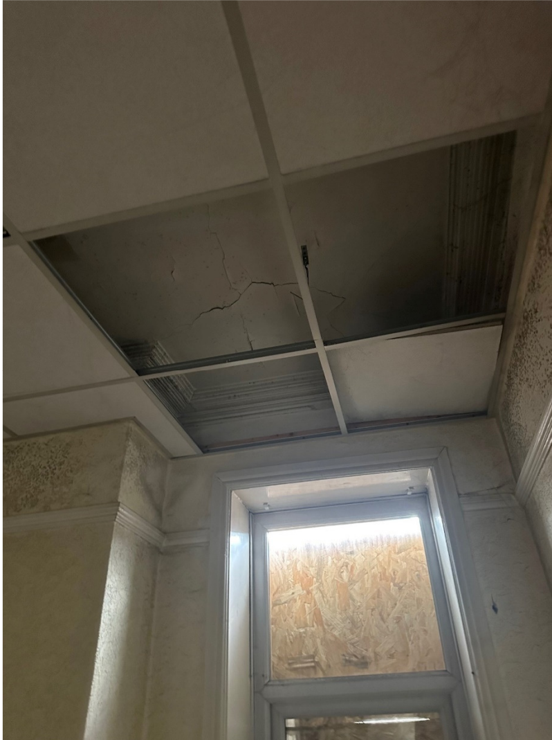
7. Admin side window & ceiling detail
