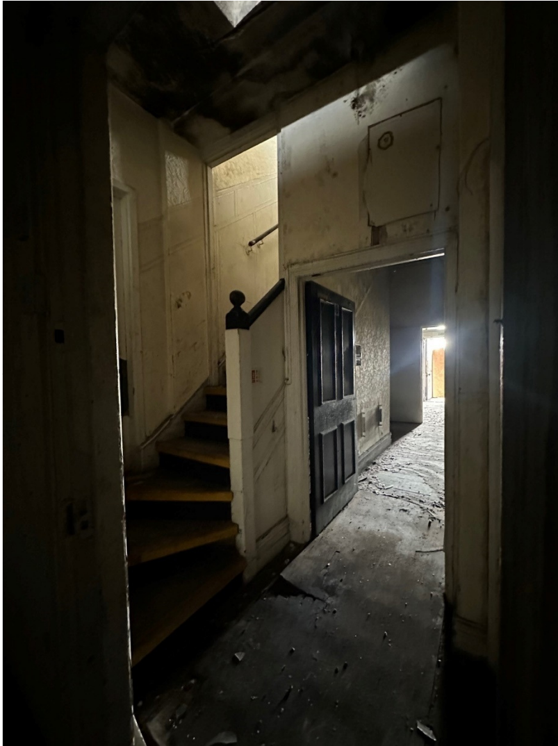
20. View of stairs leading to first floor
