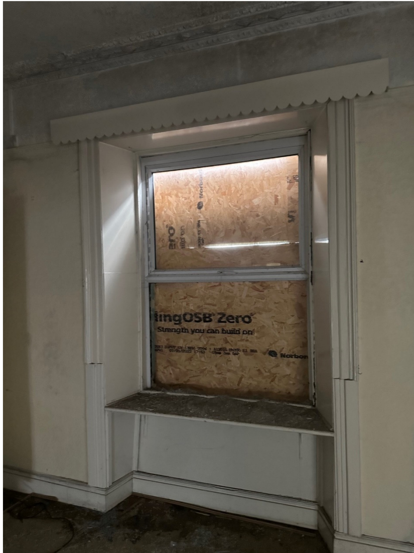
9. Office 1 front window panelling detail
