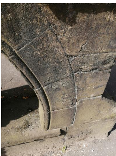
Stones numbered 31-33 - Voussoir stones profiled on 2 faces. No work required.
