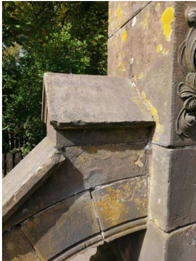
Stone number 8 – Coping stone with moulded profiles to 3 faces. No work required.
