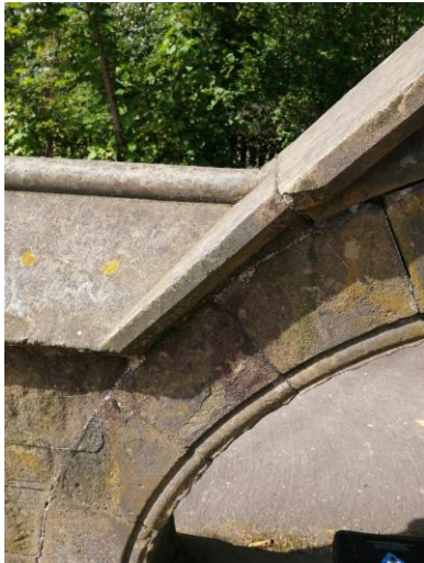
Stones numbers 13, 14 & 16- Voussoir stones profiled on 2 faces. No work required.
