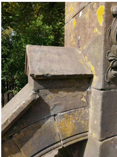
Stones numbered 10 & 12 – Voussoir stones profiled on 2 faces. No work required.
