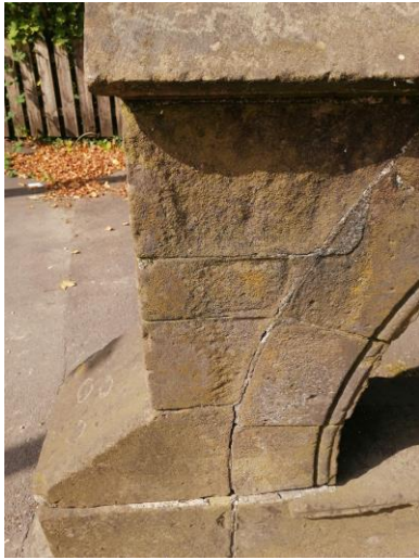
Stone numbers 19&20- Ashlar return stones. No work required.
