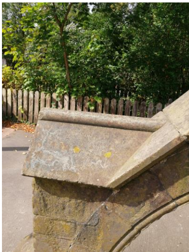
Stone number 15 – Kneeler stone profiled on 3 faces. No work required
