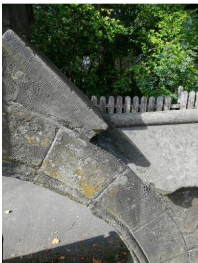
Stones numbered 27-30 - Voussoir stones profiled on 2 faces. No work required.
