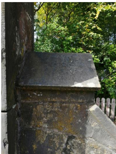
Stone number 26 — Coping stone with moulded profiles to 3 faces. No work required.
