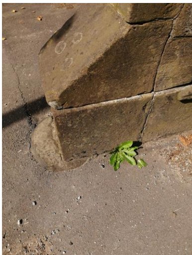
Stone number 22- Ashlar return. No work required.
