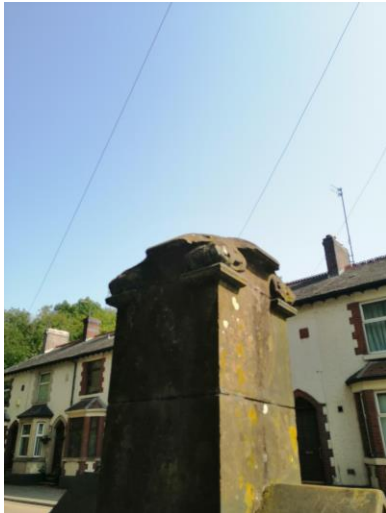
Stone number 1- Missing mouldings no work required.
