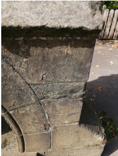
Stones numbered 34-35- Ashlar return stones. No work required.
