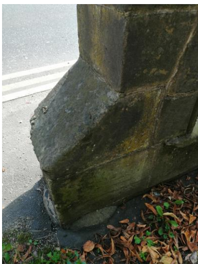
Stone number 37- - Ashlar return. No work required.
