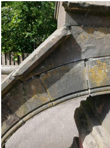
Stone number 9 & 11 – Coping with moulded detail on 2 faces incorporating radius ashlar. No work required.
