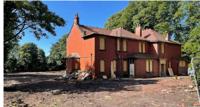
Figure 3.2: Front Elevation to the Red House (August 2022)
