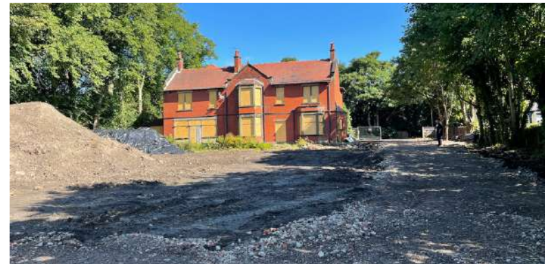
Figure 3.3: Garden Elevation to the Red House (August 2022)
