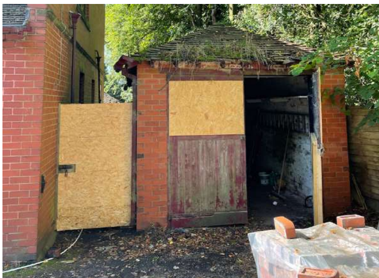
Figure 4.11: Existing Garage (August 2022)
