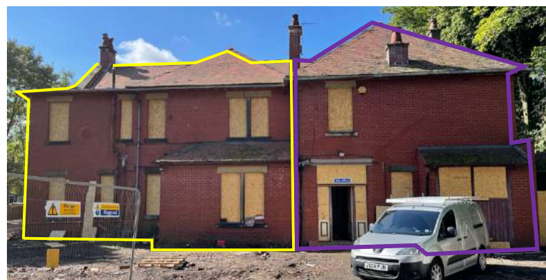
Figure 4.10: Front Elevation to the Red House (August 2022)
