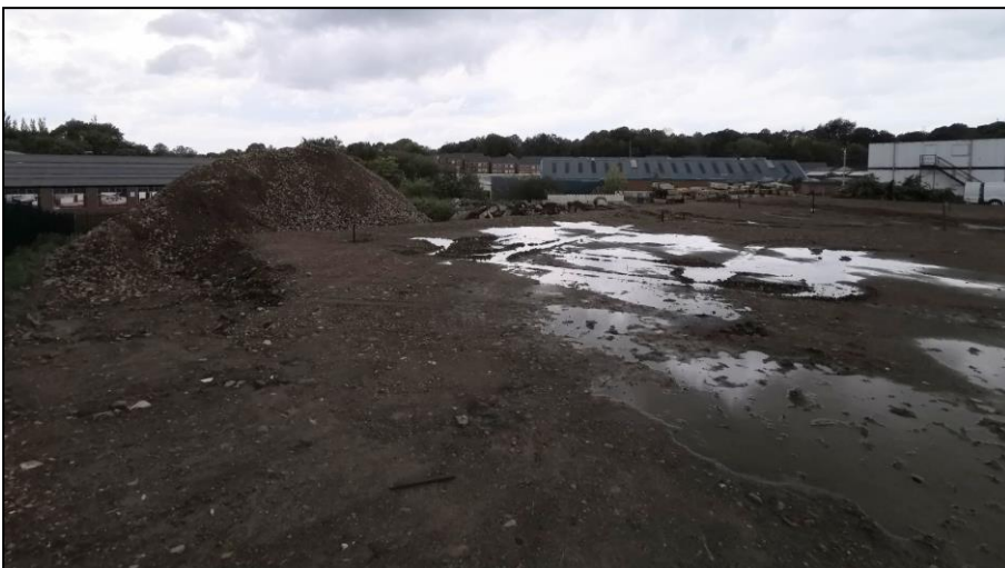
South side of the site looking west.
