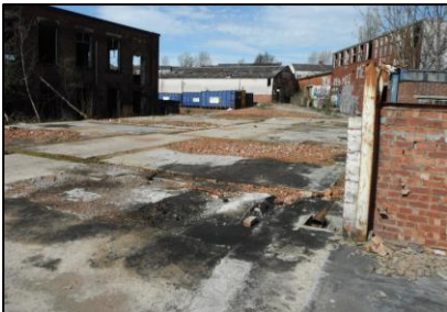
Potential spillages - putrid & minor H/C odours (Building 11).
