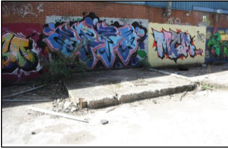
Concrete plinth to former tank adjacent E side of Building 1.
