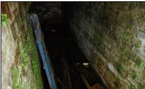
Service trench (Building 3 to N of Site).
