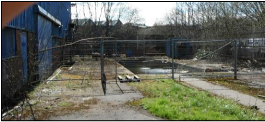
Bunded area SW of Building 1.
