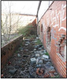
Former location of tanks to N of Building 4.
