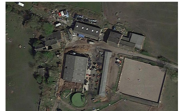
Farm off Jowkin Lane - metal sheeting to pitched roofs
