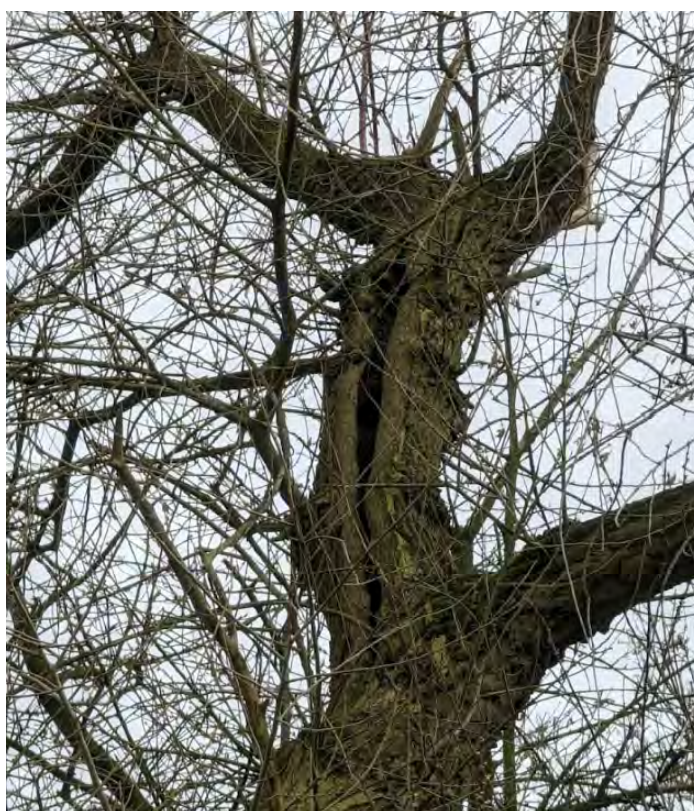
Photographic plate showing some damage in the crown of T8 likely caused by a branch failure.
