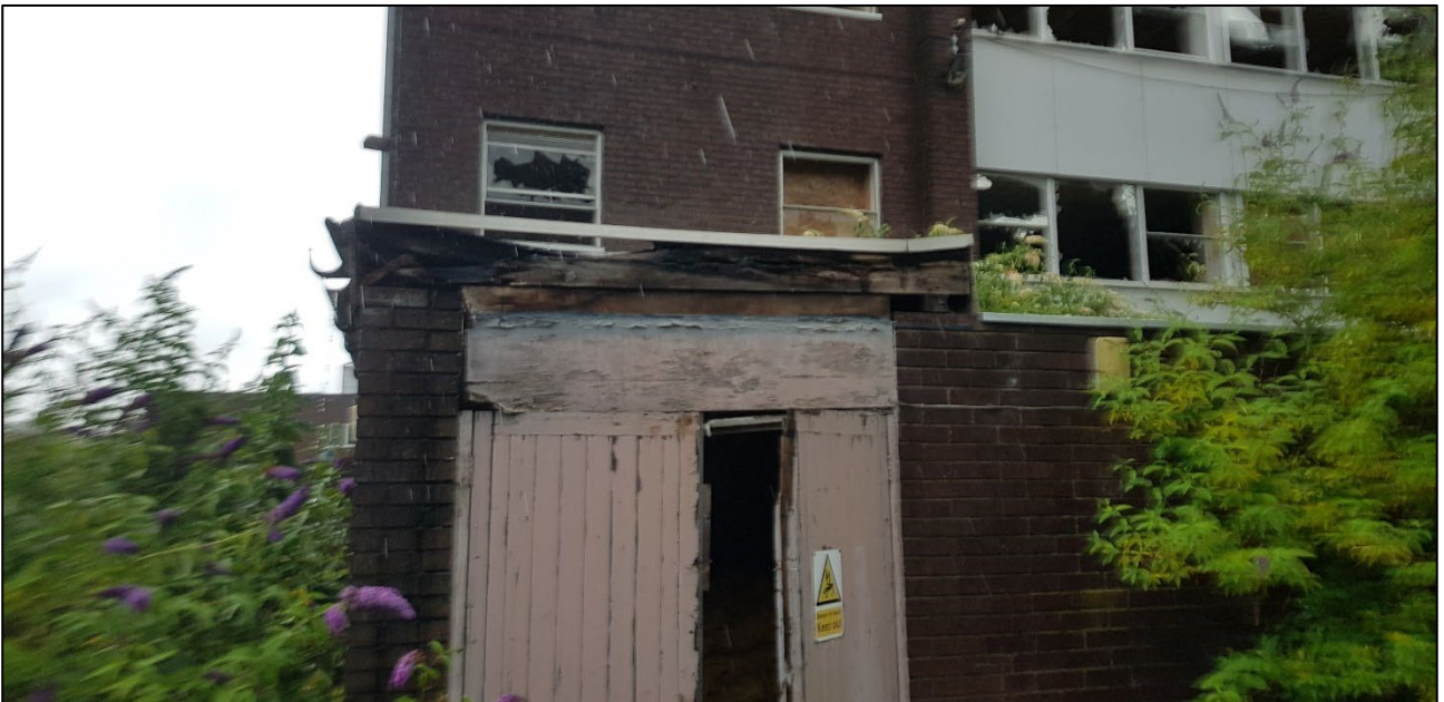
Photo 04. Small Shed/electricity generator building (u1b5)
