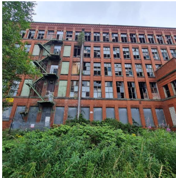
Photograph 5: Rear view of Warwick Mill
