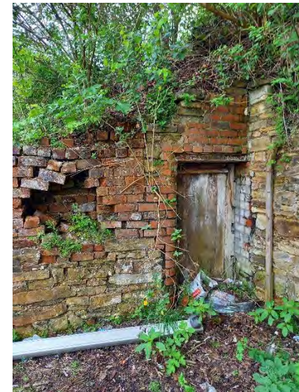
Retaining wall at south of site.
