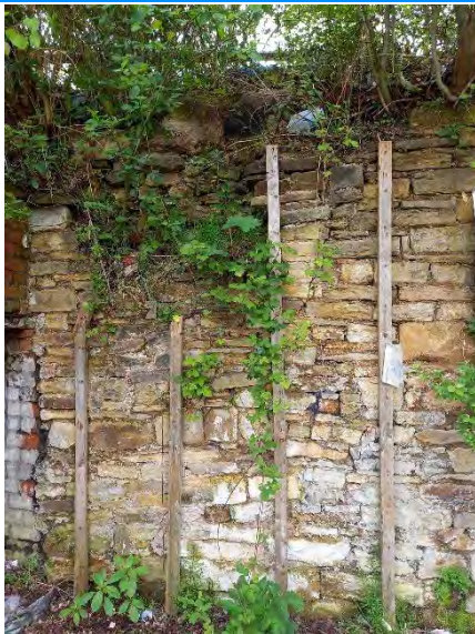
Retaining wall at south of site.
