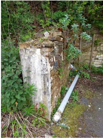
Retaining wall at south of site.
