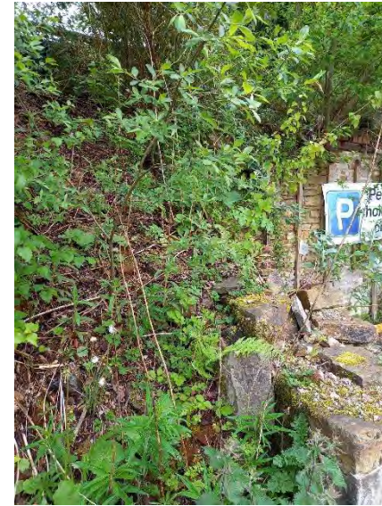
Retaining wall at south of site.
