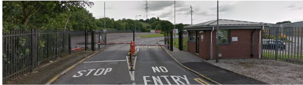
1 Existing Gatehouse to Rhodes Business Park
