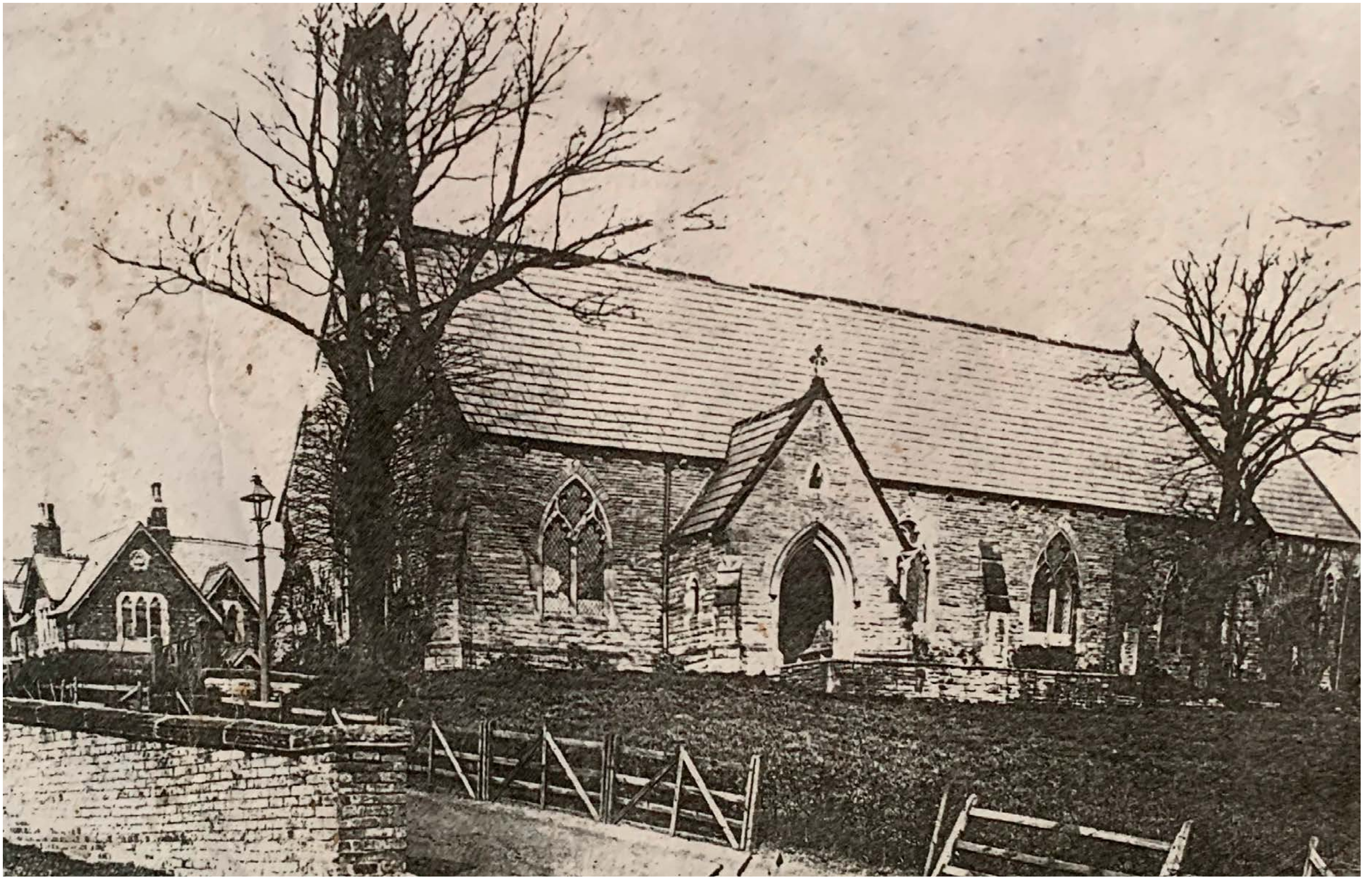
Figure 12 Historic Photograph of Holy Trinity, August 1899
