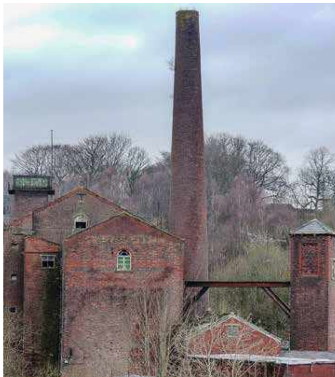
Pilsworth Clough Mills bleach works
