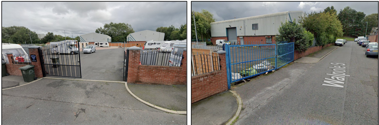
Figure 2.3 – Existing Site Accesses. Left image – Northern Walpole Street Access. Right image – Southern Walpole Street Access
